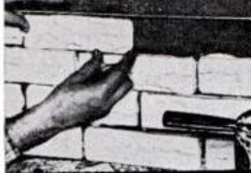
ADHERE BRICKS TO WALL
