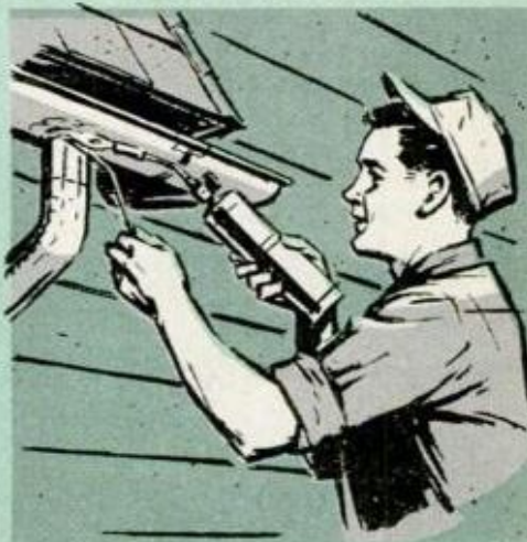
3. GUTTER LEAKS are easily stopped by flowing solder over pinpoint openings at joints. Surface must be thoroughly cleaned
