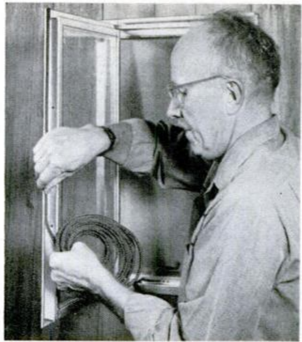
METAL CASEMENT SASH require special U-shaped strips, a number of types of which are available in both metal and vinyl, as in Fig. 5 and photo below
