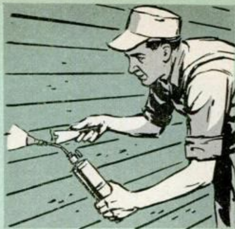
1. OLD PAINT is softened almost instantly by furnace-hot flame from a propane torch. Follow up with scraper
