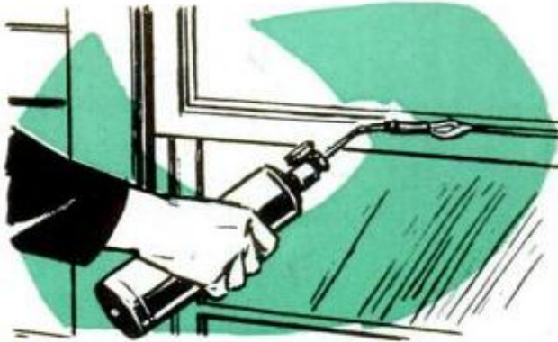
16. OLD PUTTY can be softened in a single, slow pass of torch flame. Move flame just fast enough to prevent charring wood. Remove putty while still soft
