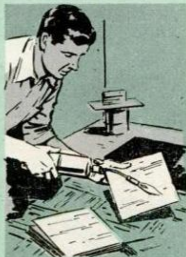
4. REPLACEMENT floor tiles drop easily into place and take floor contours when heated with torch
