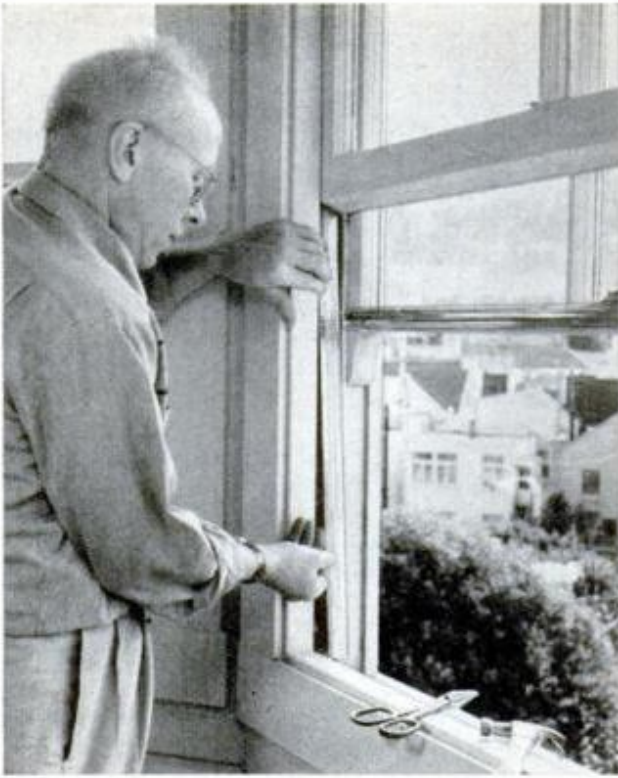
SPRING-METAL WEATHERSTRIPPING , see Fig. 2, is easily cut with small tin snips and can be installed on windows as above, or on doors. When installed on a door a special strike-plate strip is used as in Fig. 7
