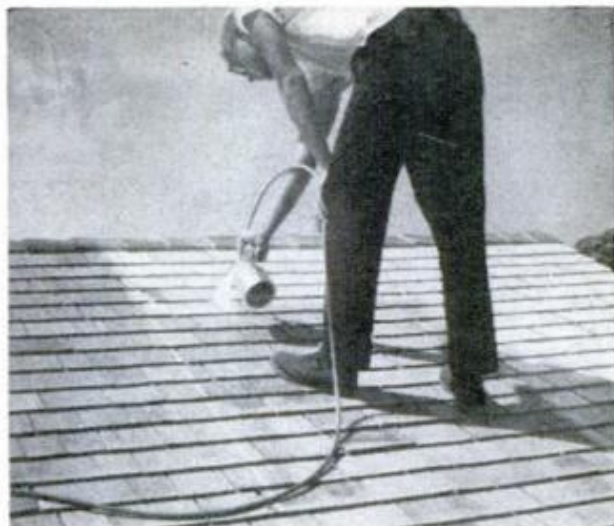
SECTION ROOF with chalk lines. Then stop spray pattern at lines and you won't end up with laps that show when paint dries. Adjust nozzle to round spray
