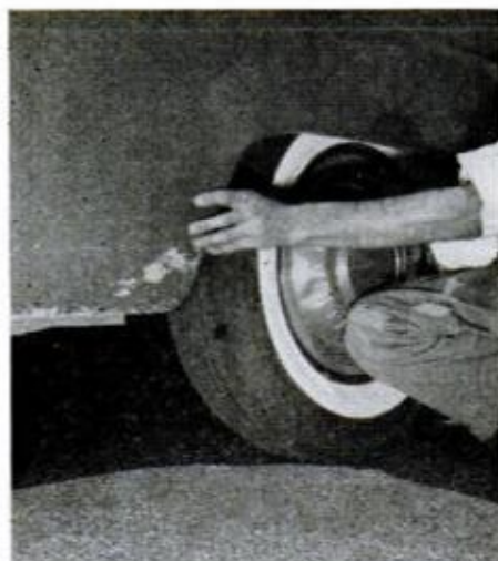
8 RUST ON ROCKER PANEL may not be serious; on doors and main panels, it spells repairs
