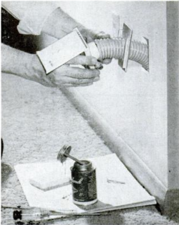
7. FLEXIBLE DUCTING is forced over stud on back of inlet valve to make airtight connection in line
