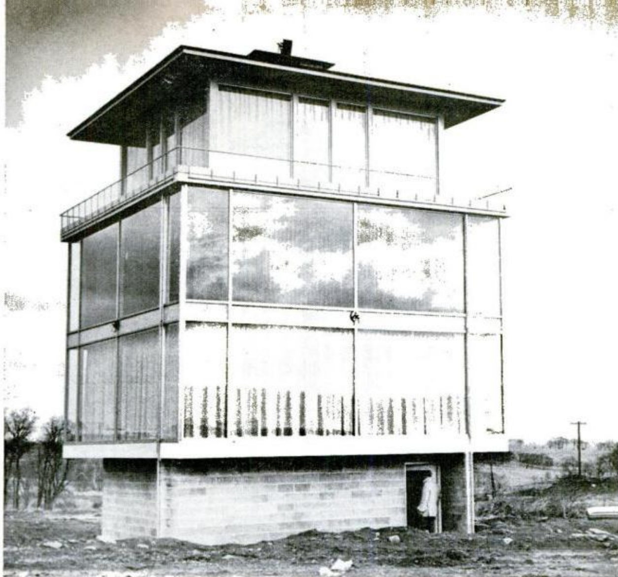
HAJJAR HOUSE has two "air wall" stories; top floor has a conventional glass wall for study control
