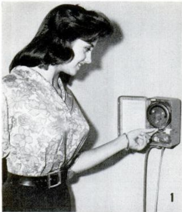
TIMER IS SET by inserting pins in slots. External manual switch may be used to shut off the system
