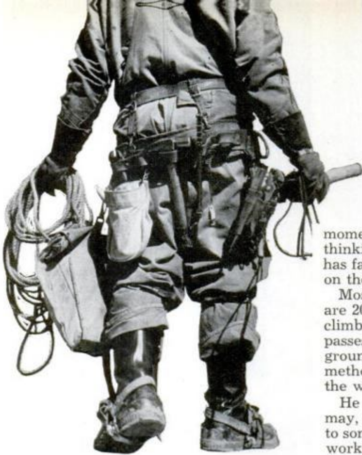
WELL-DRESSED LINEMAN will look something like an overdone science-fiction character. When fully equipped, he will carry up to 30 pounds of equipment
