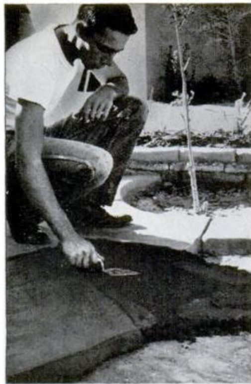
Concrete flagstones hand-troweled on the spot let you lay your patio on the installment plan
