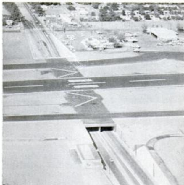
VAN NUYS AIRPORT , one of the exclusive businessman's airports, built runway over 4-lane highway
