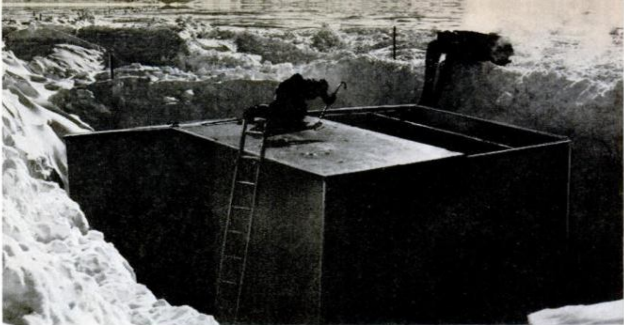
NEW BUILDINGS go up at Pole Base in deep pits. Snow is bulldozed over top to make level, driftproof surface
