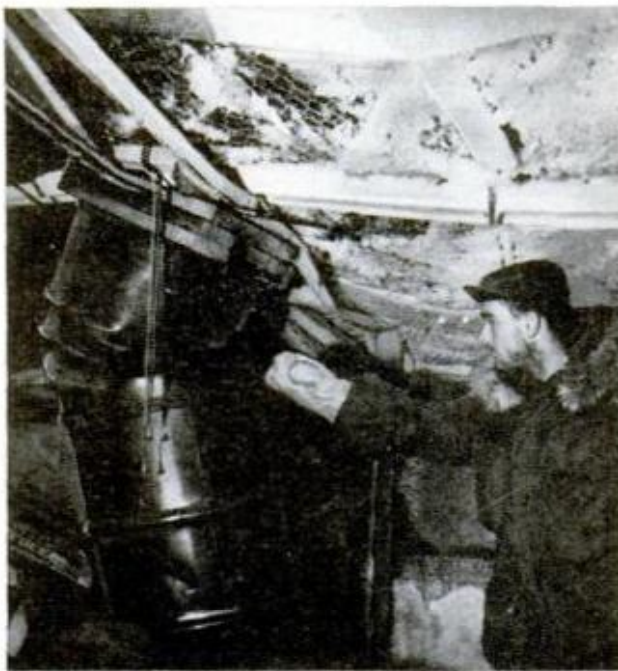
HEAVY DRIFTING over buildings at Byrd Base has started cave-ins. Even welded oil drum columns are buckling under 15 feet of ice and snow
