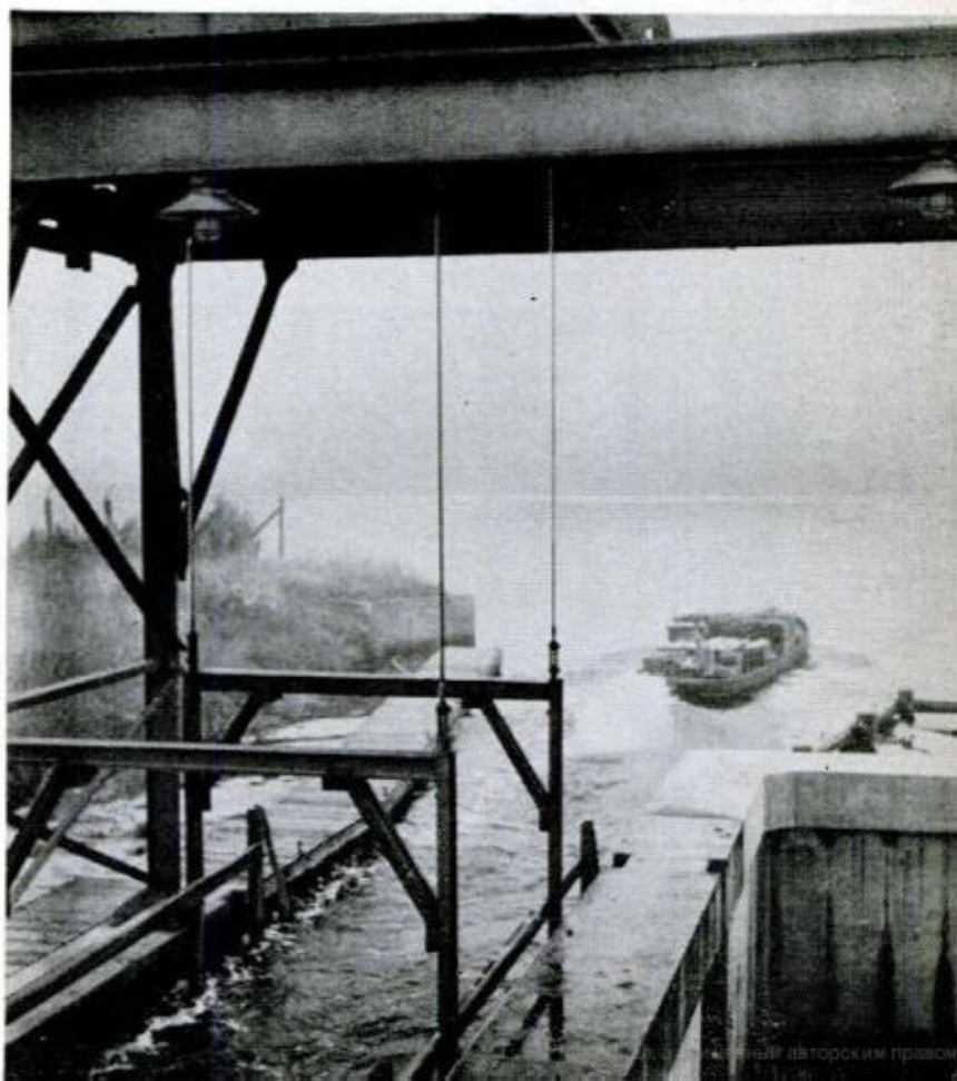
NEAR AMSTERDAM , a boat elevator lifts boat—pilot and all—out of a slip at one canal level, then rolls it across the dam to another, parallel slip at the next canal's water level
