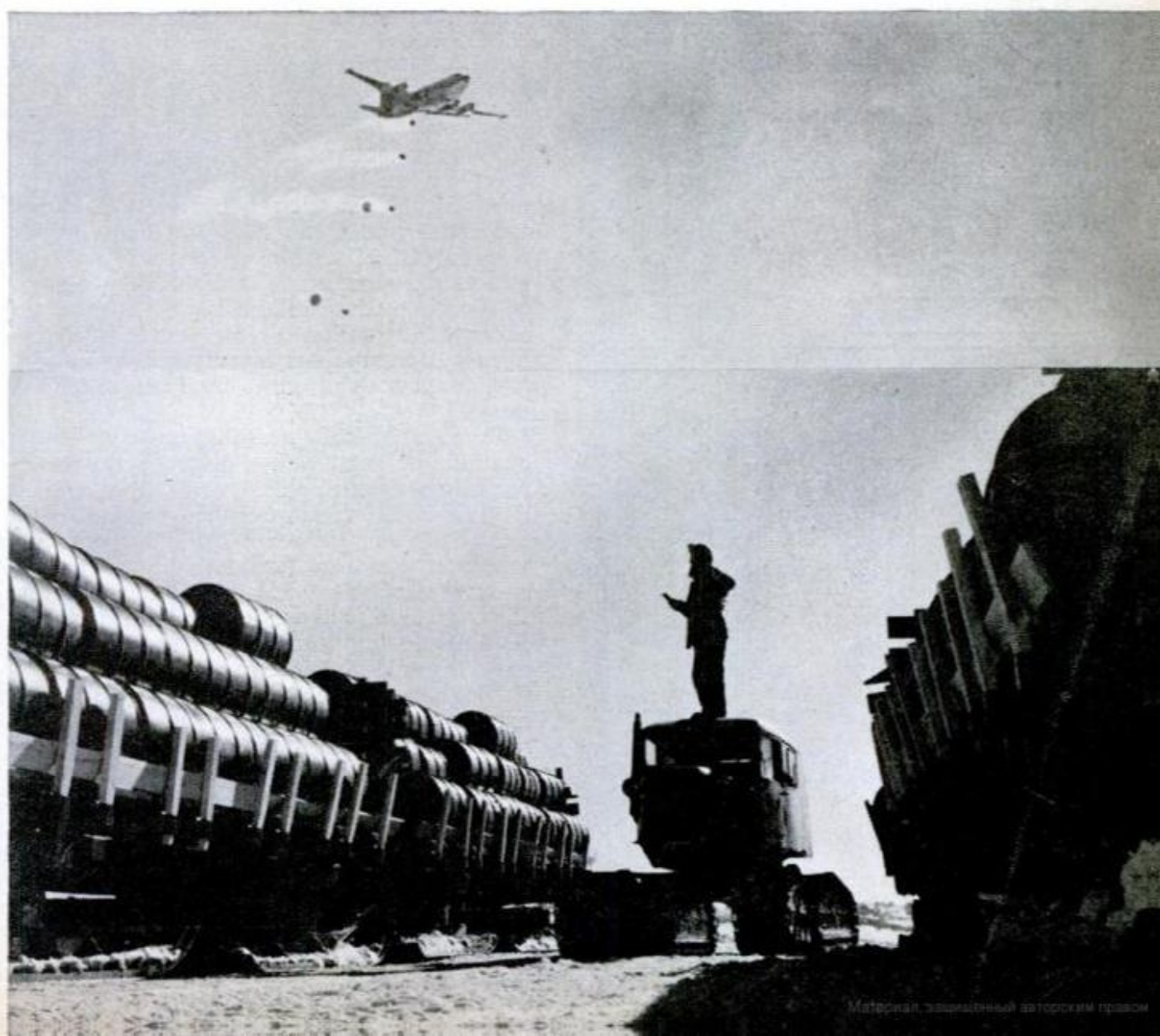
HERCULES C-130 propjet cargo planes whine through icy Antarctic summer, delivering oil and other supplies to inland bases. The boxcar-sized planes can land on skis. Engines must be kept turning in the thin air. The condensation cloud at -55 degrees F. spews for miles. Below Air Force Globemaster drops oil drums
