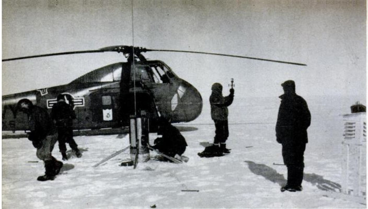
HELICOPTER CREW sets up an automatic weather station to lessen the hazards of flying over Antarctica's featureless ice. The station, at position Alpha-1 on route to Byrd Base, gives homing signals. During the polar night, below, the crews check the snow-drifted condition of lashed-down planes in -70 degrees F. weather
