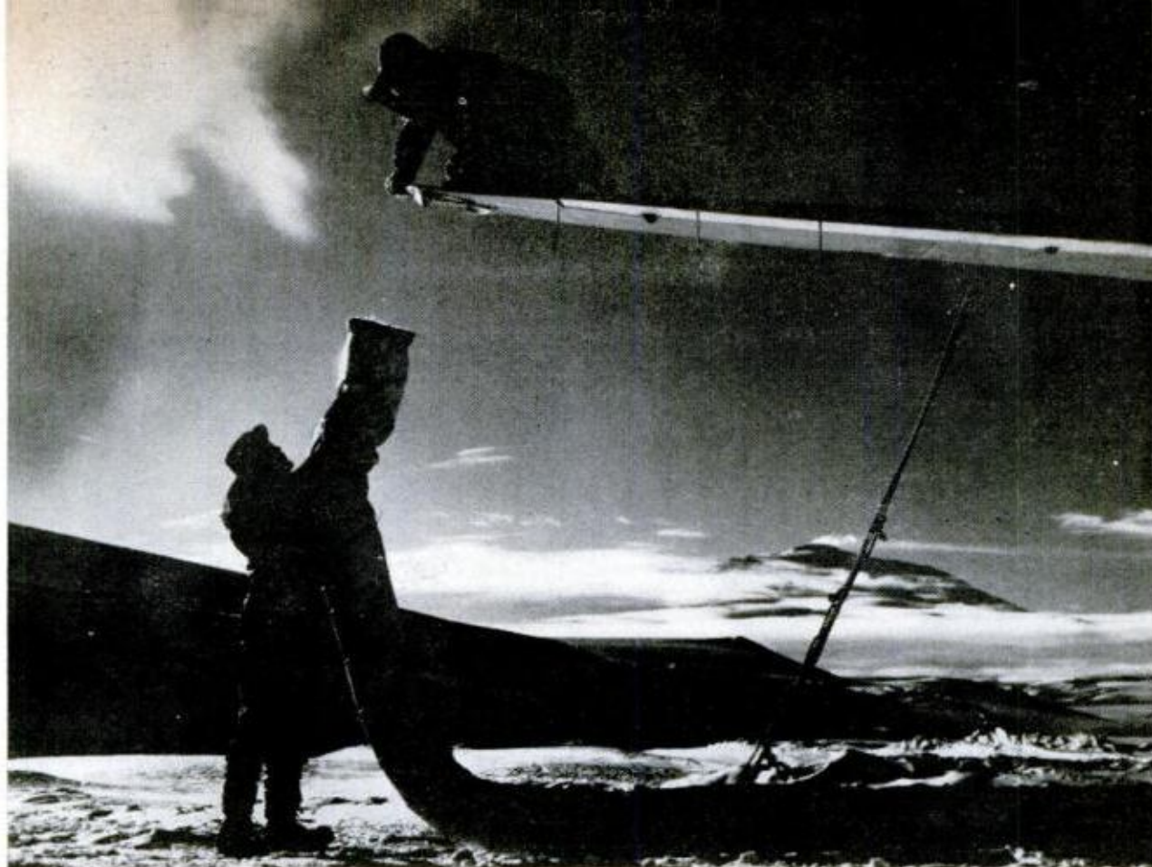
MAINTAINING PLANES in deep subzero cold takes a rugged constitution and ingenuity. A blast of air, above, is played over mechanic and wingtip during reactivation of R4D in polar dawn. Navy mechanics, below, perform an engine change on an R4D, the "Wilshie Duit," that came down 1500 miles out on polar plateau
