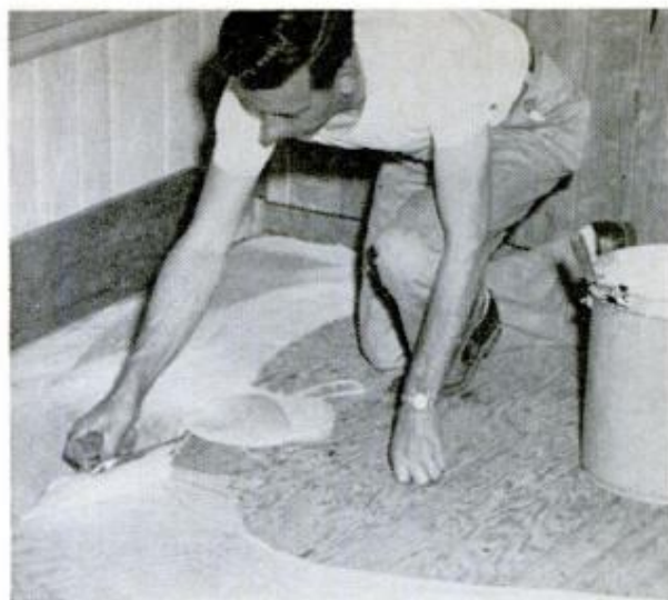
STEP 1. Carefully trowel adhesive on one quarter of area. Work close but do not cover the chalk lines
