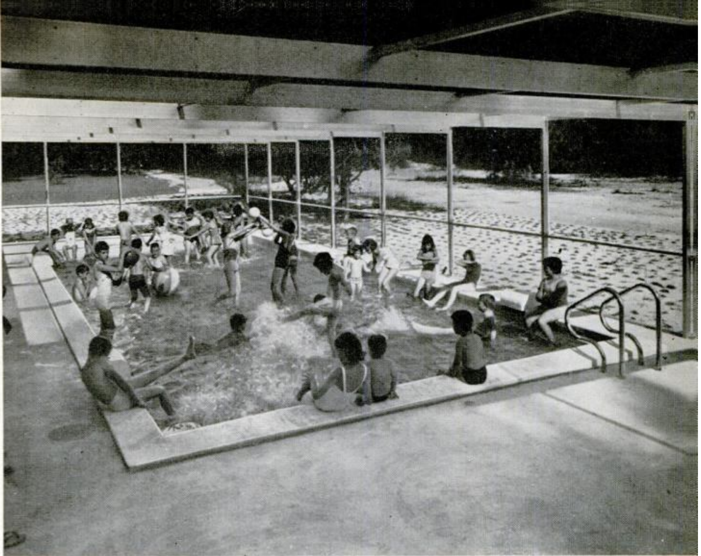
WADING POOL is obtained by lowering patio a few inches. Up and down movement is controlled by motors
