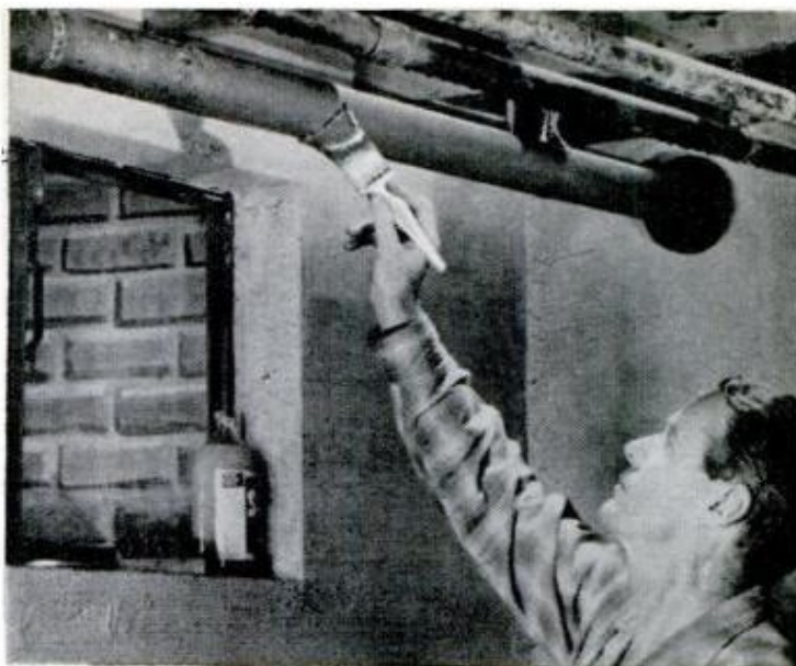
BASEMENT WATER PIPES need painting regularly with rust-resistant metal paint
