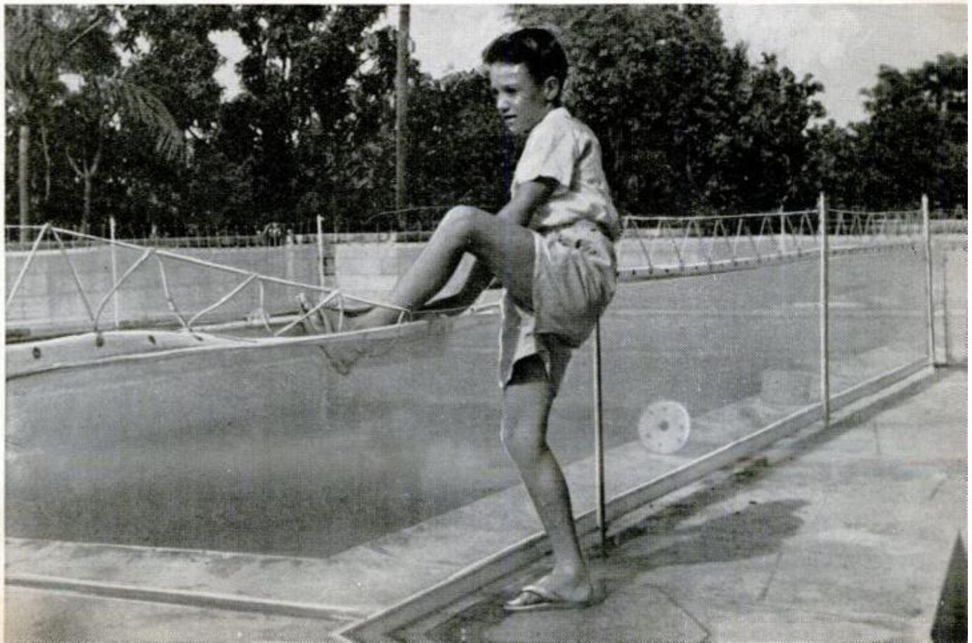
NYLON FENCE has a wire strand running along top and bottom. Inventor Fazio, left, shows bell that rings loudly when the top strand is depressed as some youngster attempts to enter pool. Fence is snapped closed
