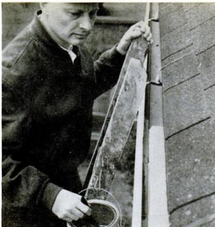
SCRAPE AND BRUSH inside of roof gutters before applying coat of antirust primer
