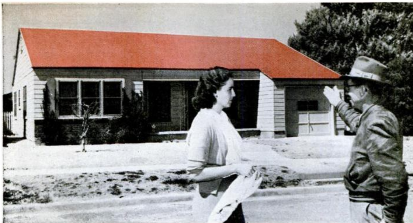
J. L. Wadleigh says Uniflex Colored Aluminum Coating will add at least another ten years of service to this roof. Uniflex is made by Alcoa Refining Co., Cleveland, Ohio.
