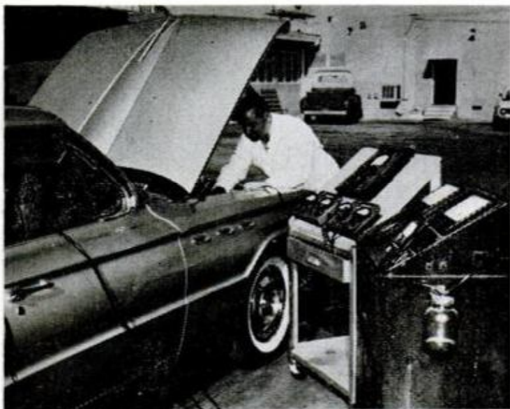
PM TEST CAR , above, is being linked to dynamometer controls. Report of its performance, with and without supplement, is shown on opposite page. Below is the rig which R. N. Metcalf, supplement manufacturer, uses to test mileages of fuel samples. Ten percent increase usually is obtained with supplement
