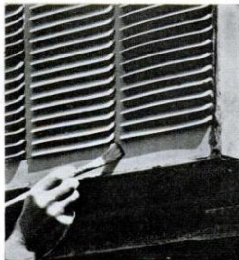
SCRAPE AND BRUSH inside of roof gutters before applying coat of antirust primer
