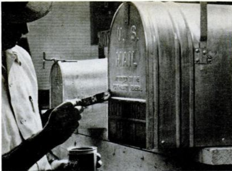
ALUMINUM PAINT with antirust properties is popular for painting rural mailboxes. Clean first with steel wool
