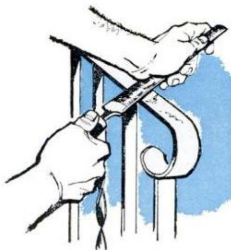
FILE WILL REMOVE those little domes of rust and smooth ironwork for repainting
