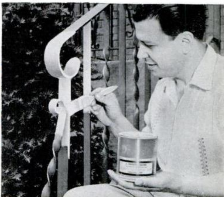
FILE WILL REMOVE those little domes of rust and smooth ironwork for repainting
