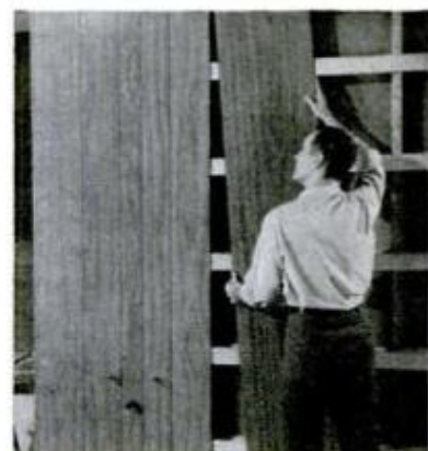
Each tongued-and-grooved plank (16" x 8" x 1/4") goes up over furring strips or existing walls without muss or fuss.
