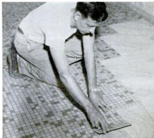
STEP 3. Do not twist or slide the tile in position. Butt edge snugly against adjacent tile and press down
