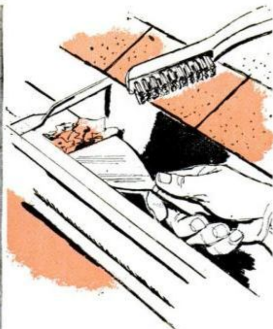
SCRAPE AND BRUSH inside of roof gutters before applying coat of antirust primer
