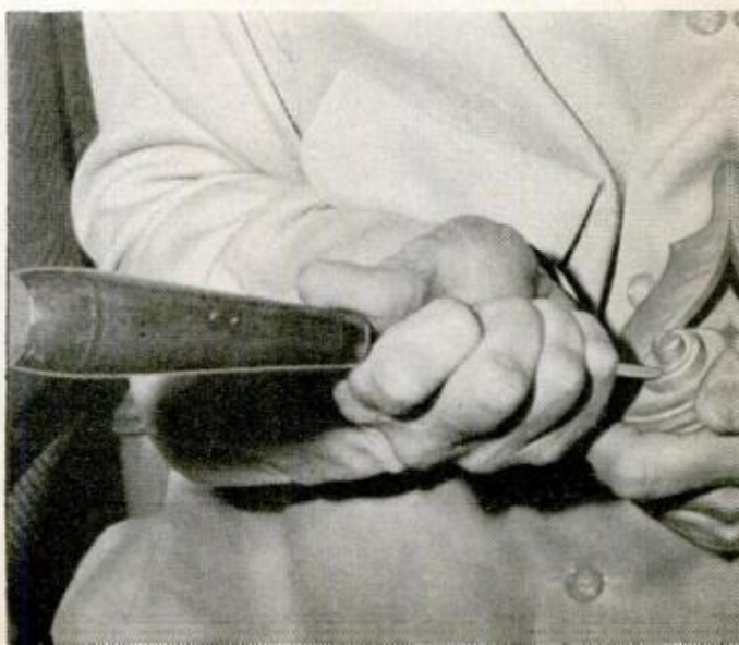
6. Scroll is finished by hand, and it is here that master violin makers work in small degrees of difference. Hand saw cuts it to rough shape
