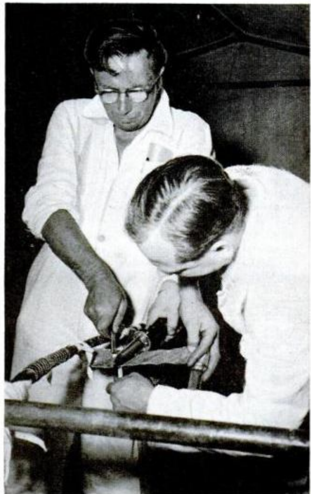
Bearded cableman winds armor wire over a splice. Below, critical wrappings are done in a tent on deck
