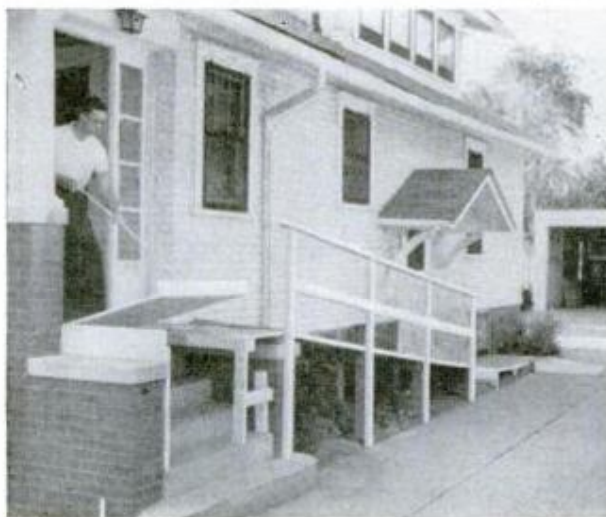
PLYWOOD PLATFORM IS LOWERED into position by rope to connect head of ramp with porch floor. Platform is stored on porch when ramp is not being used
