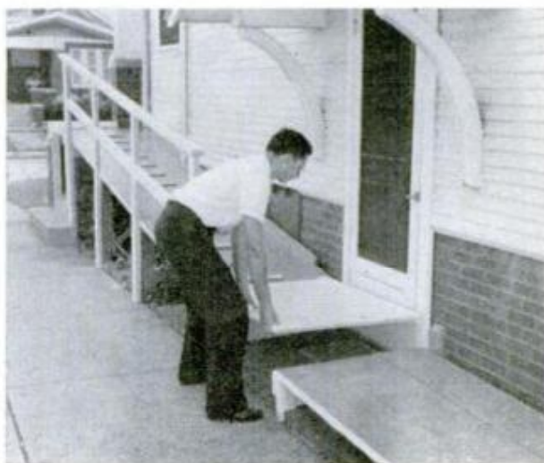
HINGED "DRAWBRIDGE" across side entrance is swung back onto ramp when latter is not being used so that door can be opened without interference
