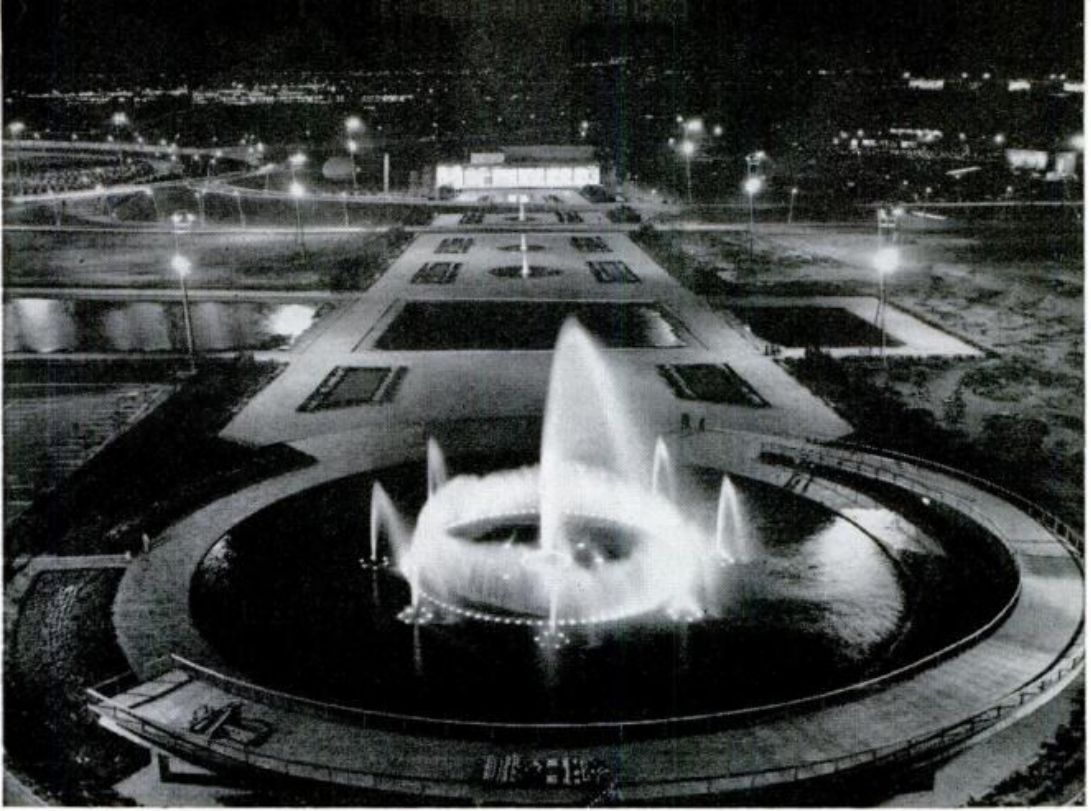
Here is view from control tower, facing into heart of Terminal City, 655-acre service center of the field. Past the lighted fountain is a $7,000,000 heating and air-conditioning plant. It displays colorful pipes
