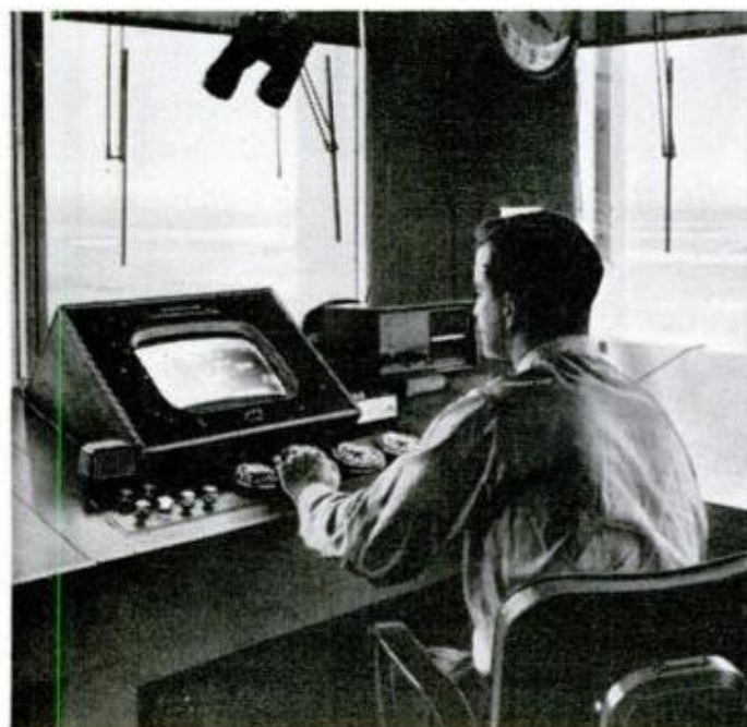
Operator on ninth floor of tower monitors the arrival board via closed-circuit television, and posts times
