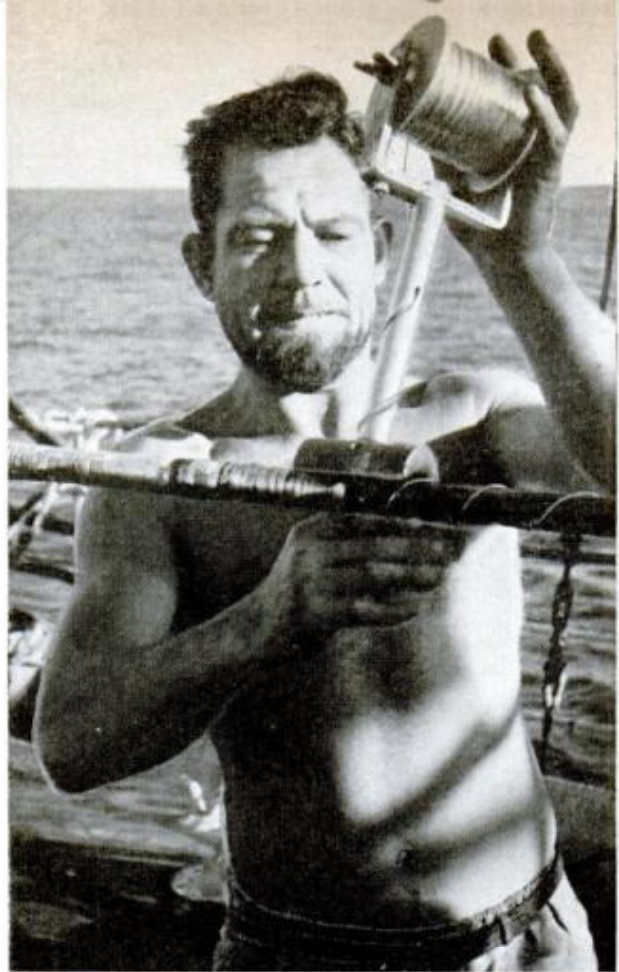
Bearded cableman winds armor wire over a splice. Below, critical wrappings are done in a tent on deck
