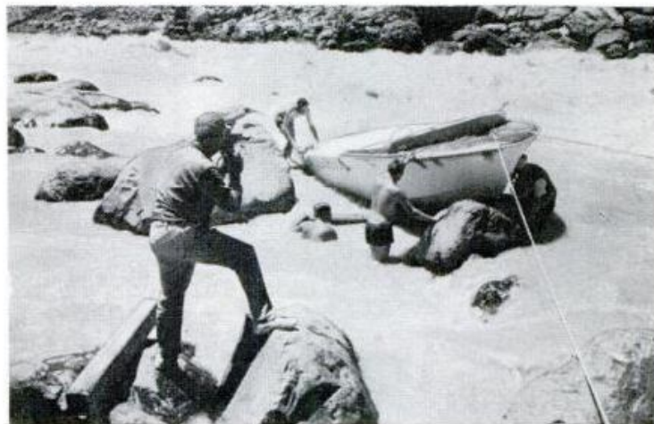
Big water flexed its muscles and tossed this boat clear out of the river. The tough plastic hull survived, and the jet system, all inside the hull, wasn't damaged. All hands turned to, shoved it back into the current and drove it away. Below, another boat hangs up in the rapids
