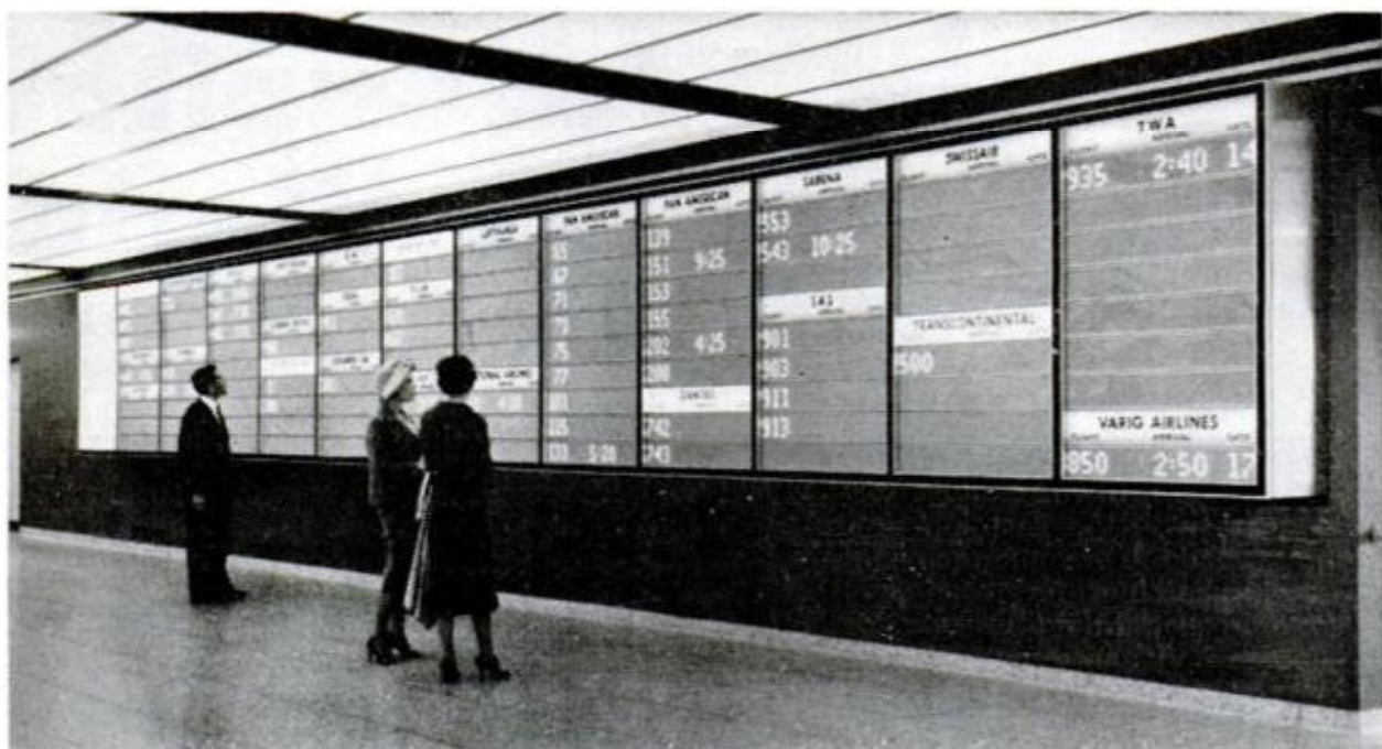
Arrival information board is remotely controlled. It can quickly display news about 94 flights of 25 airlines
