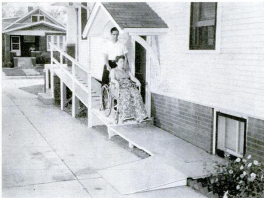
PLYWOOD PLATFORM IS LOWERED into position by rope to connect head of ramp with porch floor. Platform is stored on porch when ramp is not being used
