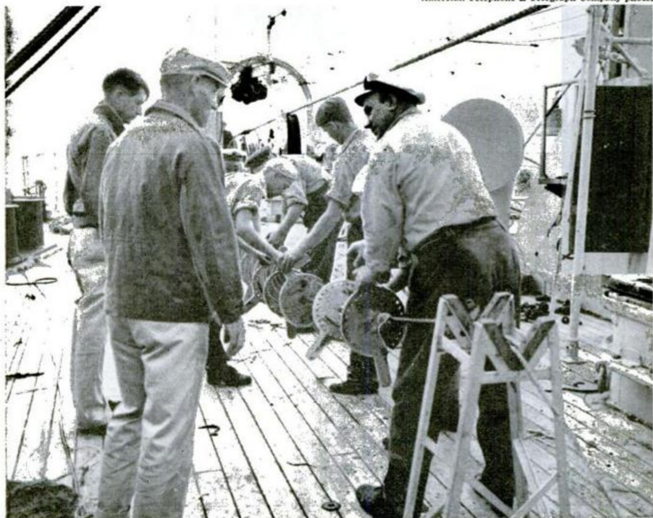
Tricky job of lifting and lowering the cable without changing the tension is helped by this tension drum. Using stripping disks to keep all the wires separated and in order, all hands fall to stripping a new section
