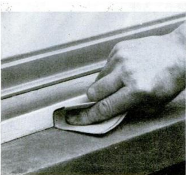
ROUGHEN SURFACES with coarse sandpaper or coarse steel wool. Rough surface promotes adhesion of calk
