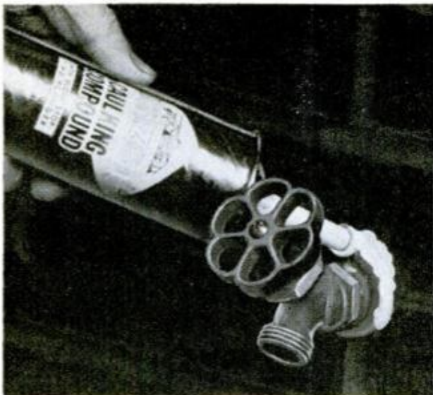
OPENINGS AROUND SILL COCKS, lead-in wires and clothes dryer vents need calking to keep out moisture
