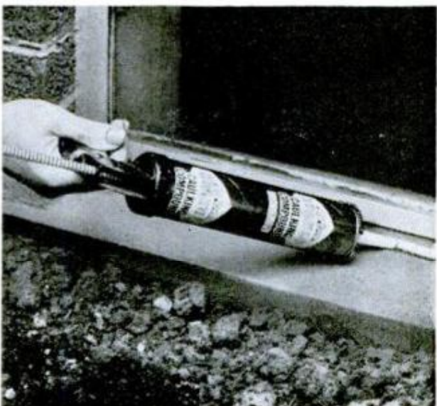
PAY PARTICULAR ATTENTION to metal casements, such as basement windows, where moisture is found
