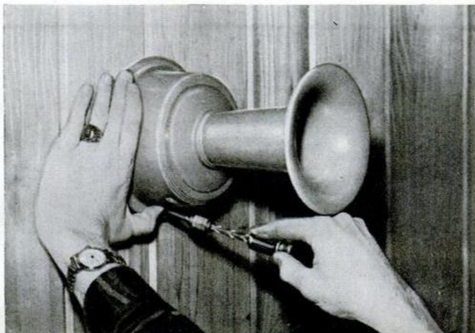
Panel and bell tell location of house fire; push-switch tests unit. Outdoor horn notifies neighbors
