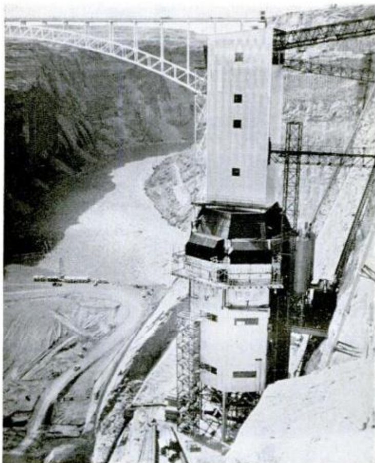
Before tunnel was built, trucks were lowered to river bed by cables. Below, concrete mixing plant rests on canyon shelf
