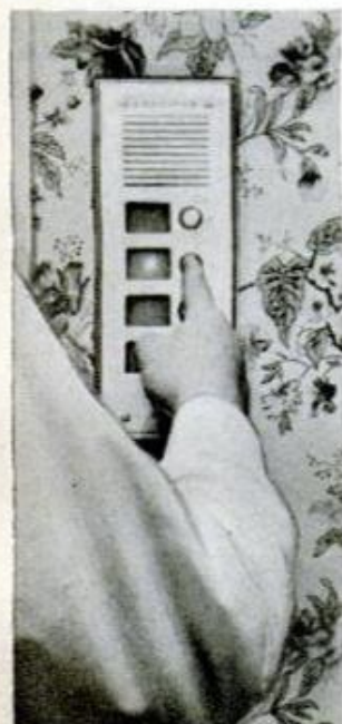
Panel and bell tell location of house fire; push-switch tests unit. Outdoor horn notifies neighbors
