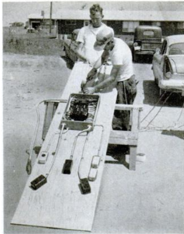
Prebuilt electric panel will be one component of future wall. Other panels will "plug into" this one
