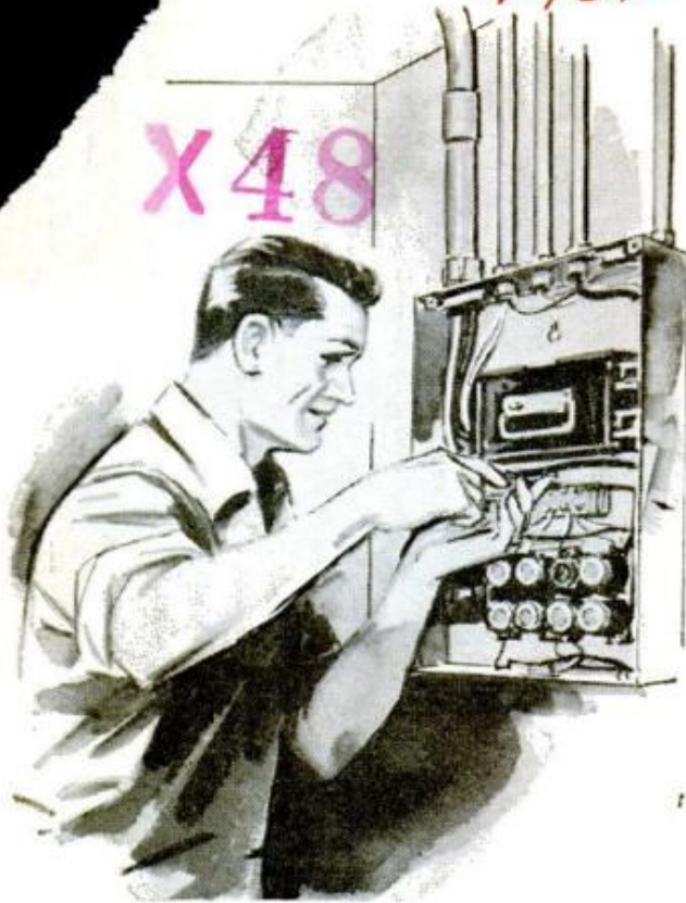
NEW CIRCUITS for light and power can be tapped-in at service entrance or into a branch circuit box
