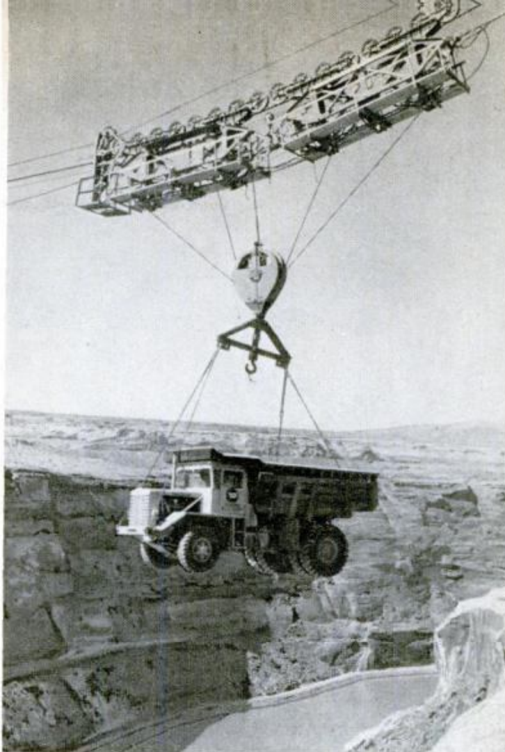
Before tunnel was built, trucks were lowered to river bed by cables. Below, concrete mixing plant rests on canyon shelf
