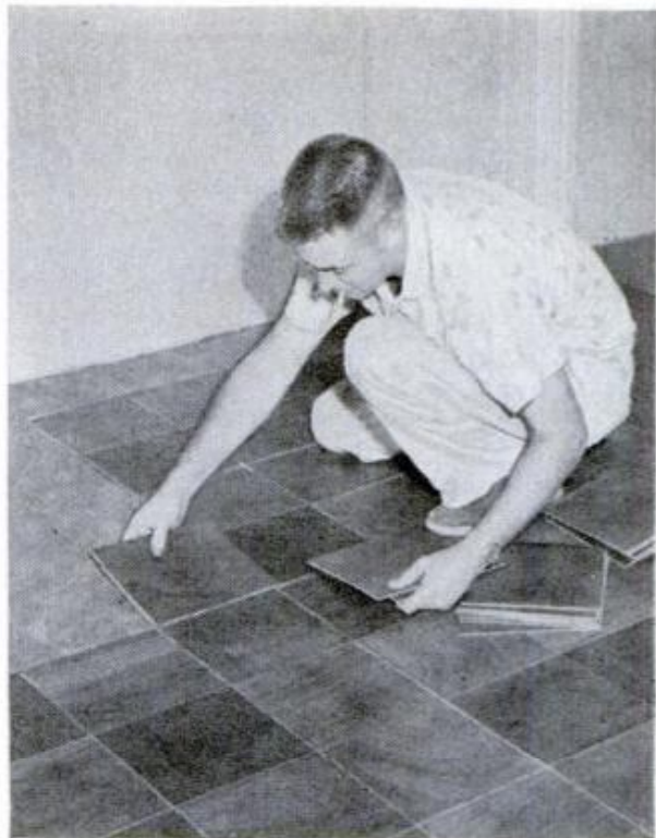
Fibers of these real wood tiles are stretched and dried, making tile flexible and dimensionally stable
