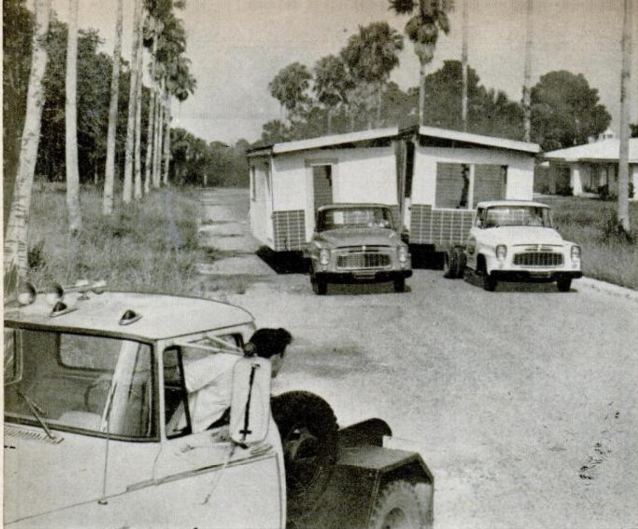
Halves of a manufactured 680-square-foot ranch house are hauled by truck to the buyer's building site
