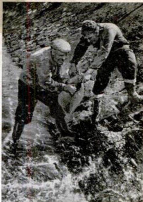
Water is splashing around the wall when Jan closes the gates which shut off the road leading to the harbor on top of the dike. Since the sea has already weakened the dike walls, Jan and son jam sandbags into the gap, right. Dike watchers employ telephones and trucks for quick operations throughout maintenance system
