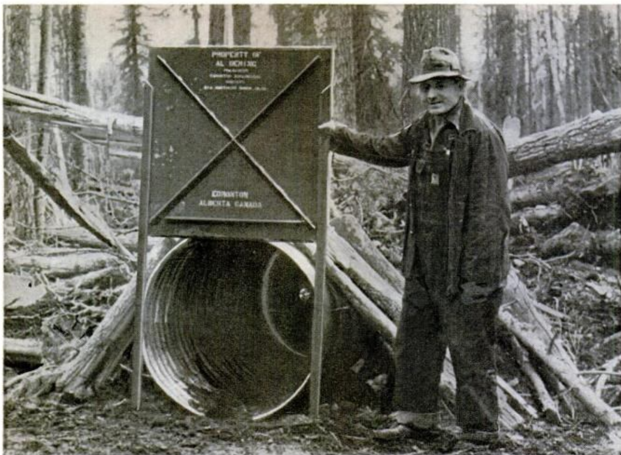
Ten-foot length of steel culvert provides grizzly trap body; door drops over opening when trigger is touched
