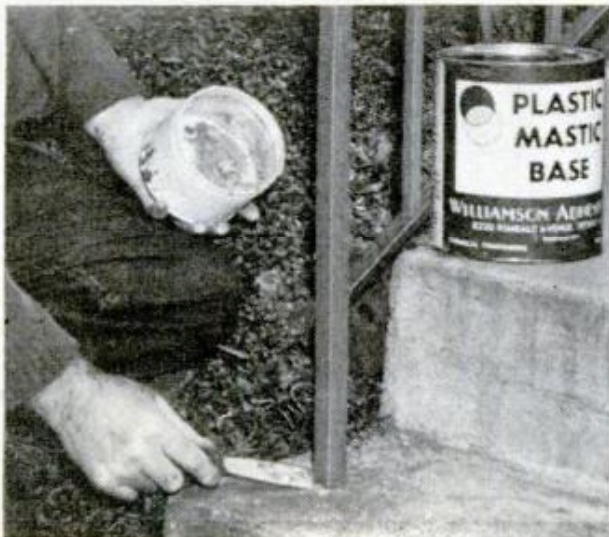
1. Mastic-type compound used to cement loose railing in step as shown, is fine for metal-to-metal joints
