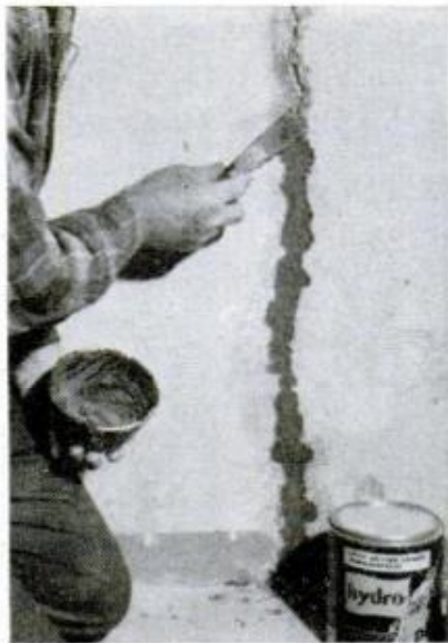
6. This fast-setting two-part compound is ideal for cracks where moisture is present, as in basement
