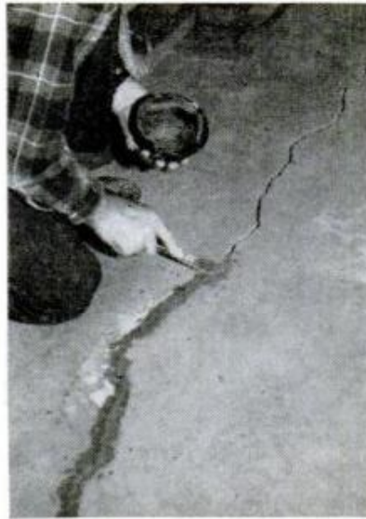
6. This fast-setting two-part compound is ideal for cracks where moisture is present, as in basement
