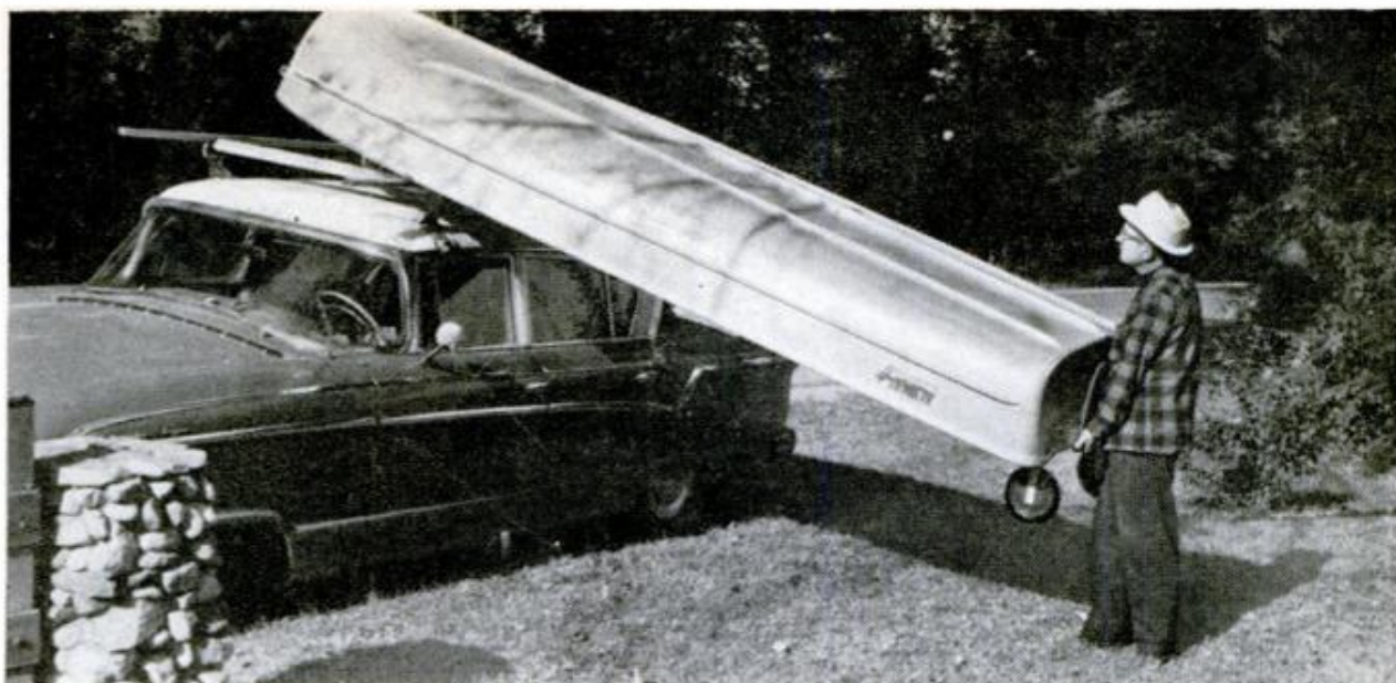
Car-topped boat is easy to unload and wheel to water's edge when wheels are mounted temporarily on transom
