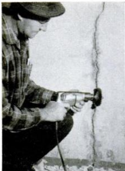
6. This fast-setting two-part compound is ideal for cracks where moisture is present, as in basement
