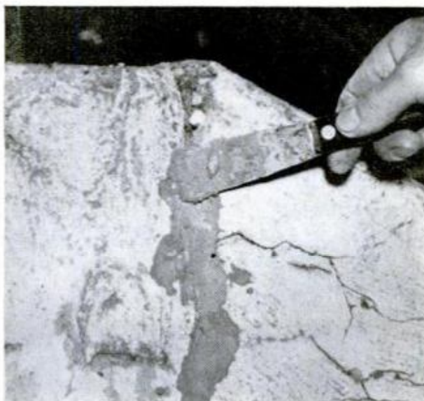
9. Fine cracks in concrete are widened slightly to give patching compound a better chance to anchor
