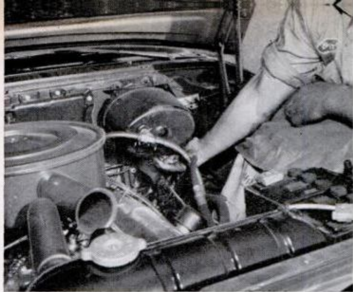
Checking master cylinder on a Plymouth with power brakes is tough. It's hidden under the power assist and can be felt but not seen by service attendant
