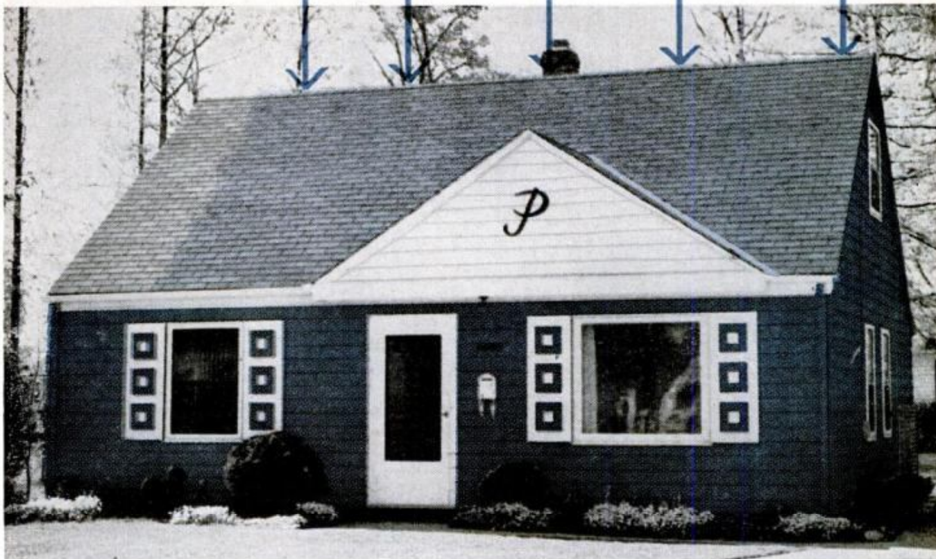
John Primeau chose blue Masticote to match his house. Masticote is made by The Madison Paint Co., Cleveland, Ohio.
