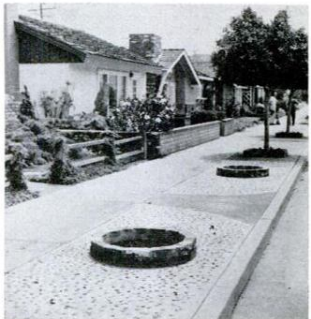
Clean, quiet dignity is achieved on this street front by a combination of pebbled-concrete paving and shade trees. Wells for the trees are of alternating red and gray bricks, offering a colorful contrast to the somewhat severe aspect of the paving
