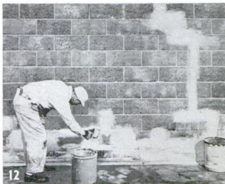
Above, after the puttied spots are moistened with water, they are concealed by coating them with sealing compound. Below, rest of wall is coated, moistening it first with water
