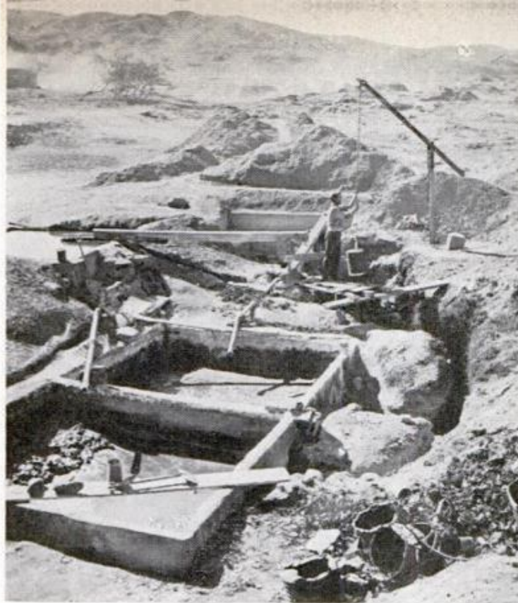
Gaston built equipment for copper mine in northern Chile's Atacama Desert. Salt water poured over ore dissolves out copper sulphate; sulphate is precipitated out of solution later
