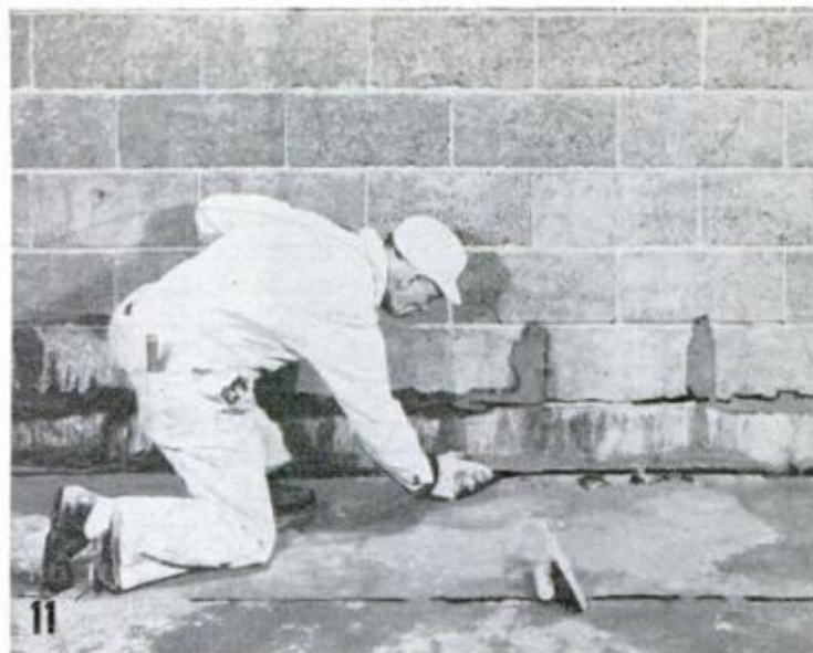
Joint where wall meets floor is plugged last. Weep holes in blocks are left open until wall is coated with sealing compound
