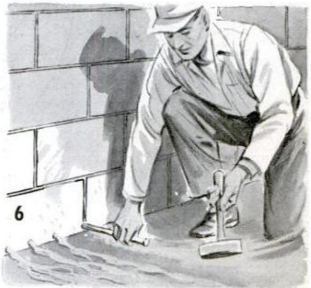
Water trapped in cores of block foundation is drained through weep holes made in the blocks at the floor line. This relieves pressure, makes filling holes easier
