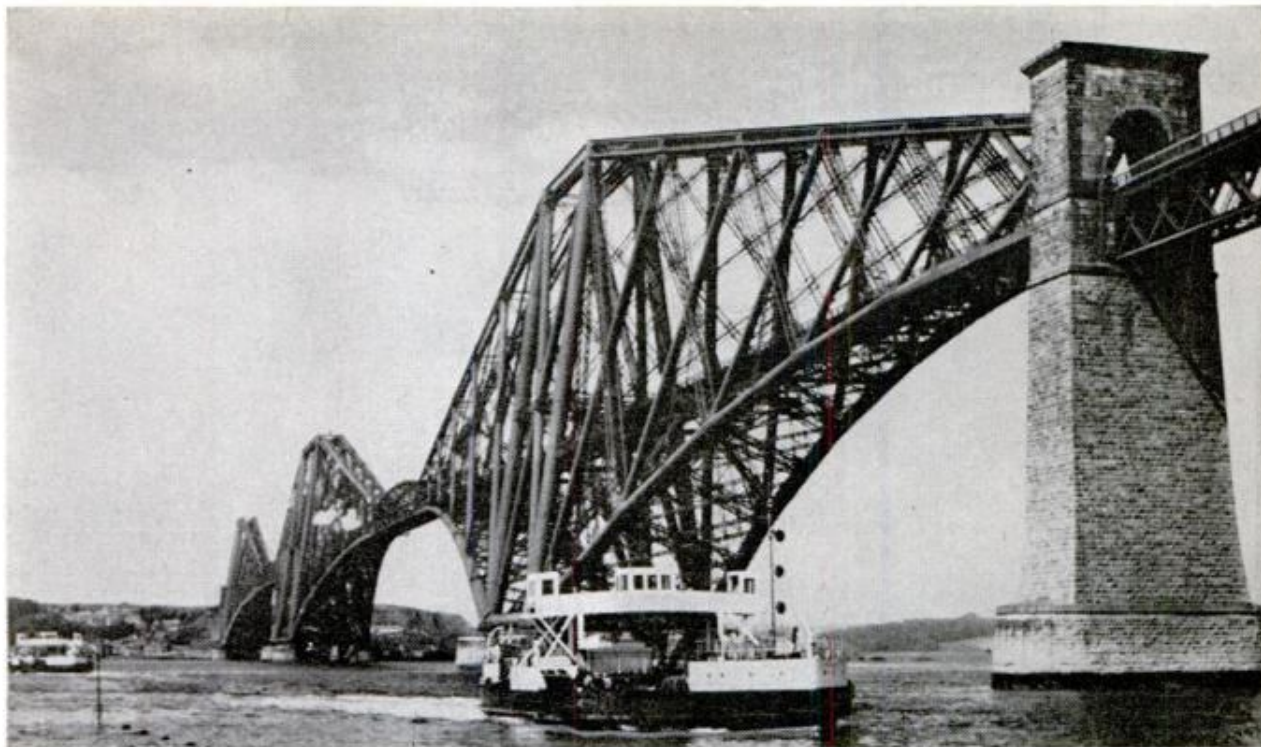
Old railroad bridge across the Firth of Forth for a generation was the longest span bridge in the world
