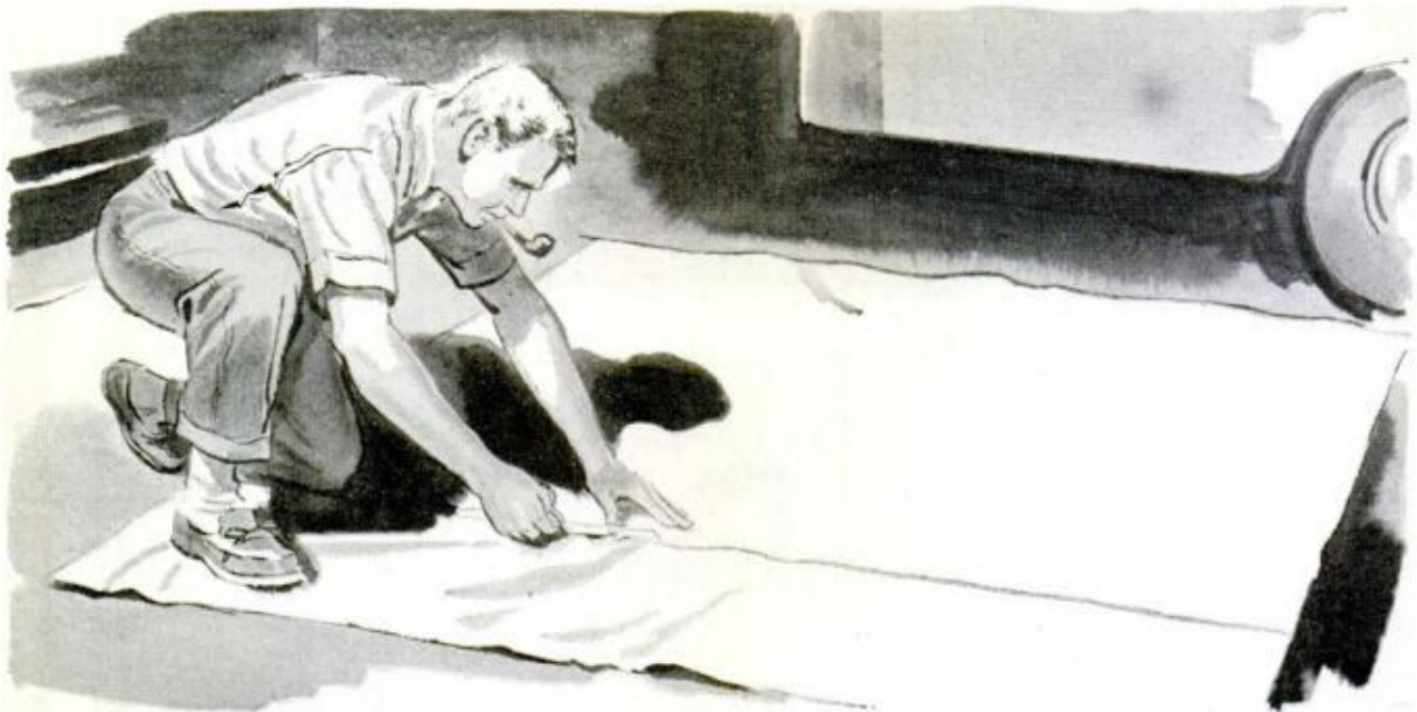
Spread glass-fiber fabric on a flat surface, the garage floor will do, mark size and cut with scissors
