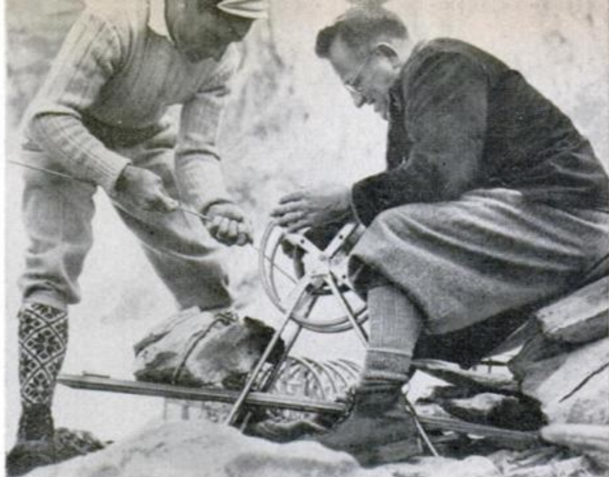
Base crew secures cable at bottom, stretching it taut with winch
