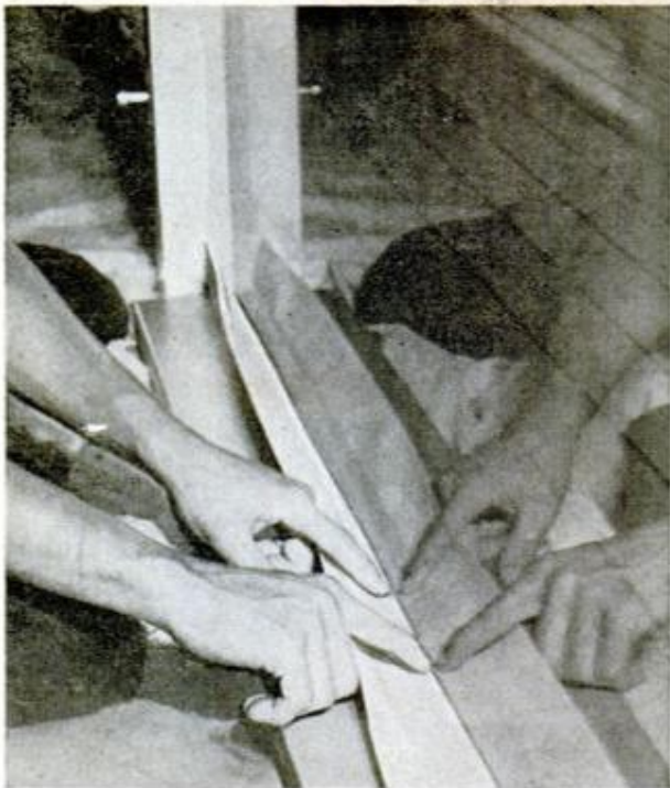
1. As the emulsion flows down the window a certain amount of overflow is unavoidable. To catch it, a trough of moistureproof butcher paper is used
