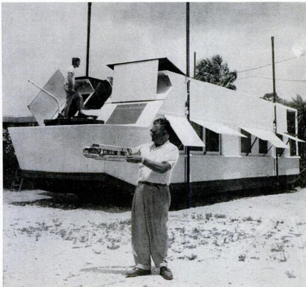
Dr. Johnston holds the original scale model. In the background, son Bill stands on the finished foredeck
