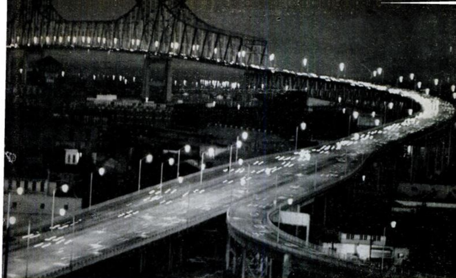
Junction of the Greater New Orleans Expressway and the Greater New Orleans Bridge over the Mississippi.
