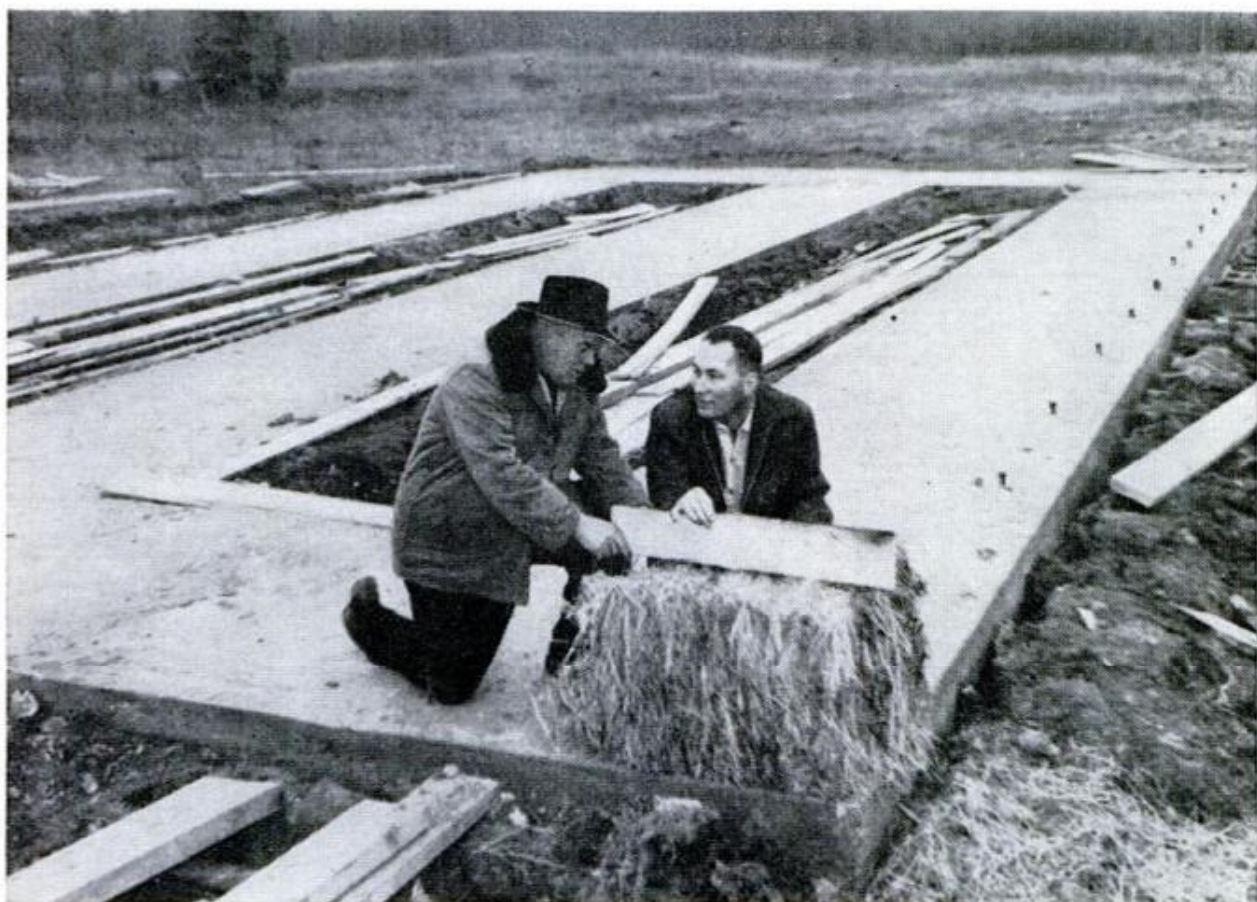
Bales of straw—plentiful around Sexsmith which claims to be grain capital of the British Empire—placed on concrete form the walls. Below, with steeple in place and the walls stuccoed, the chapel is almost finished
