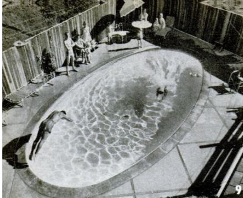
Without diving board or ladder, this 30-ft. glass-fiber pool costs about $3000 installed in areas close to manufacturer
