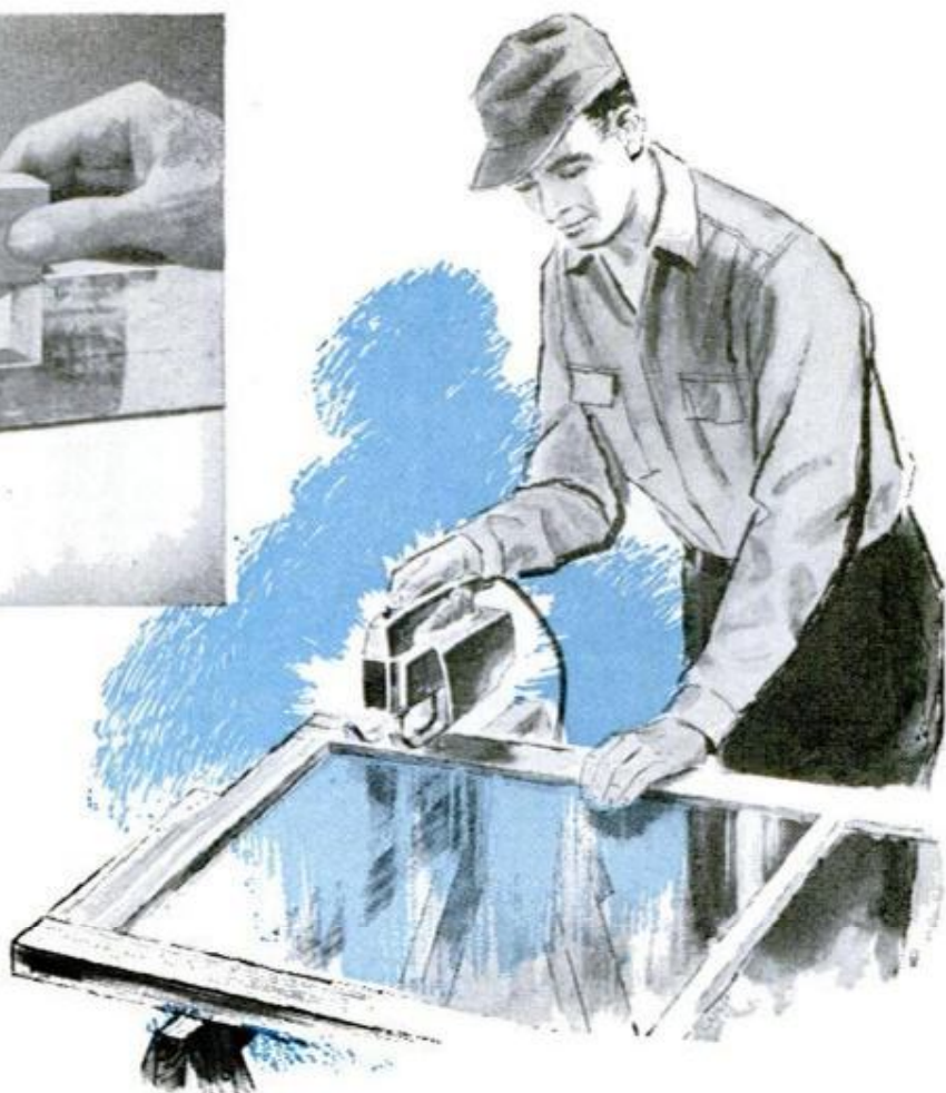
Rotted wood cut from sash is replaced by new wood cut to fit
