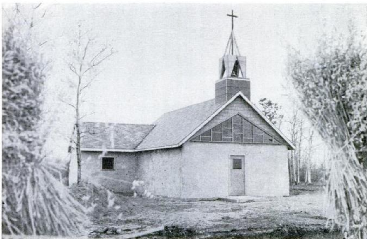
Bales of straw—plentiful around Sexsmith which claims to be grain capital of the British Empire—placed on concrete form the walls. Below, with steeple in place and the walls stuccoed, the chapel is almost finished
