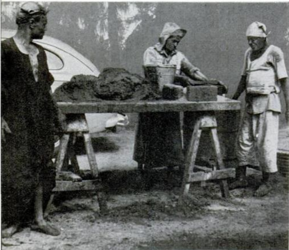
Egyptian farm workers mix mud with a petroleum by-product, bitumen, which makes their mud huts resistant to rain. ADL suggested the technique as a means of helping solve a housing problem for over 16 million workers
