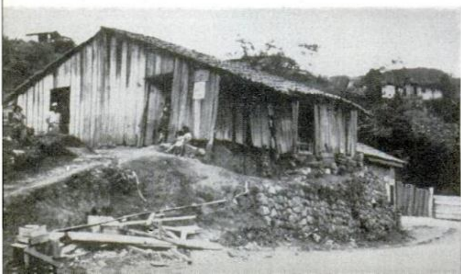
..... Before: Some Hondurans lived in ramshackle houses made of wood and ADL's problem was to find how they could help make their own houses at low cost
