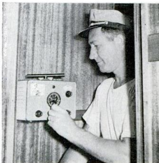
Below, radio direction finder was mounted on the forward bulkhead in the Sea Joy's head, which saw double duty as radio room. This kit-built unit also has a standard broadcast band for music and news
