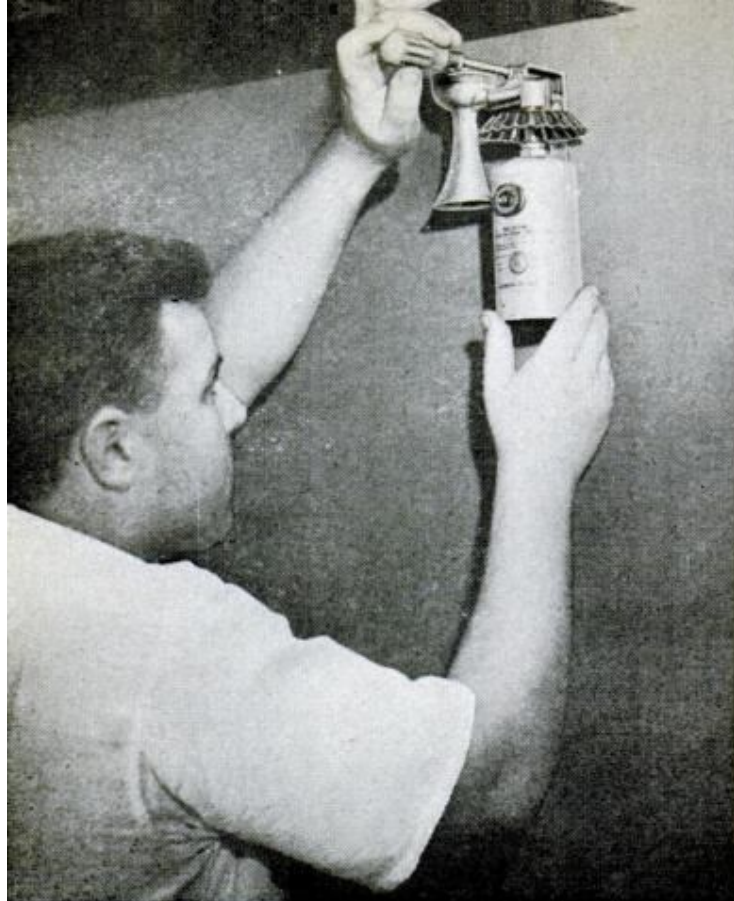
Individual pressurized horns can be mounted anywhere in the house. Heat sets off loud blast of horn
