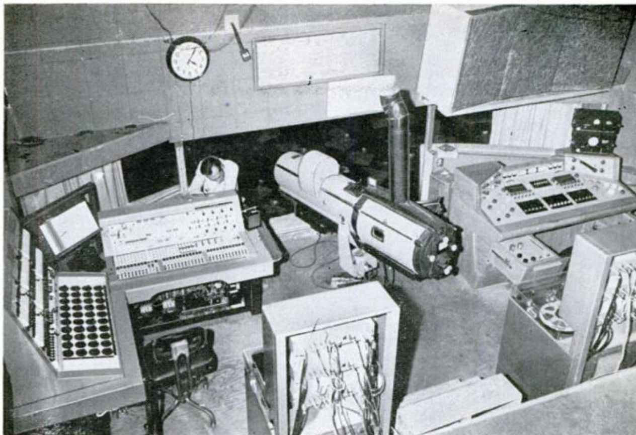
Interior of Stardust Hotel's show booth discloses an array of hi-fi controls, right, and lighting controls
