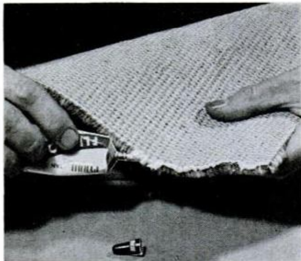
Bead of liquid rubber applied along cut edge of rug prevents fiber "fallout," serves as neat binding
