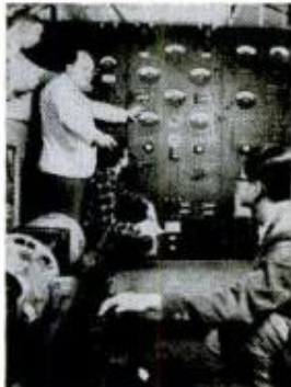
Photo of Heald Students in Electrical Laboratory
