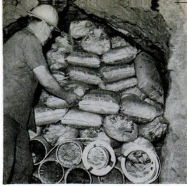
Atlas Powder Company engineers stuffed the tunnels at Promontory Point with 1½ million pounds of Amocol blasting agent spiked with 385,000 pounds of dynamite to insure total detonation. See the dramatic result at right
