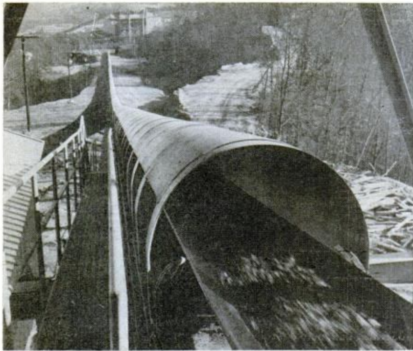
Rock, shale and other refuse extracted from the coal climbs a 2400-foot hill aboard one of plant's conveyors. At top, the load is automatically dumped and then spread into a valley
