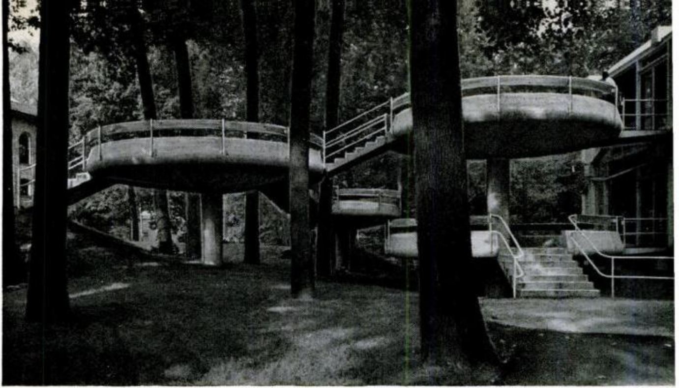
Four "lily pad" landings with their stairways enable students to get out of the building's second and third levels quickly. There are circular benches around the edges of each of the concrete structures at Commons
