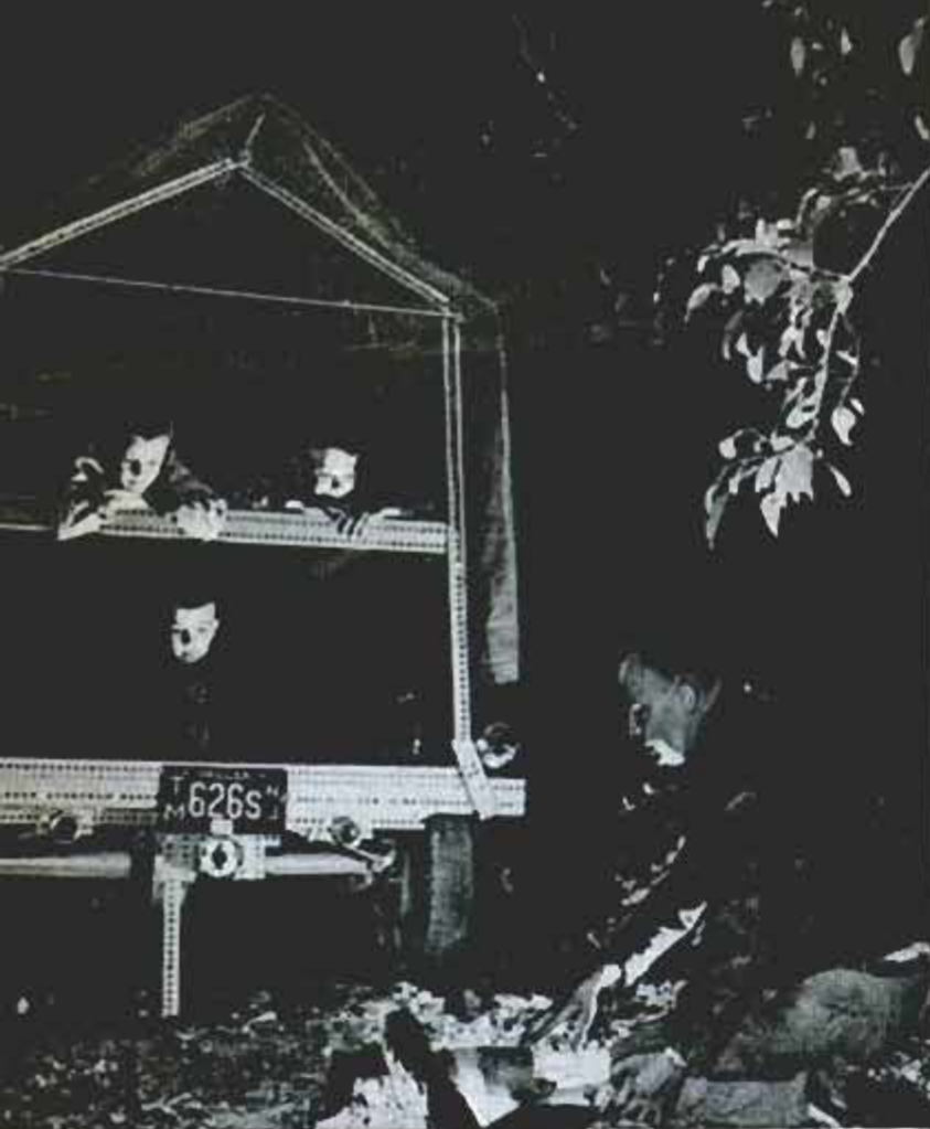
To add bunks to trailer, Metal Lumber bar is bolted down center and another piece is added across back. Canvas bunk platforms are rope-lashed through grommets to holes in side rails
