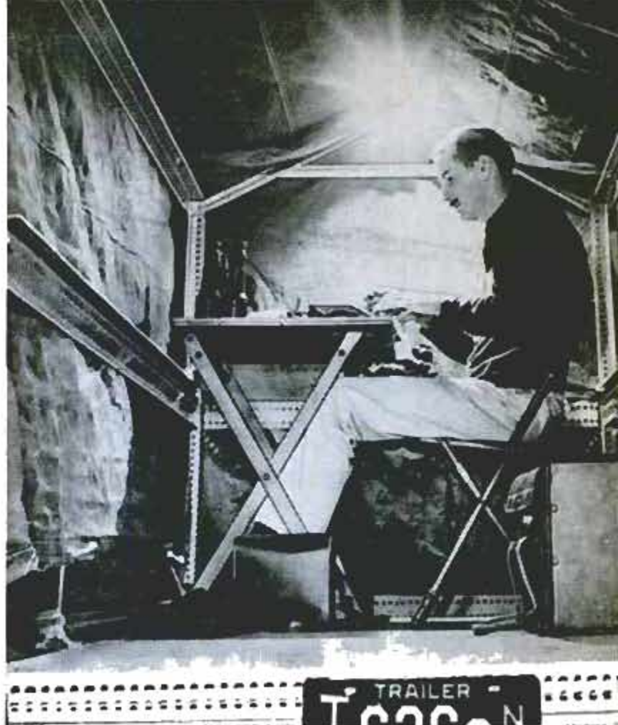
Office on boat trailer is five feet high. Peaked gable sections at each end are bolted in place, and lightweight ridge-pole of tubing supports canvas cover. Mobile rack below is example of how do-it-yourself steel is applied industrially
