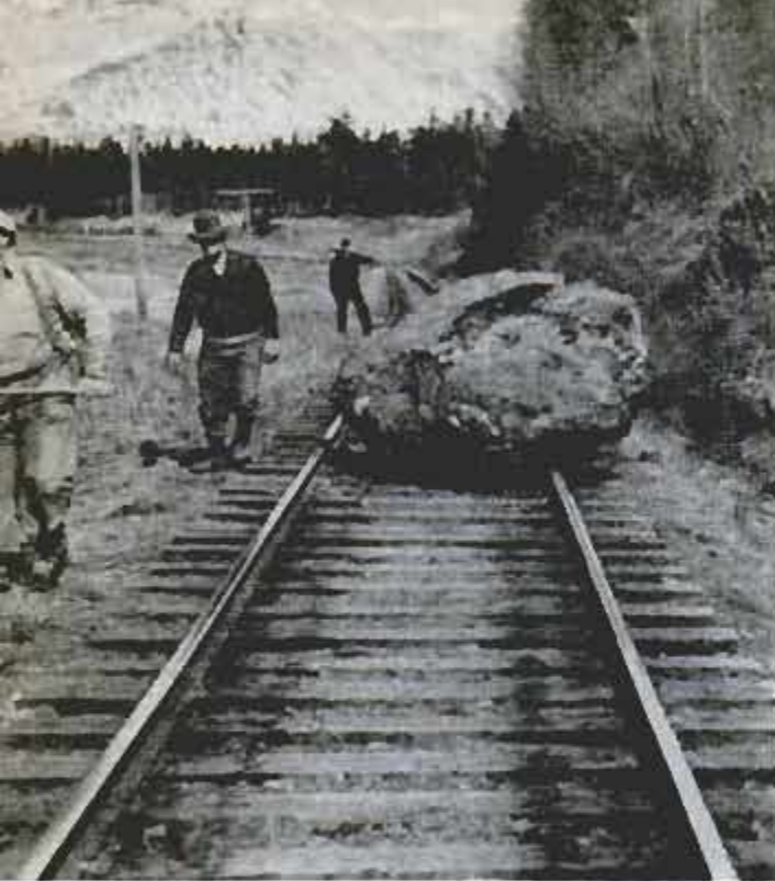
When glacial moraine thaws, mud slides send tons of boulders tumbling down on tracks for crews to remove
