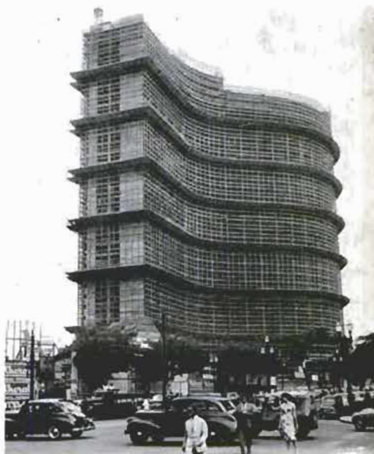
Huge office building under construction reflects Brazilian mastery of reinforced-concrete architecture
