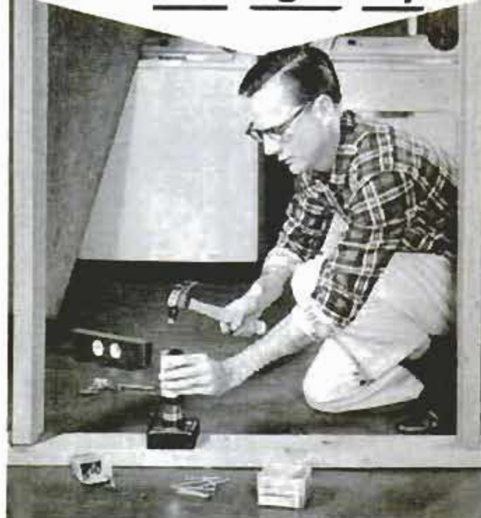
Anchoring 2x4 partition plate to basement floor.
