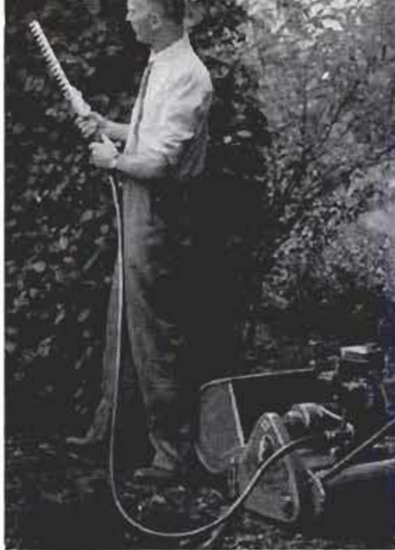
Left, flexible shaft powers the hedge trimmer. Right, rotary tiller is lightweight and easy to handle
