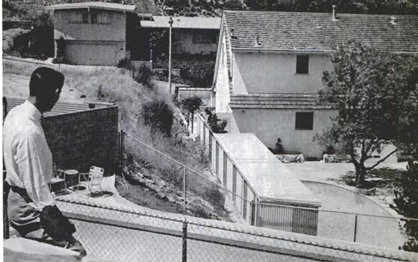
In yard above, the cabana wall is too high. Usually, back-yard walls may be no more than six feet in height. Furthermore, cabana is built too close to property line. This violates building code's side-yard law
