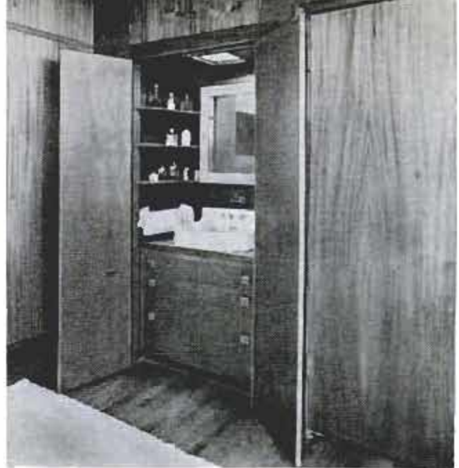
Bathroom capacity of a home can be increased by installing a lavatory in the master bedroom closet
