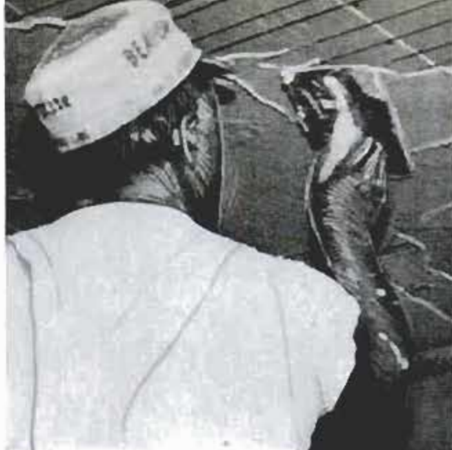
Coils are covered with plaster. Radiant heat warms plaster finish and radiates gently throughout room
