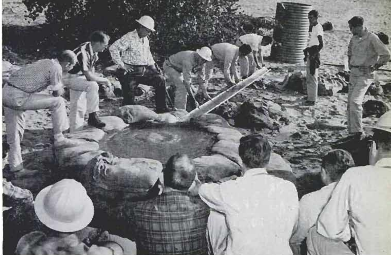
Operation of sand-bag chimney is explained to trainees. Device reduces flow of water and sand from boiler
