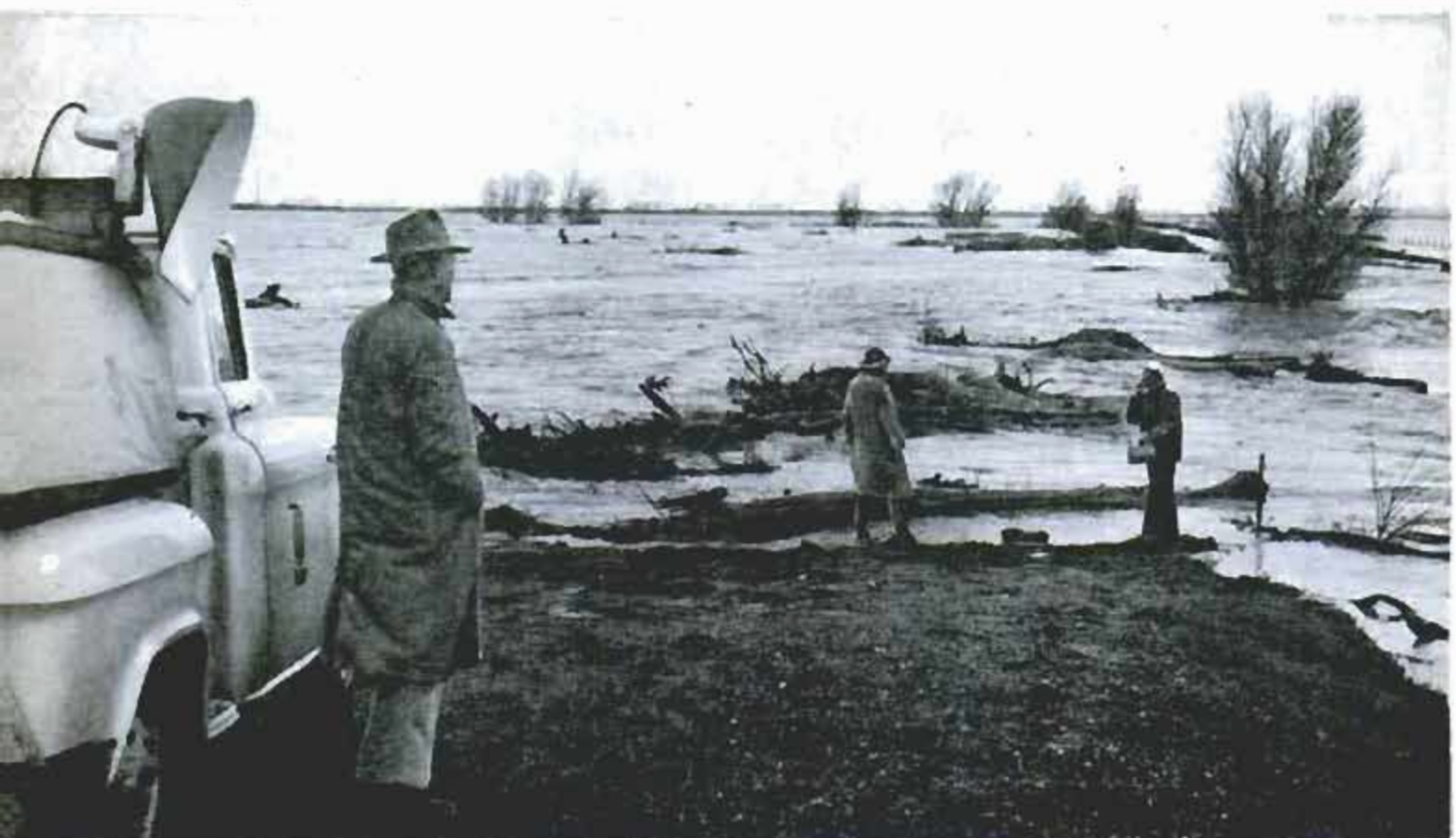
After break of Feather River, Yuba City, Calif., suffered big flood on Christmas, 1955. When Cache Creek threatened its levee on February 24, 1958, below, experts watched rise of stream to determine amount of wave wash occurring against levee. Truck carries public address system and flood lamp for night work
