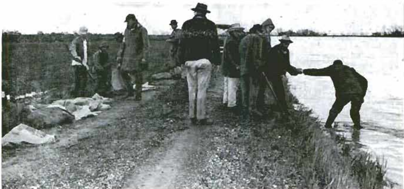
When Cache Creek reached critical flood stage, workers patrolled bank, feeling for washouts with feet
