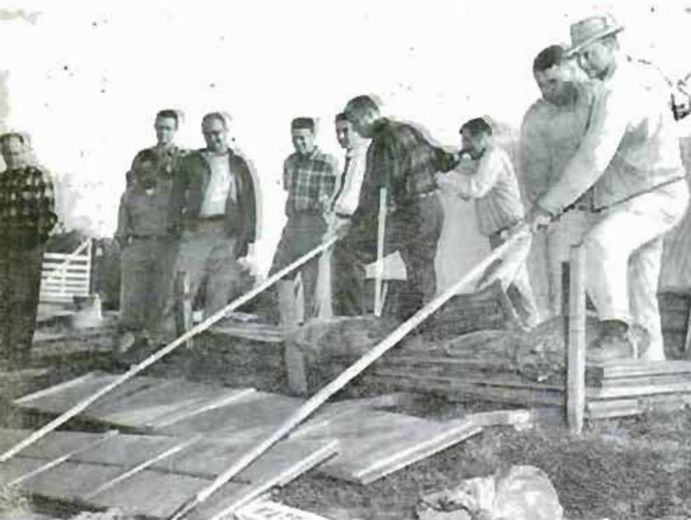
Practice session: Trainees learn how to prevent wave wash, which exists when waves, pushed by wind, strike at levee slope and tend to erode it. Panels laid on earth and held down by sand bags help prevent washout
