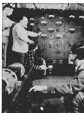
Photo of Heald Students in Electrical Laboratory
