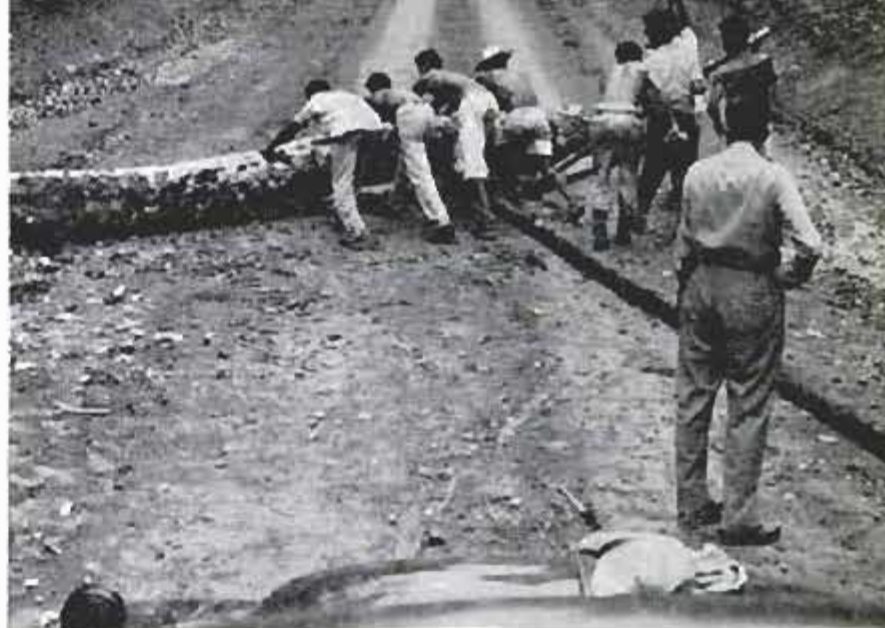
Tree is rolled away after toppling across the roadway. Thirty subposts are being set up along the road for maintenance
