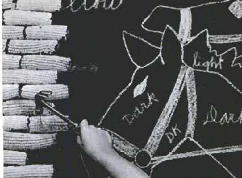
Following Howe's full-scale drawing and color guide, workmen nail split ears over pattern. Background is always yellow
