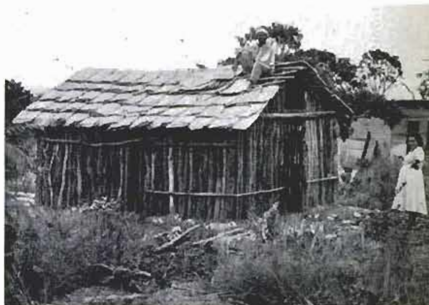
Farmer uses empty paper cement bags for house roof. Rains harden small amounts of remaining cement to make sound roof
