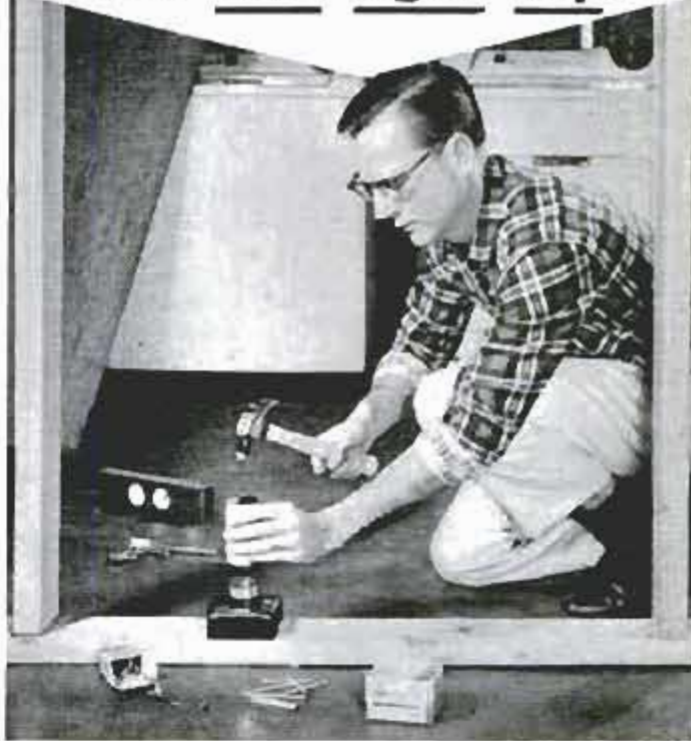
Anchoring 2x4 partition plate to basement floor.
