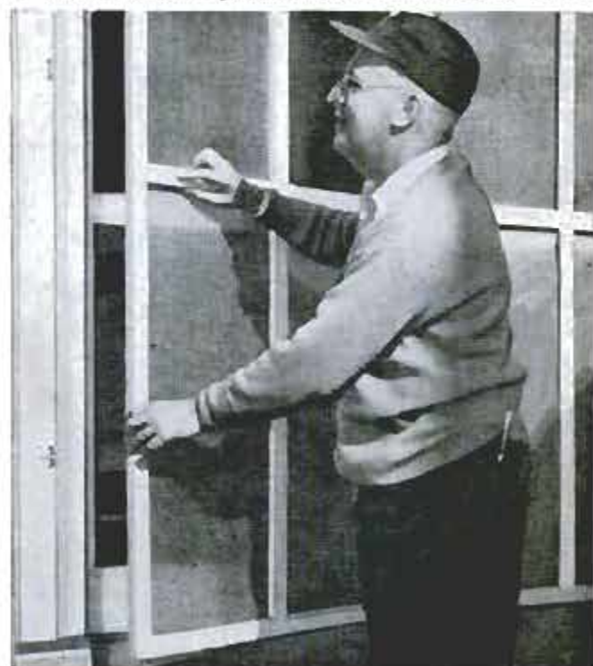
7. Below, screen-enclosed porch, and furniture stored on it, are protected from winter weather by removable "storm sash" made from 1 x 2-in. furring strips to which durable plastic-coated screening is nailed
