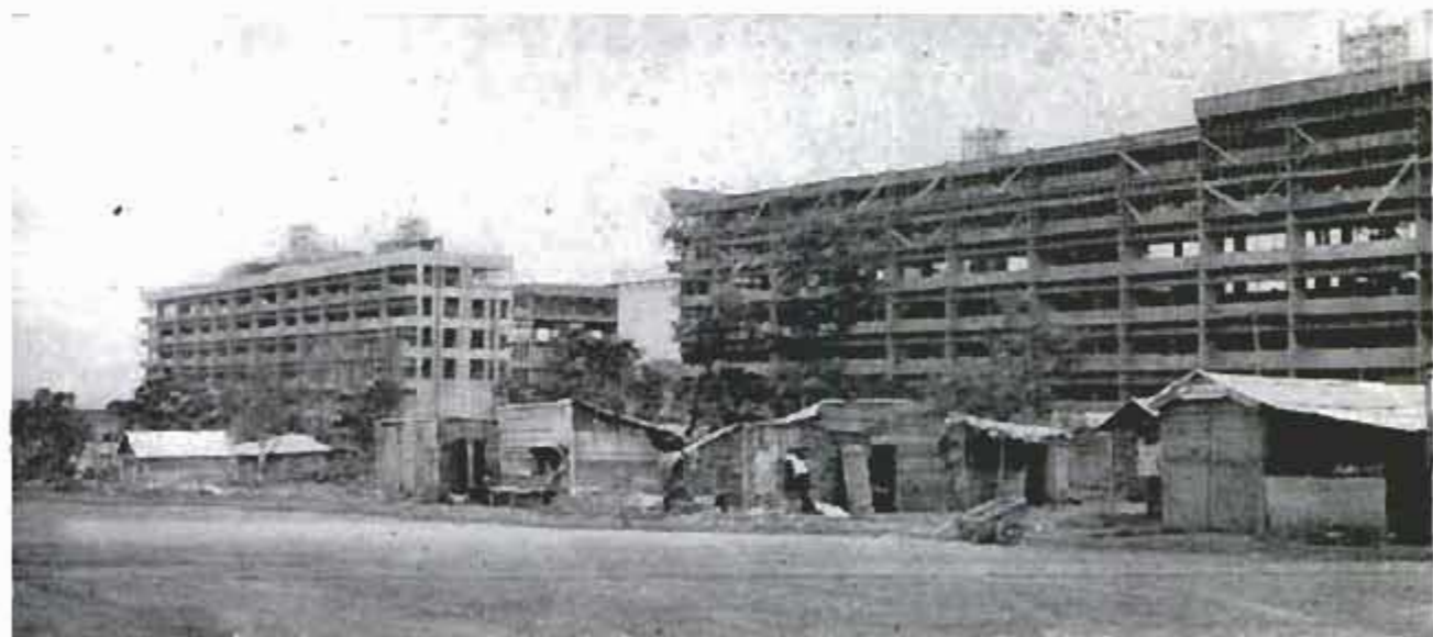
Ultramodern office buildings seem to grow overnight, and provide startling contrast with shacks of workers
