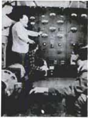
Photo of Heald Students in Electrical Laboratory
