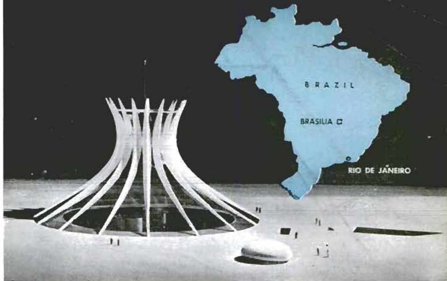
National cathedral will have boomerang-like ribs supporting glass walls. Map shows remote site of Brasilia
