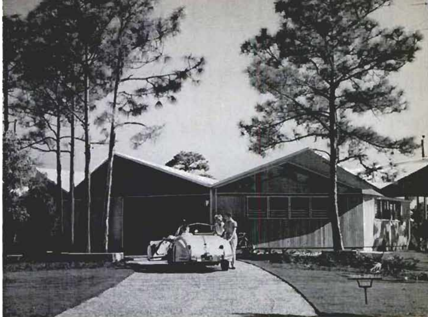
Eight-sided house in Naples, Fla., has glass gables and a driveway that goes right under the concrete roof
