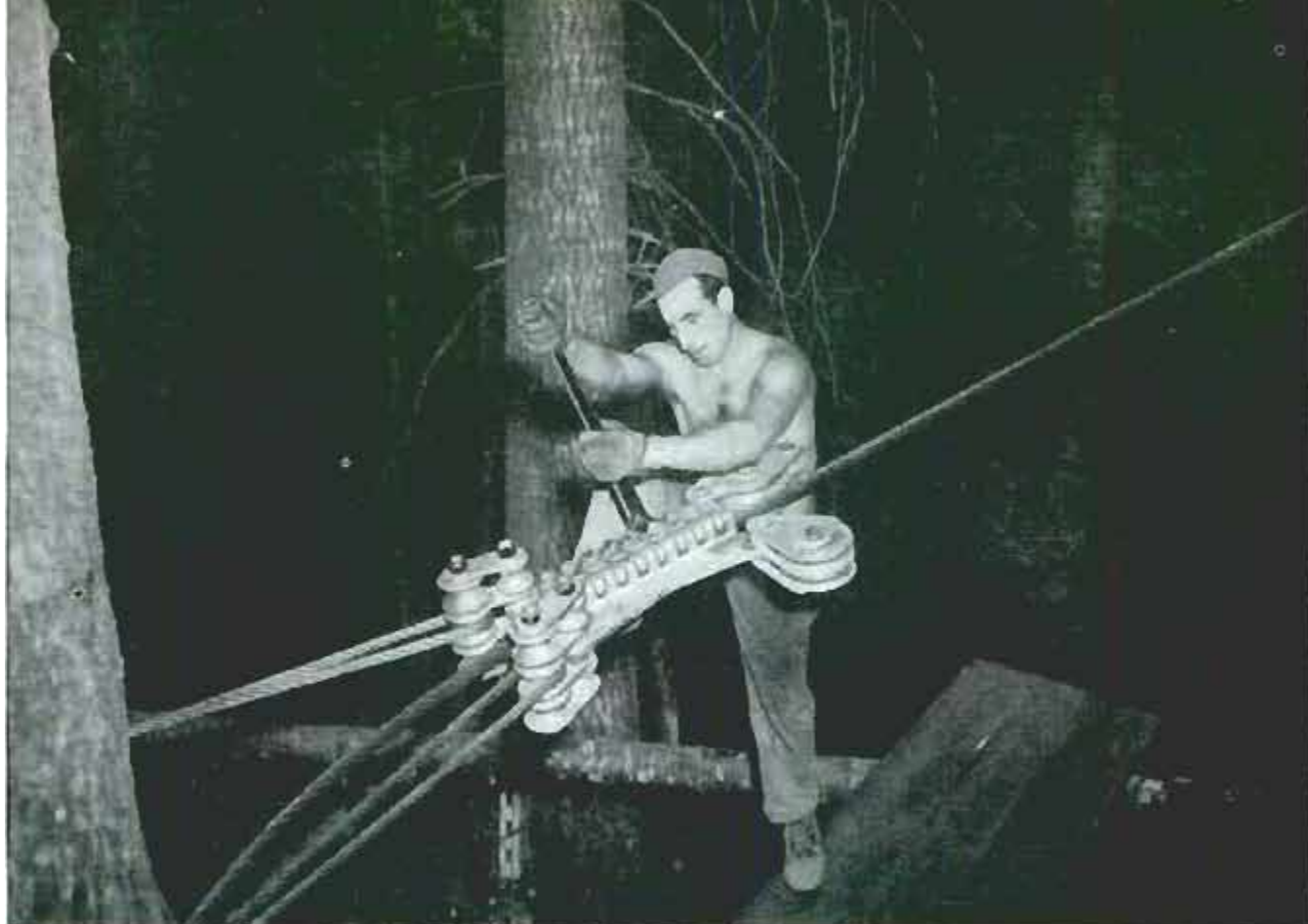
Lumberjack tightens the bolts of clamp that secures cable to anchor tree. Logs then ride the cable
