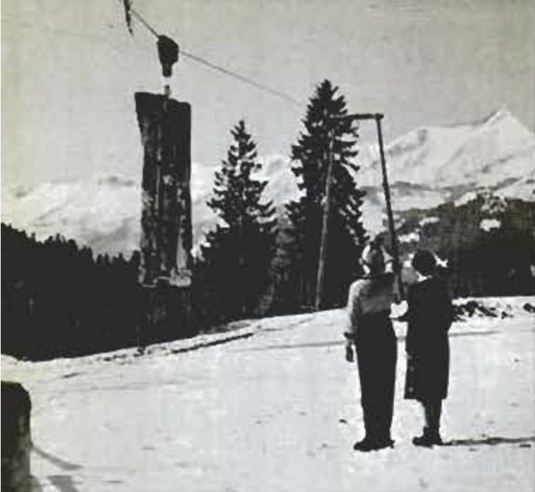
Timbers move to mill or storage on this test installation in Switzerland that traverses level ground
