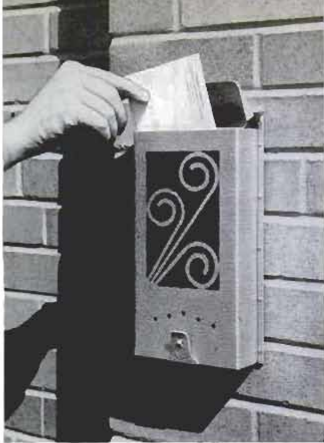
Box then is "stuck" to a brick wall without aid of masonry anchors. It will stay there for a lifetime
