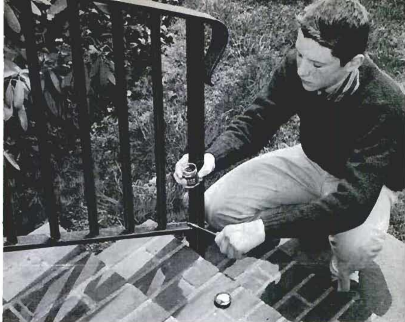
Tough grip of these new glues makes them useful for repairing, or even installing, wrought-iron balustrade
