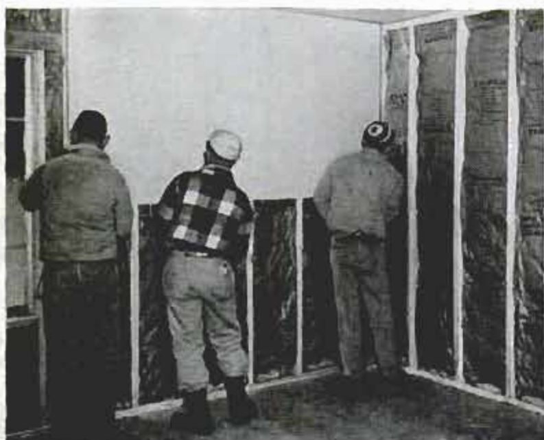
Here, sheets of rock lath are being installed on inside of external walls. The sheets are pushed tightly against the ceiling lath
