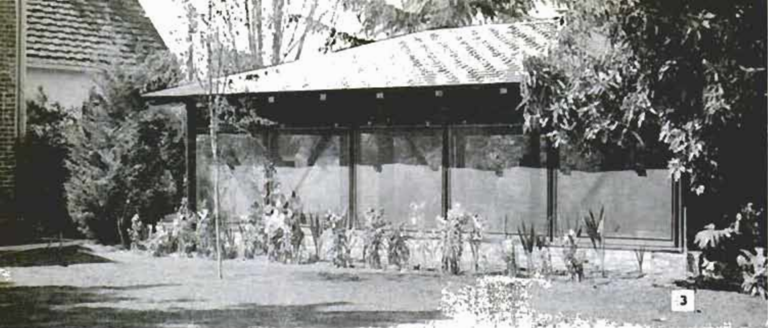
Wide aluminum screening permits use of large screen panels that can be removed, replaced with windows
