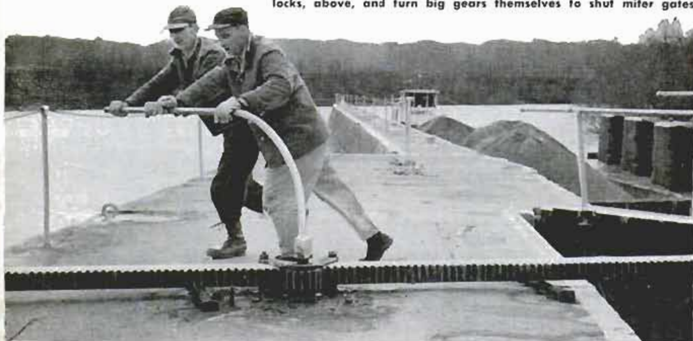
Boatmen on the Kentucky go ashore to open valves in the river locks, above, and turn big gears themselves to shut miter gates
