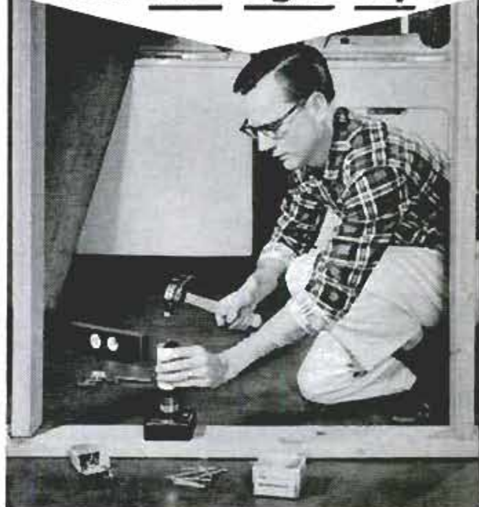
Anchoring 2x4 partition plate to basement floor.
