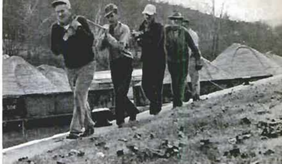
Locks won't accommodate boat plus barge, so crewmen help lockmaster haul the winch cable that pulls each barge through
