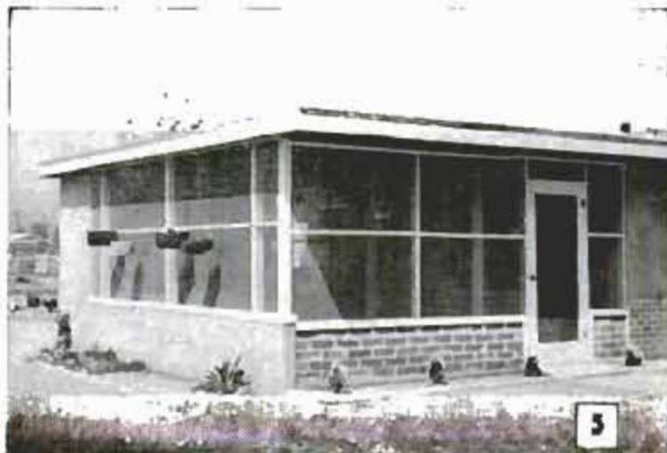
Made unnecessary by wide screening, cross members in these screened walls are for appearance only
