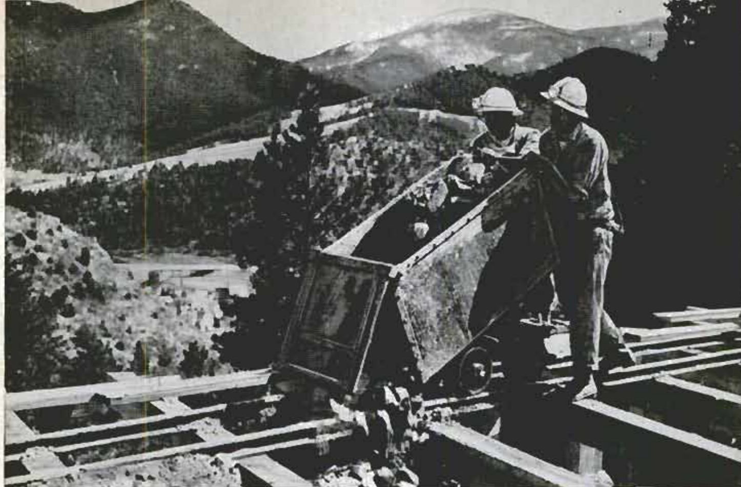
Students also learn hand-mining techniques. Here, ore shoveled by hand in mine is being dumped by hand
