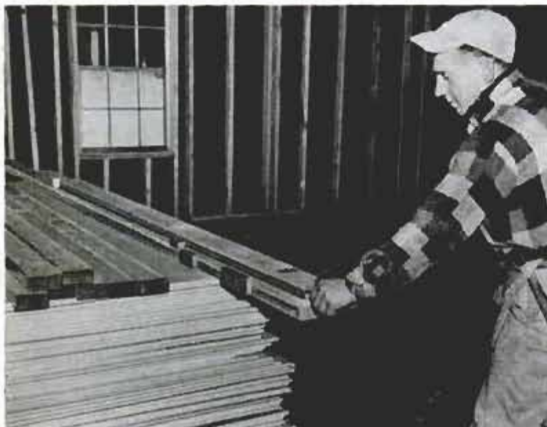
Here, sheets of rock lath are being installed on inside of external walls. The sheets are pushed tightly against the ceiling lath
