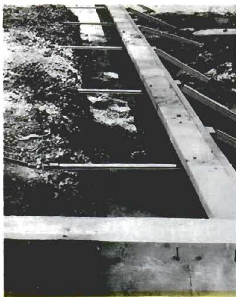
View above shows installation of pipe in gravel fill
