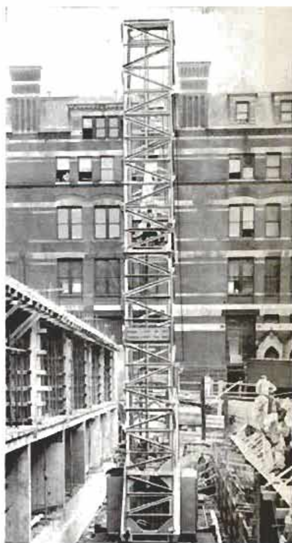
Crane rides rails in well of walls. Its "inside job" eliminates need of encircling big building with elevators
