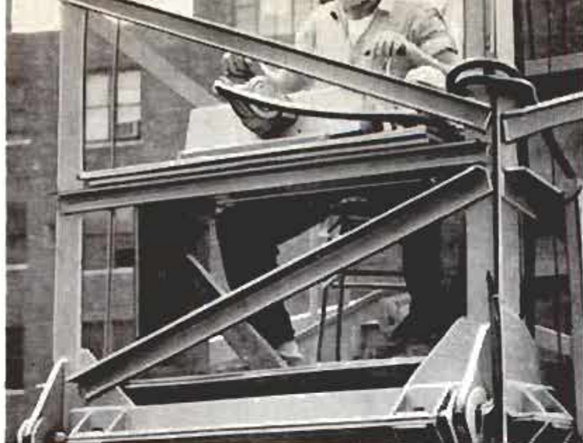
Operator can see all corners of building from movable platform
