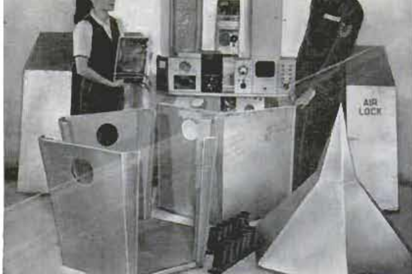
Parents built the 13 subassemblies in top secrecy. Right, punctured tin can projects "blips" on radar screen
