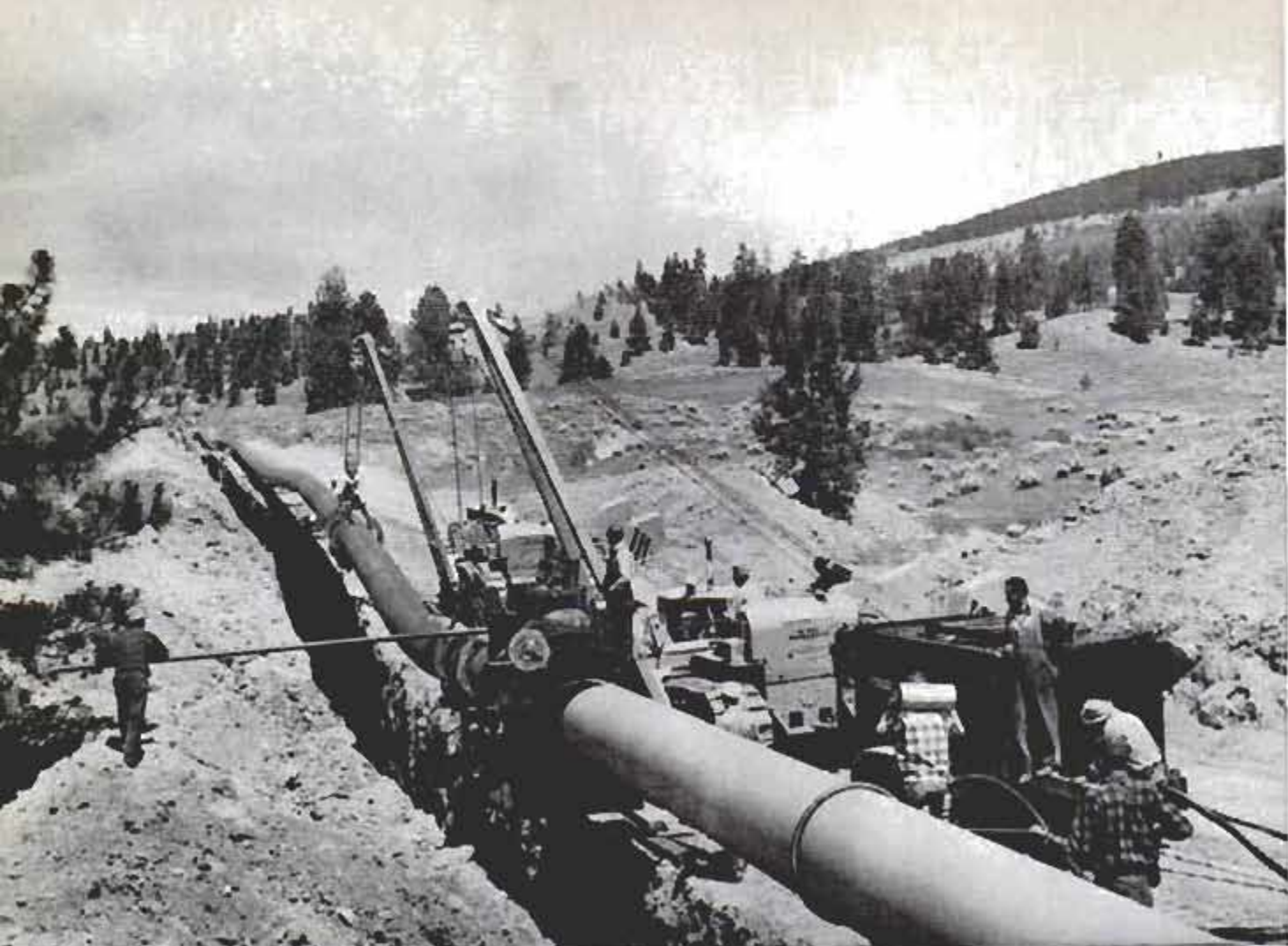
Electronic device known as holiday detector is moved along pipe to find weak spots in coating, wrapping
