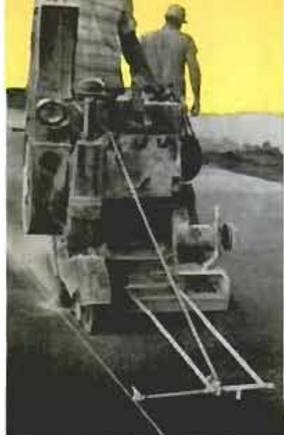
Carborundum saw cuts expansion joint in partly-cured concrete
