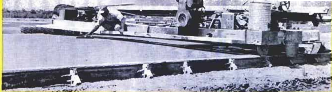
Concrete surface is smoothed by finishing machine's 12-inch rubber belt. Job formerly required two men Nonskid texture is added to paving surface by dragging a wet canvas behind the belt-finishing machine
