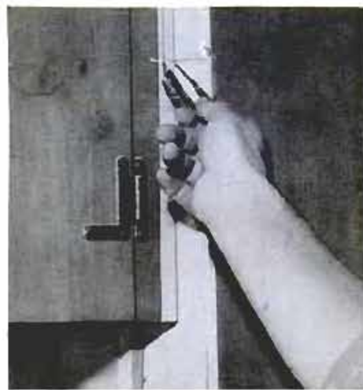
Above, cabinet is propped in position and member next to wall is taped for marking. Below, surface irregularities of wall next to cabinet are outlined on tape by compass
