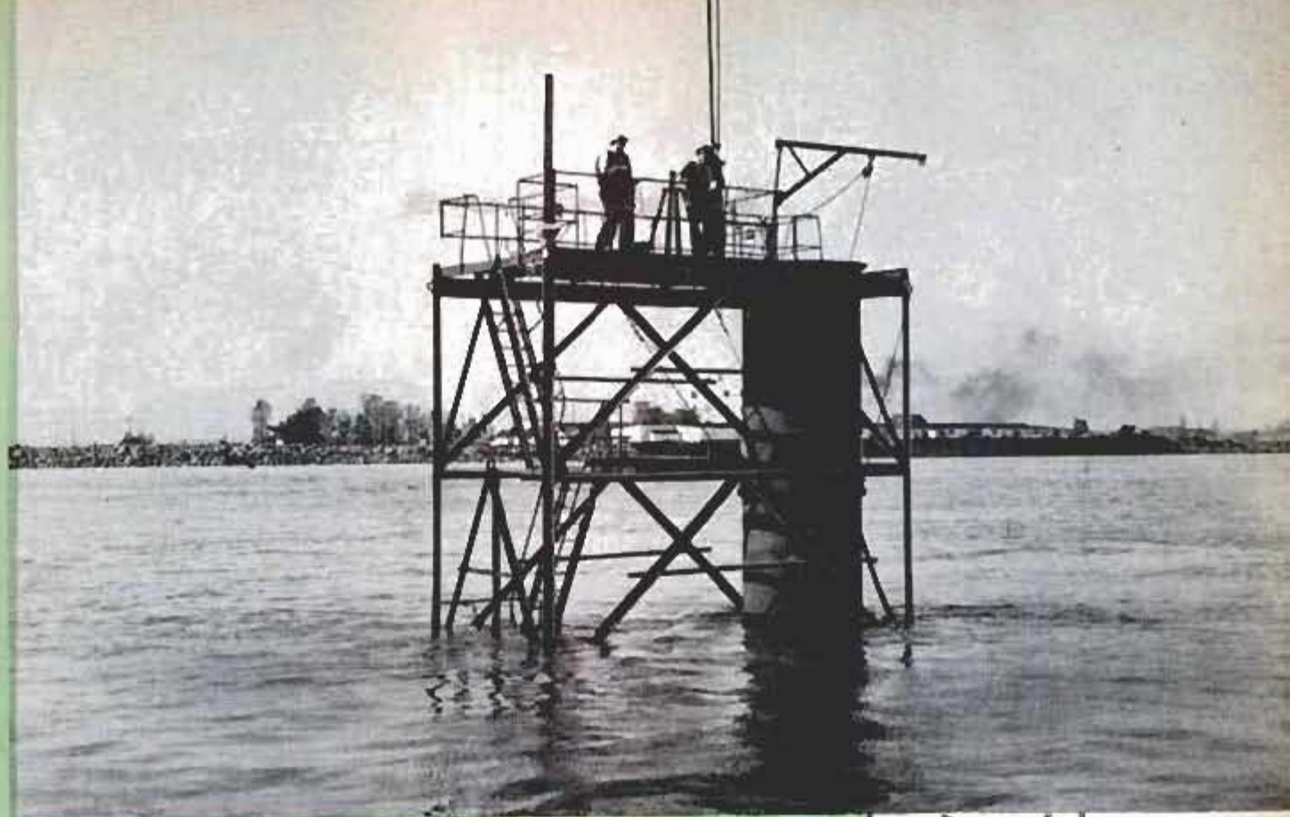
Shafts 70 feet high were fitted to the sections before sinking. Right, dotted lines show main traffic route via tunnel
