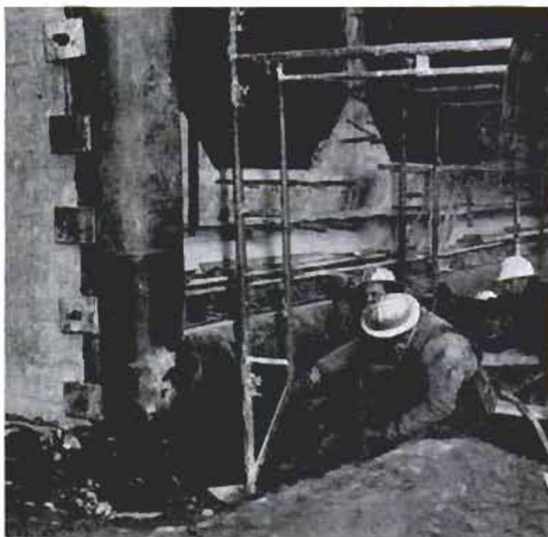
Workman inspects rubber pneumatic seal at the end of section
