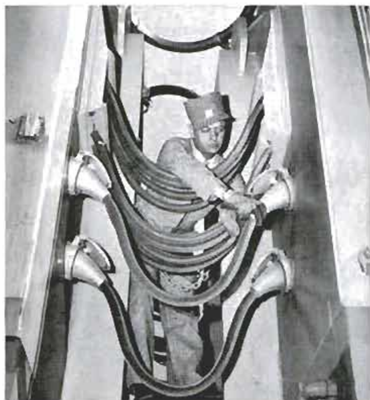
William Alberts, road foreman of engines, inspects electric cables between the turbine unit and the diesel auxiliary
