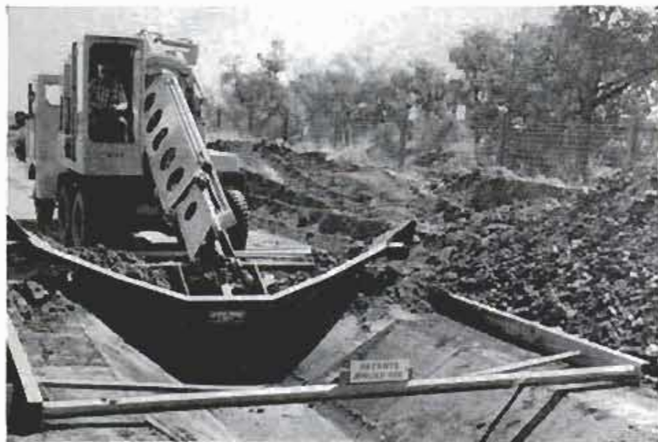
Steel sloper blade, above, is used to clean and re-shape the side walls of a canal. Dirt is carried to top of bank where lister spreads it behind tractor
