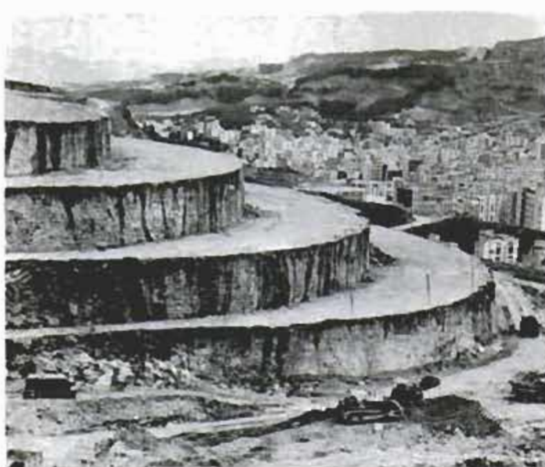
Daring in design is the Helicoid, being built in spiral around a small mountain. Shoppers will drive up "through" the building
