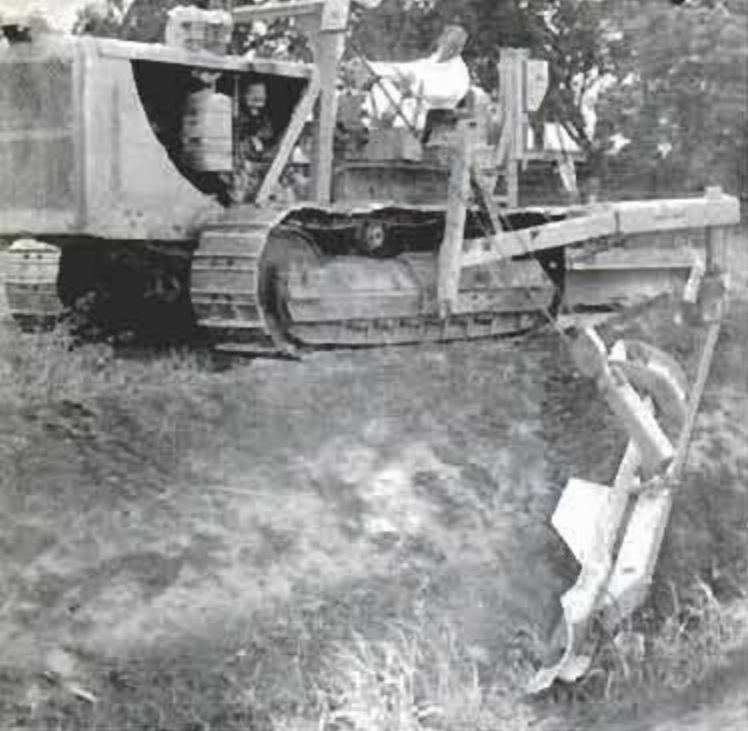
Steel sloper blade, above, is used to clean and re-shape the side walls of a canal. Dirt is carried to top of bank where lister spreads it behind tractor
