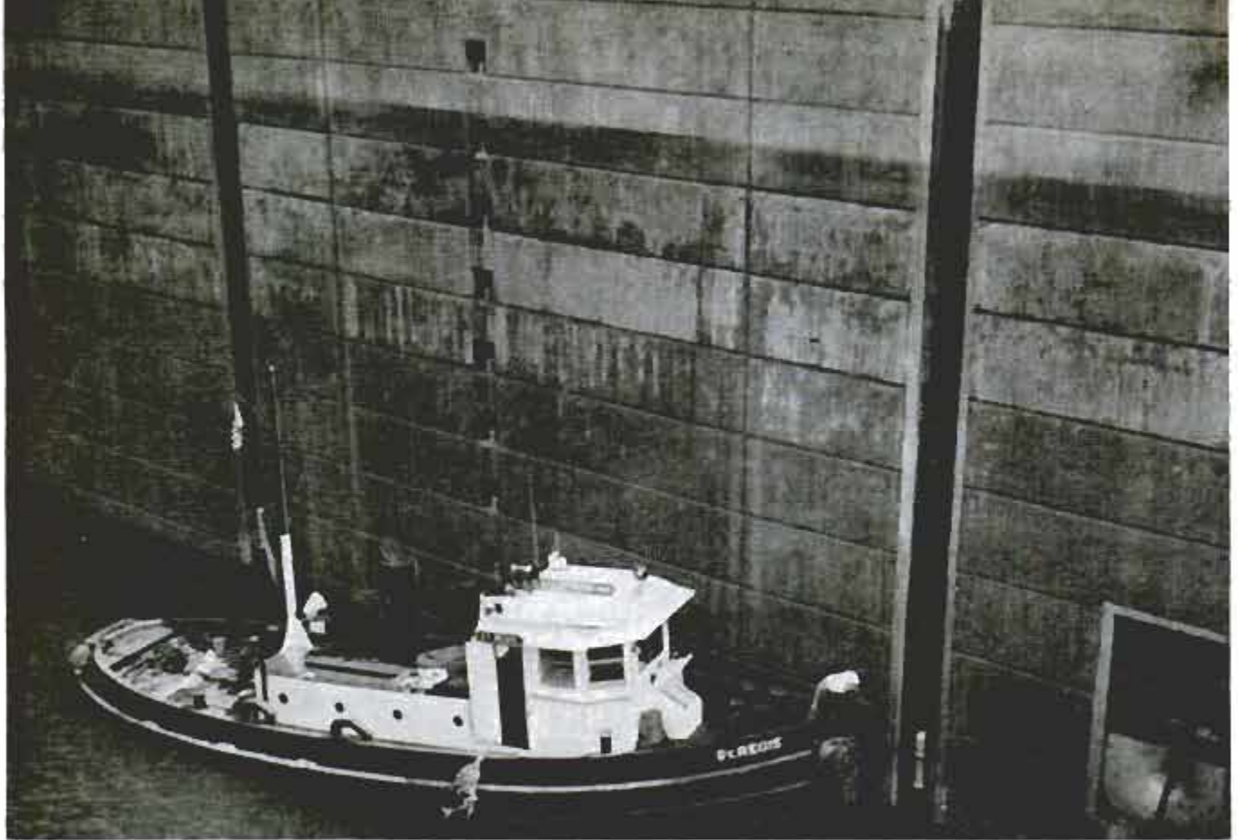
Innovation in the locks are mooring posts that slide up and down in slots in wall as water level changes
