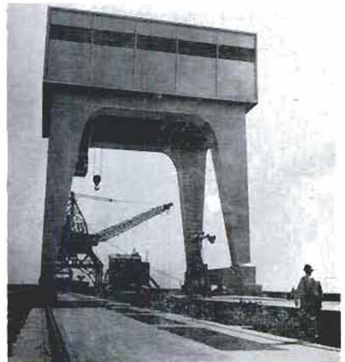
Riding the top of power dam like giant four-legged stool is gantry crane that lifts and lowers gates
