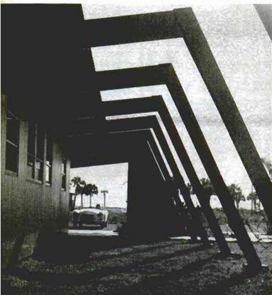
Outriggers shown at the back—or is it the front?—of the house are made of two by eights and support entire weight of the roof. Exterior walls here are to kitchen and dining area
