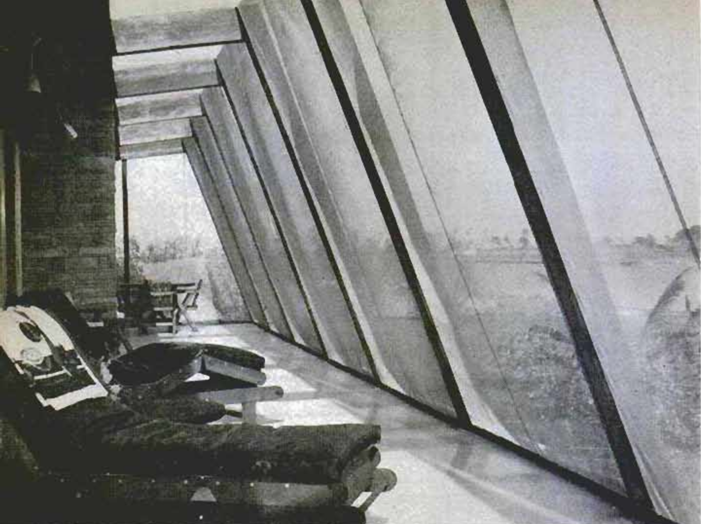
Screened outriggers across length of house provide an outdoor-living area 11 feet wide and 64 feet long
