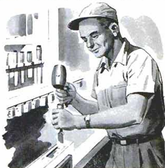
SAW CHEEK CUTS IN WASTE
