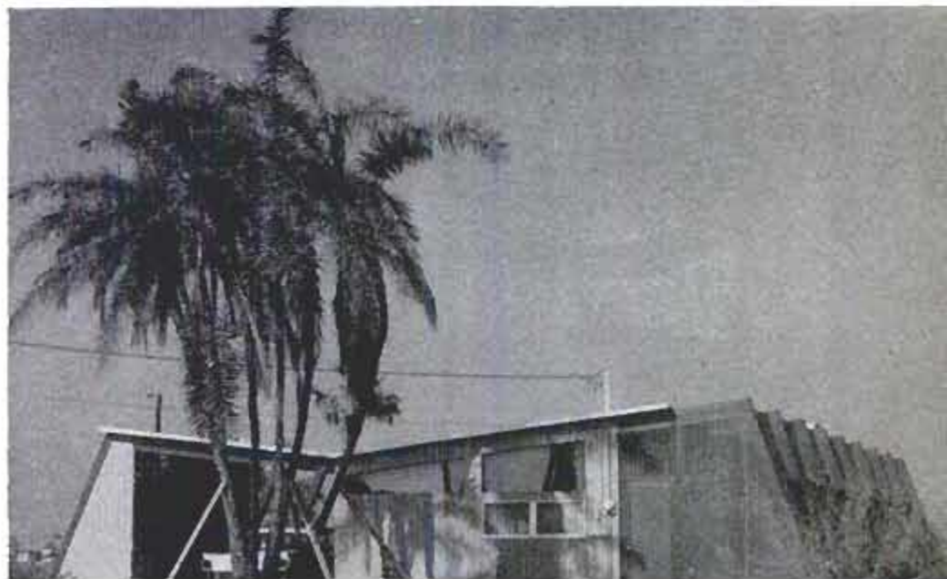
Outriggers are enclosed beside carport to form utility room. This view also shows windows of bath and multiuse area, plus big porch
