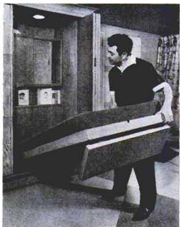
Owner demonstrates built-in guest room with fold-up bed and storage area in back
