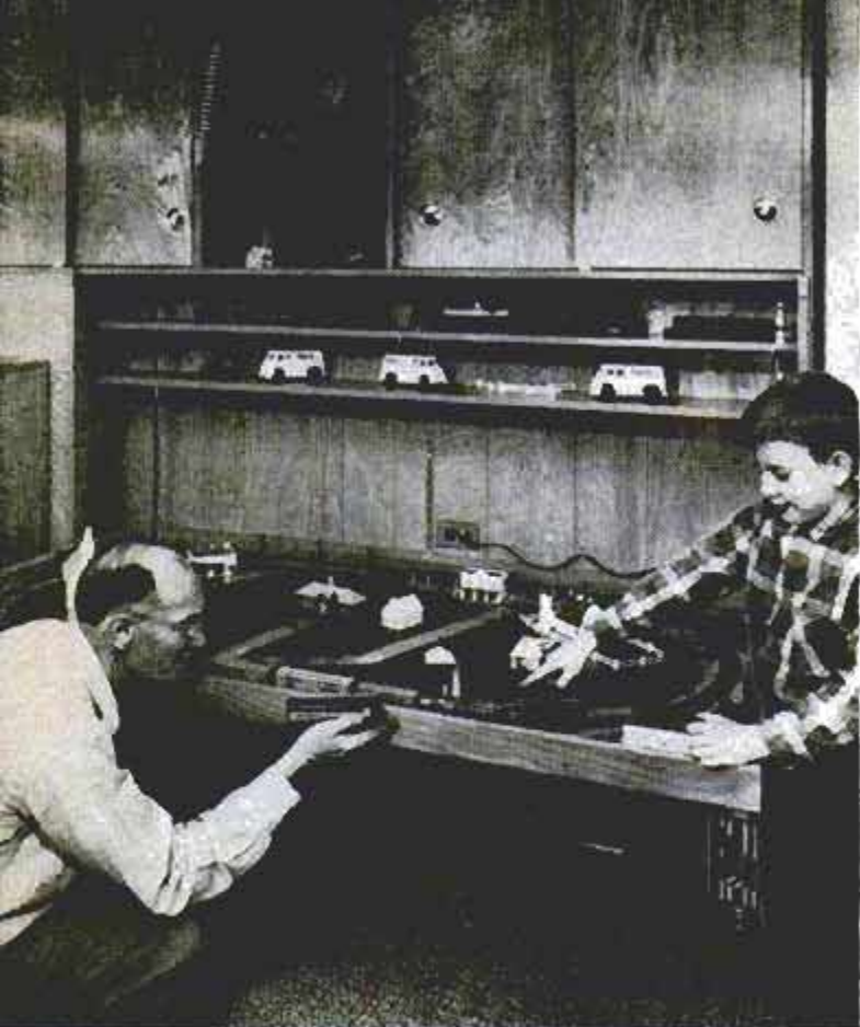
In the boys' room, tracks for toy train are mounted on board which folds into wall, becoming chalkboard
