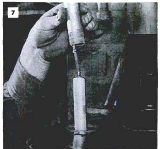
Figs. 5 and 6, when there is limited clearance above hot-water tank, flexible magnesium anode is used
