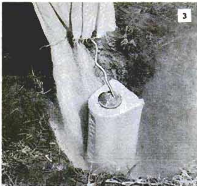
2 Above, lead wire from magnesium anode is soldered to cleaned surface on sprinkler pipe. Figs. 3 and 4, after backfill is poured around anode, it is saturated with water and completely covered with soil
