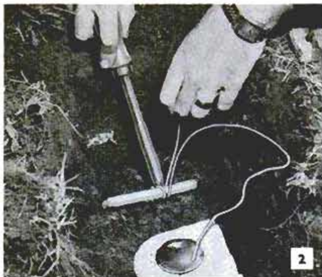
2 Above, lead wire from magnesium anode is soldered to cleaned surface on sprinkler pipe. Figs. 3 and 4, after backfill is poured around anode, it is saturated with water and completely covered with soil
