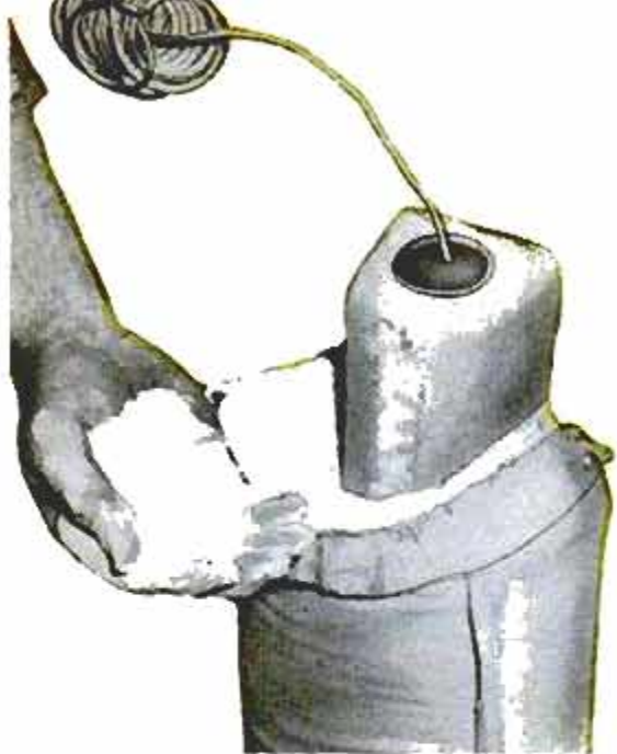
1 Above, magnesium anode is packed in quick-wetting backfill that is buried with anode to retain ground moisture, assuring constant flow of electrical current
