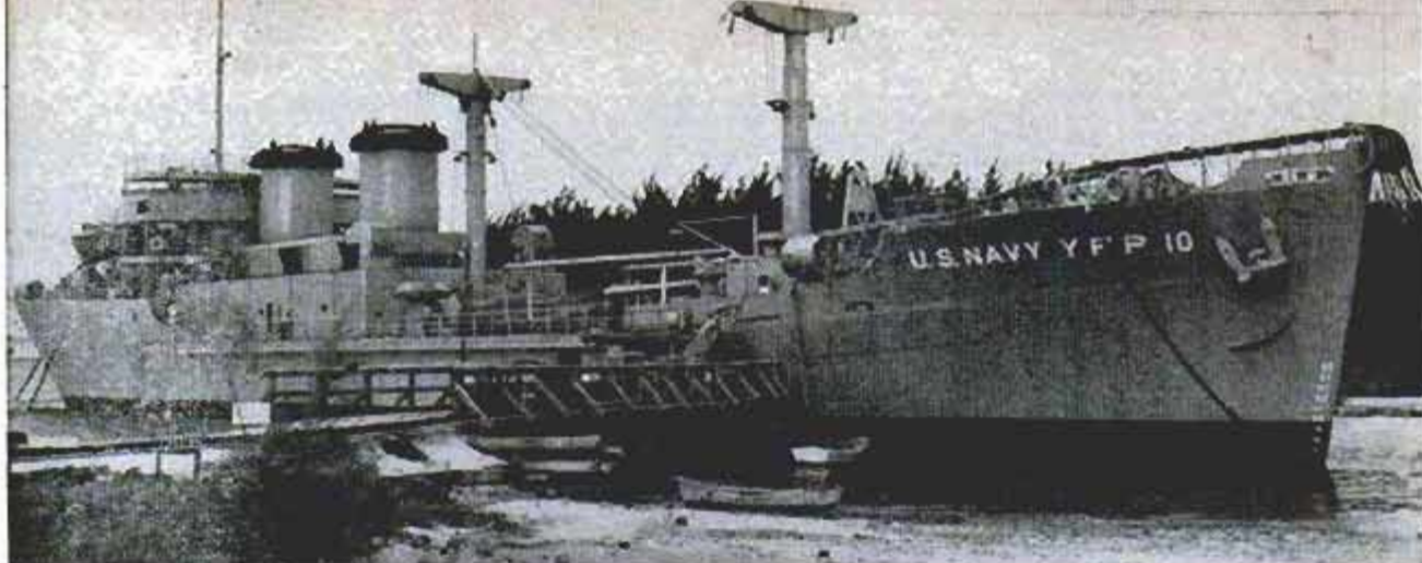
The YFP-10, a floating power plant, is moored with seven anchor chains to I-beams sunk in coral rock
