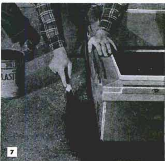
Above, roofing cement is spread around frame of skylight to seal joint between frame and roof. Below, strips of roofing felt are pressed into cement. This is repeated until several layers have been applied
