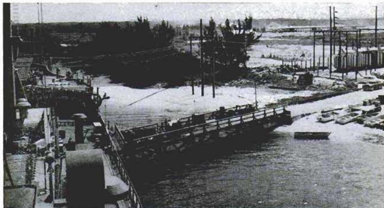
A substation, right, was built so the YFP-10's current could be converted for land-line transmission
