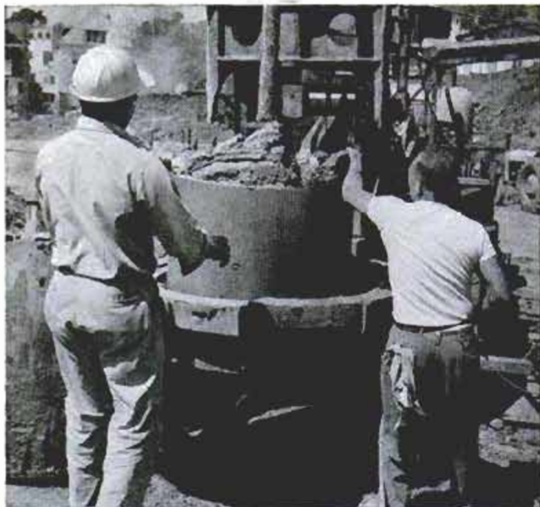
The boring bucket brings 300 pounds of earth to surface. Cutters on the bucket's side slice the earth and force it inside
