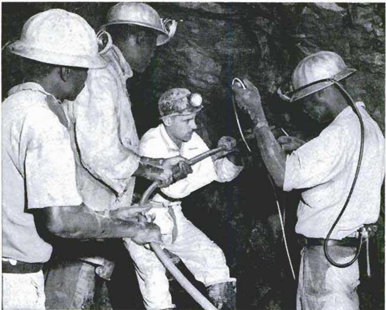
Workers use 115,000 miles of safety fuse annually in driving shafts and tunnels through gold-bearing rock
