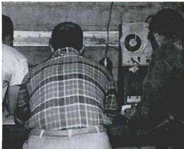
Inside the blockhouse, crewmen watch the rocket launching through slit windows. Rockets are triggered from this building. Recorder, used for research, picks up sounds of launching
