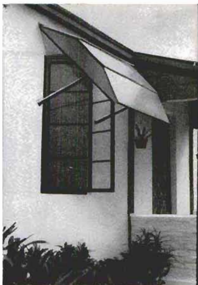
Above is shown the storm-shutter awning in the "up" position. The supporting braces for the awning part of the assembly are pivoted on the storm flap that swings up inside when the unit is held in this position
