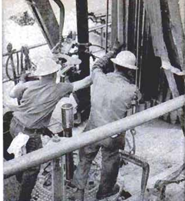
Drillers putting down well at Paradox Basin location add another length of drill pipe to the "string"
