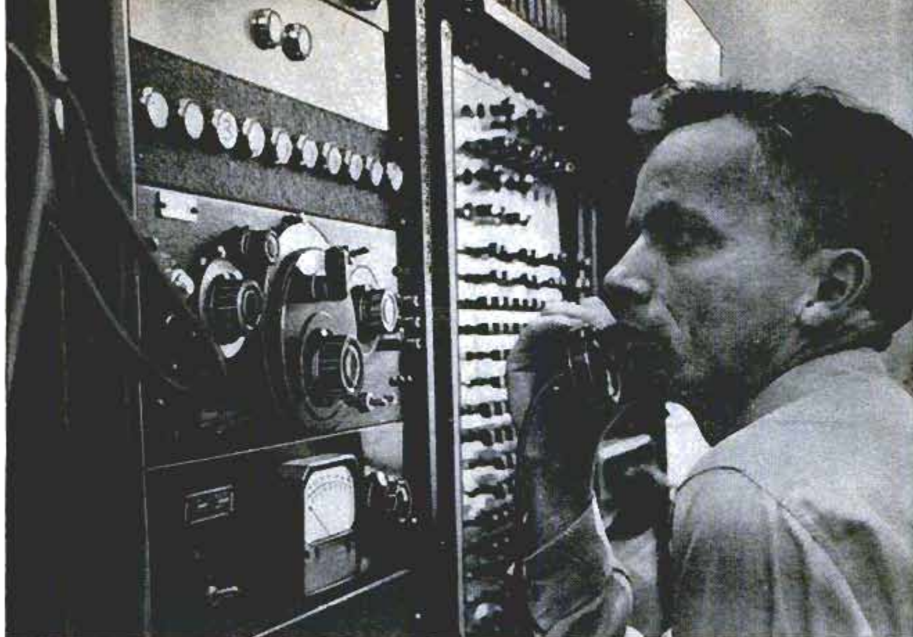
Bell engineer demonstrates "Audrey"—electronic device that reacts "intelligently" to 10 spoken numbers
