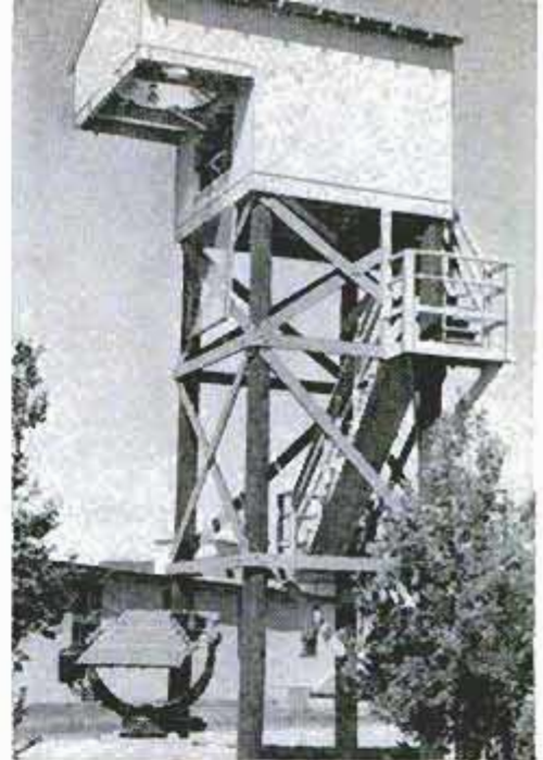
In tower furnace, sunlight reflects from flat mirror up to paraboloid, then to 6000-degree focal working spot
