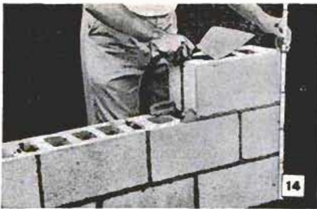
Rule, instead of course pole, can be used to assure that block courses are maintaining proper 8-in. height
