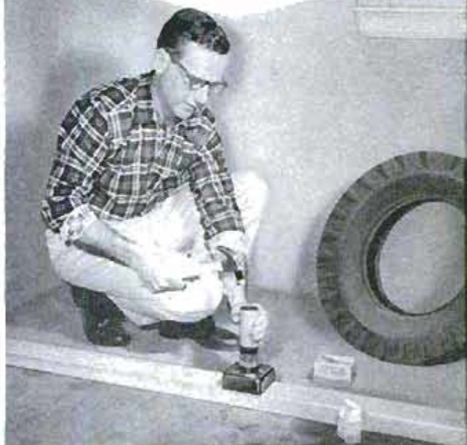
Anchoring 2 x 4 car stop to garage floor.
