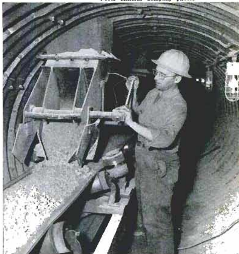
Workman adjusts feed chute which carries crushed ore to an industrial plant for lithium extraction Foote Mineral Company photos
