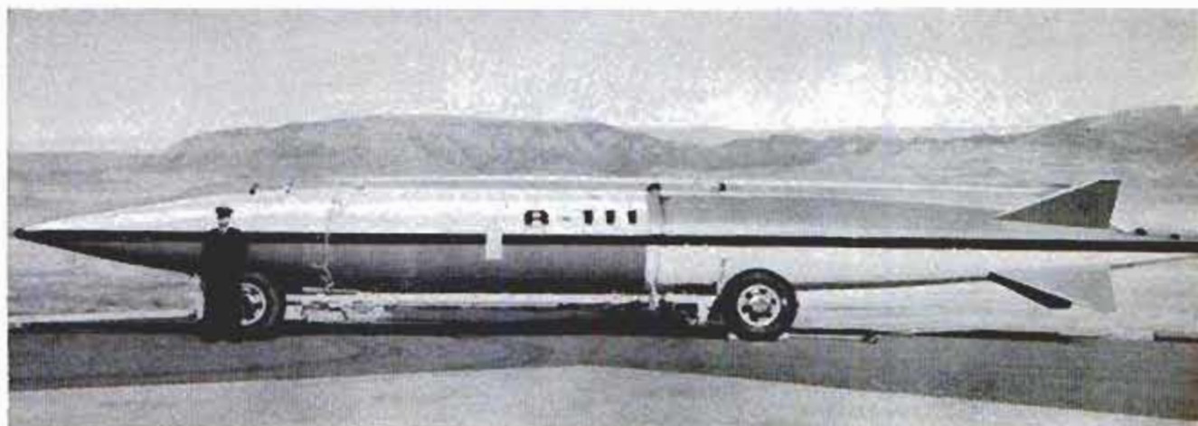
Airman appears small beside detachable pod carried by B-58. Pod gives plane nuclear-bomb capability
