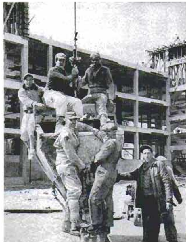
Here are some of the men who rode concrete bucket to safety from 13th floor after flames trapped them
