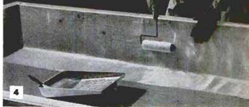
Above, resin-saturated paint roller is used for removing bubbles and wrinkles from glass-fiber cloth, starting each stroke at top and working downward
