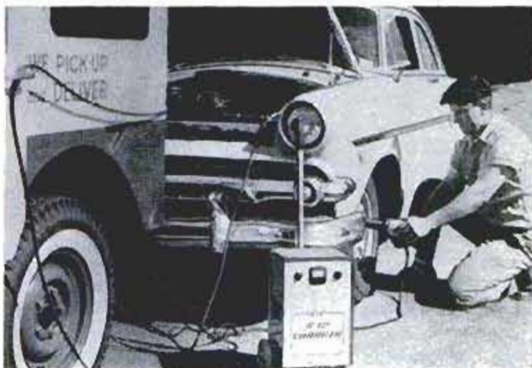
Combination a.c.-d.c. generator can be connected piggyback fashion to original equipment unit for extra power, above. Power tools, below, also can be operated by combination unit
