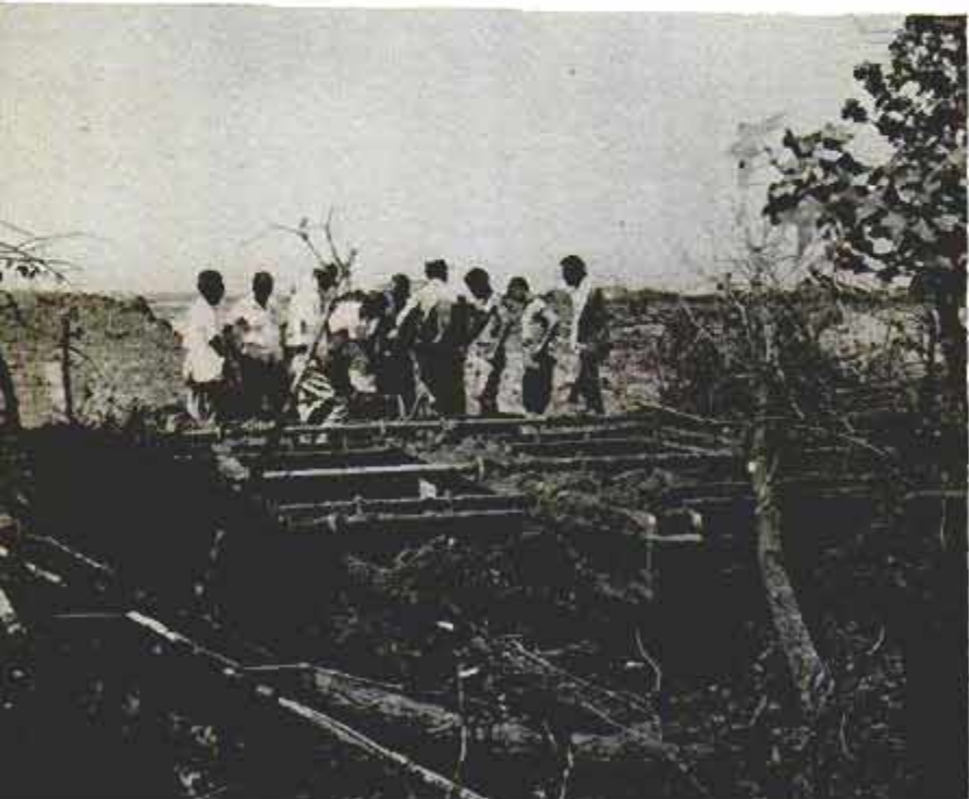
If arresting gear fails, 30 tons of steel dead load hurtles off runway. This one landed in mud on other side of lake
