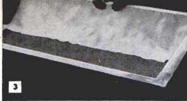
Next, end and side pieces of glass-fiber cloth are applied one at a time as shown above. Each piece is cut and checked for proper fit before applying resin
