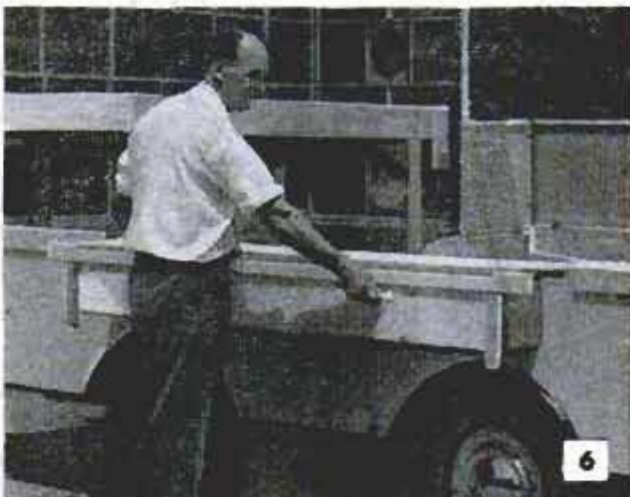
Drawer pulls attached to pull-out bunks permit handling them like bureau drawers. Hinged side walls of bunks then are raised and tubing brackets installed
