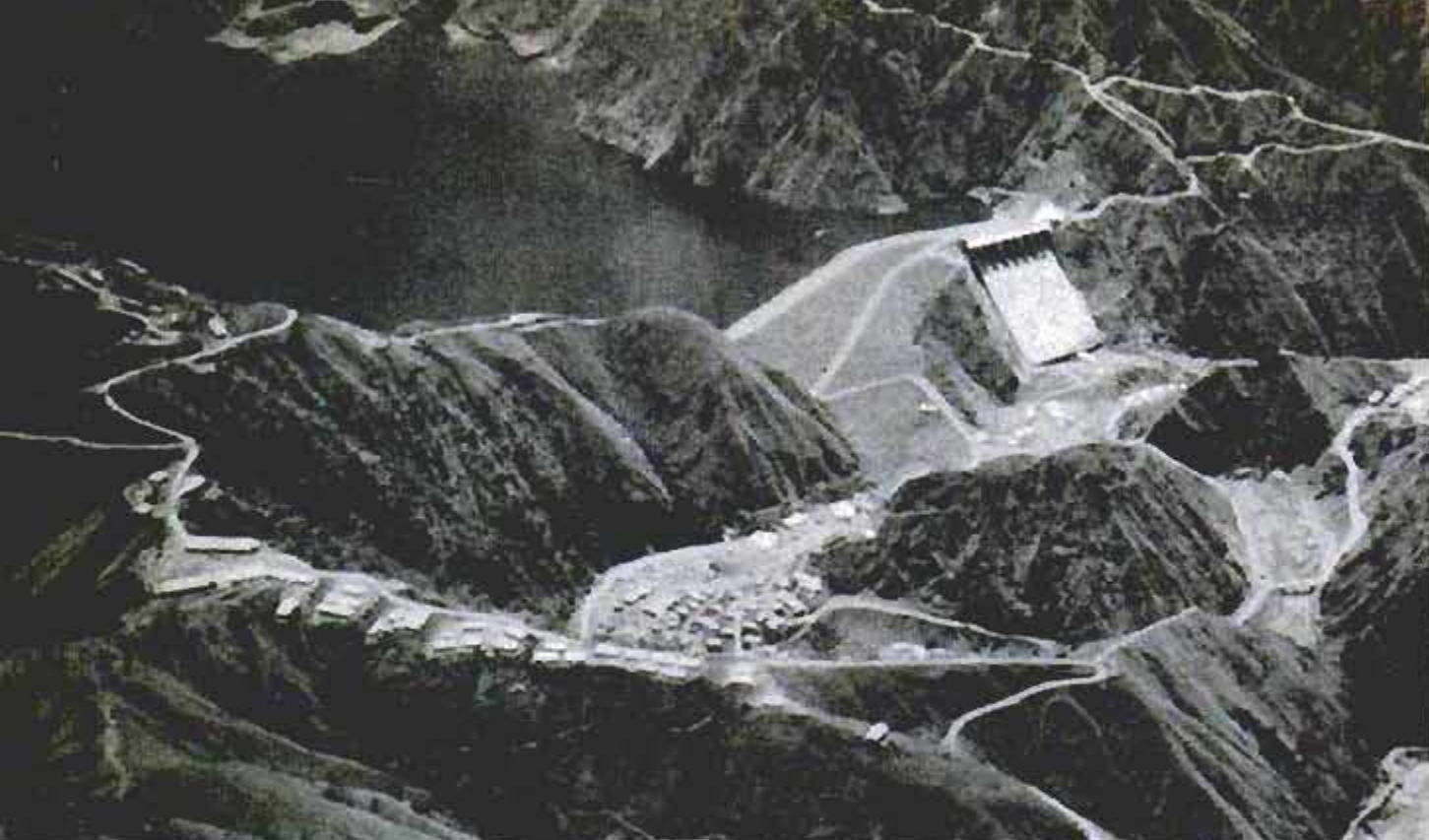
Ambuklao, biggest rock-fill dam in the world, was completed last year as first of six in northern Luzon
