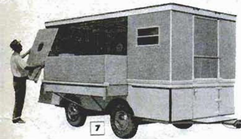
In this photo one side wall has been left off to demonstrate headroom inside trailer for 6-ft. man, and to show how bunk beds are set up on brackets
