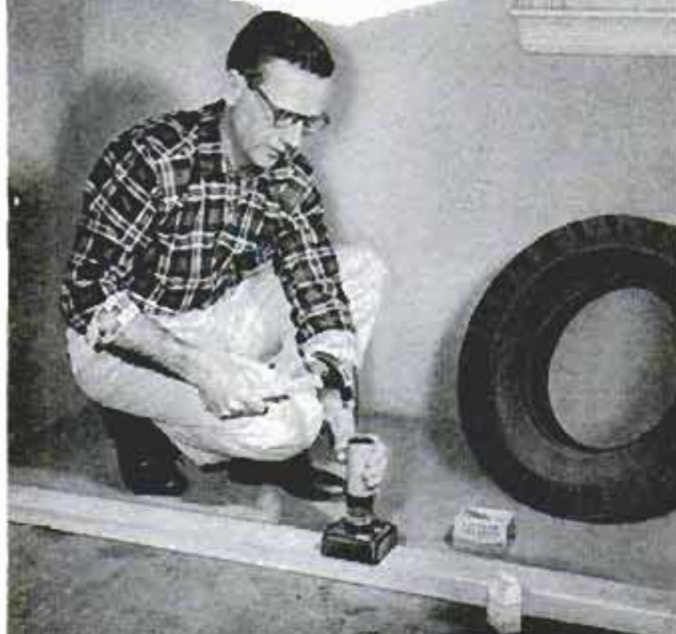
Anchoring 2 x 4 car stop to garage floor.
