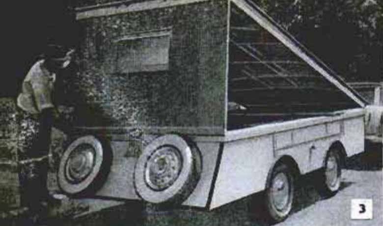
First step in setting up trailer is to raise one end of roof and swing down one end wall that is hinged to roof. Lower end of wall is screwed to trailer body
