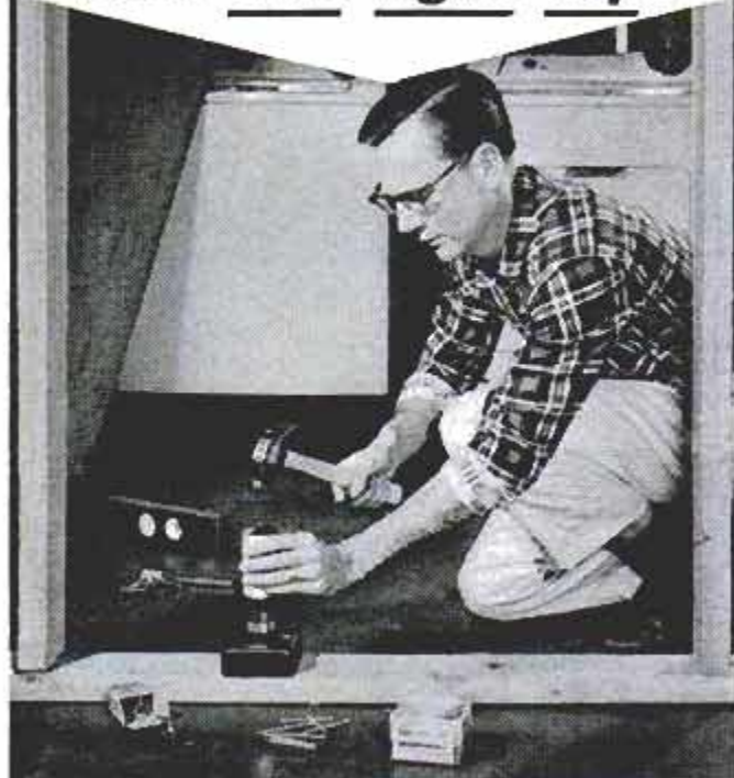
Anchoring 2 x 4 partition plate to basement floor.
