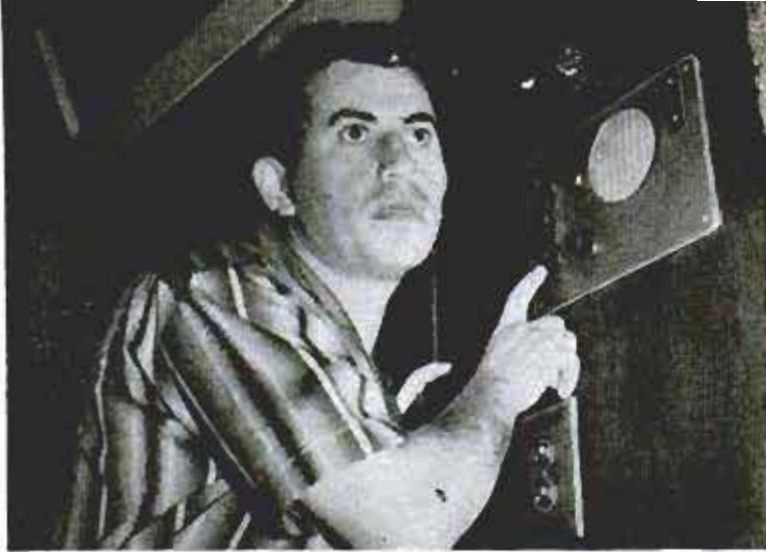
Intercom system linking house with movie-viewing room lets Basches monitor children's room while watching film. It also lets family know when movie is about to start. Car-type speaker, below, has been replaced with an 18-inch hi-fi speaker
