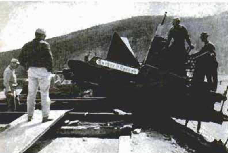
Dam's steep slope and narrow top created problems. There was not enough room for machinery to turn around. Below, the lay-down machine is pulled on turntable and moved along dam to lay next strip
