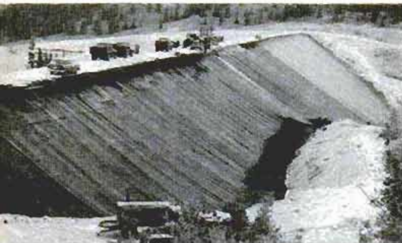
Dam's steep slope and narrow top created problems. There was not enough room for machinery to turn around. Below, the lay-down machine is pulled on turntable and moved along dam to lay next strip
