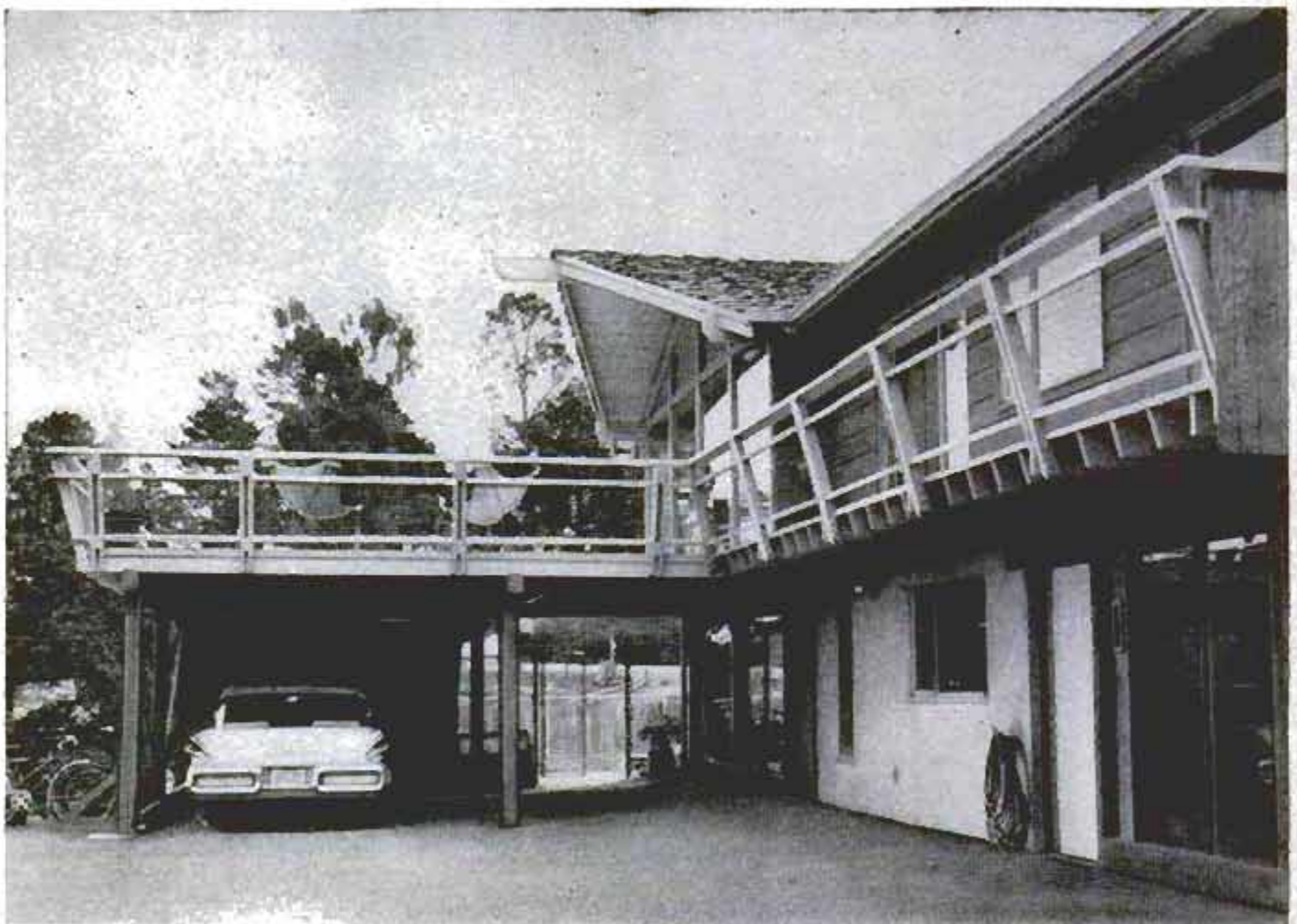
Roof-top patio of Jack Lind home has area of 24 by 27 feet plus deck walk. The floor is one-inch-thick concrete poured on \frac{3}{8} -inch exterior-grade plywood. Ground-level view, below, shows carport beneath patio
