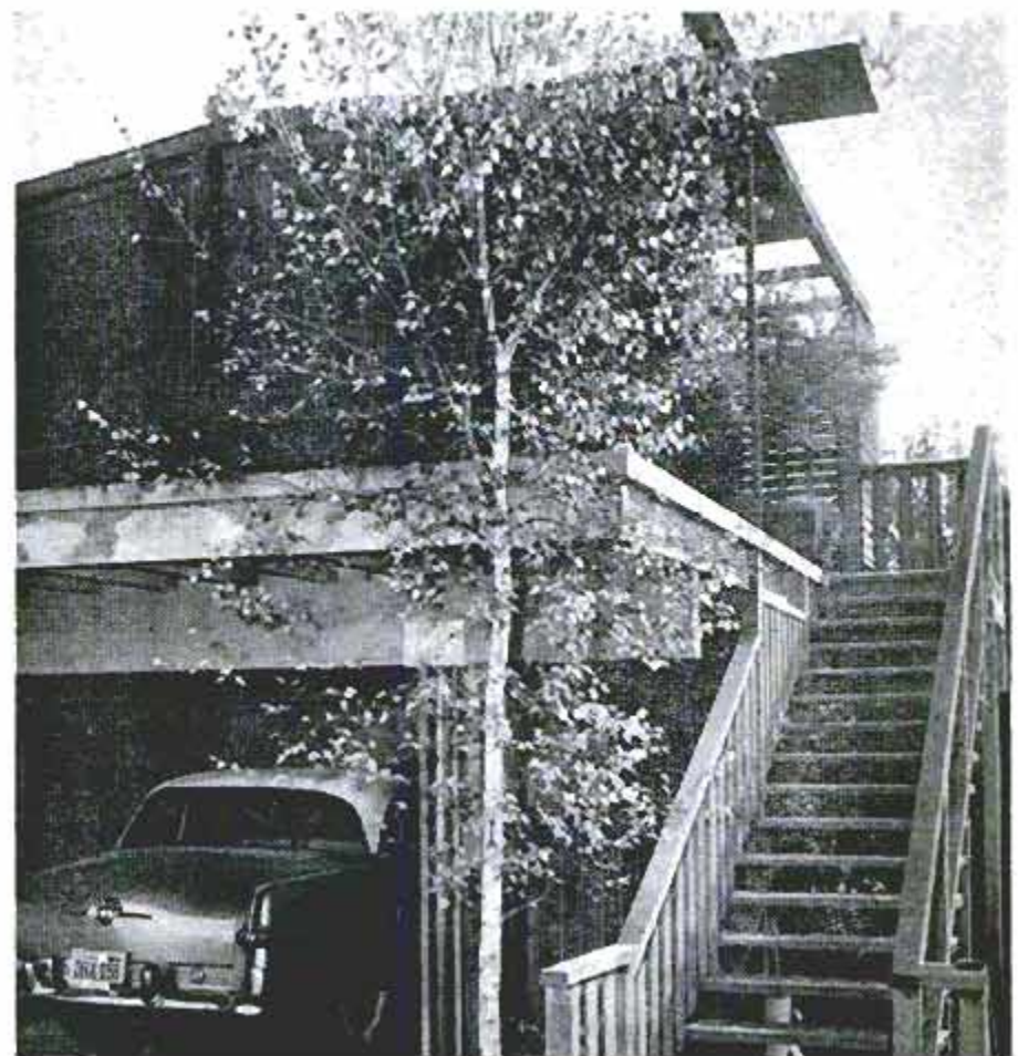
Outdoor-living area on roof of Hugh Henes carport is 12 feet above ground but gets garden look from vines on fence and tubs of flowers and shrubs. Patio floor is concrete panels with two-inch redwood dividing strips. Sunlight and shade are controlled by overhead canvas panels
