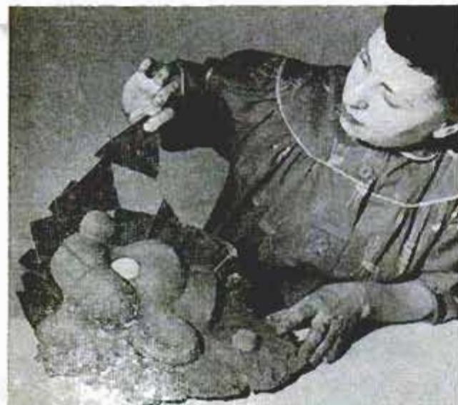
Sheet-metal shims pressed in clay at center of face serve as parting line for plaster-of-paris castings
