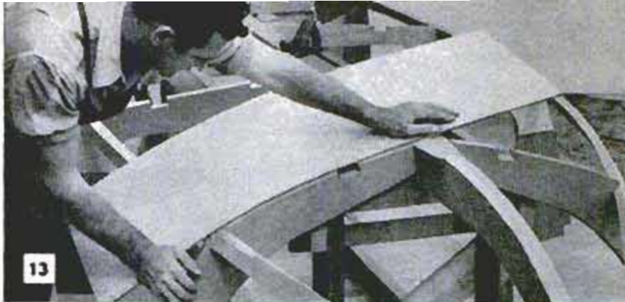
Fig. 13, thin plywood strip is pressed against each member in curved sections of hull framing that is to receive planking to check on fairing of these members
