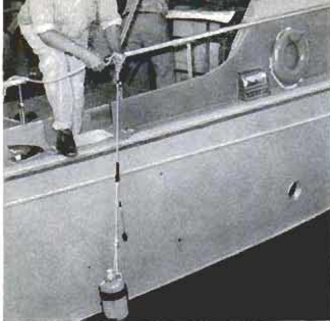
Plastic bottle goes over the side to collect water specimen for analysis in battle against the red tide
