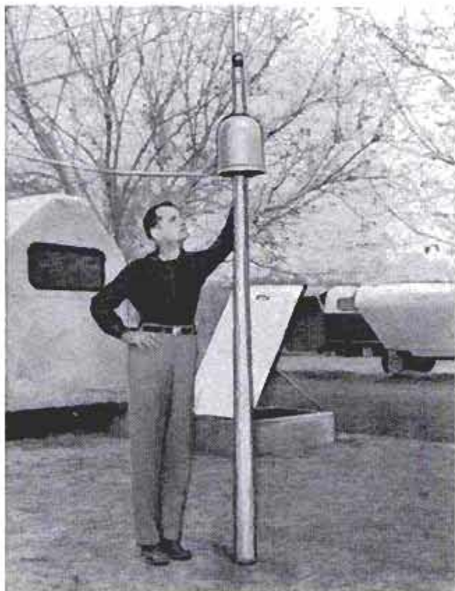
Transmission antenna for radio transmitter extends through roof of shelter. Hatch is in the background
