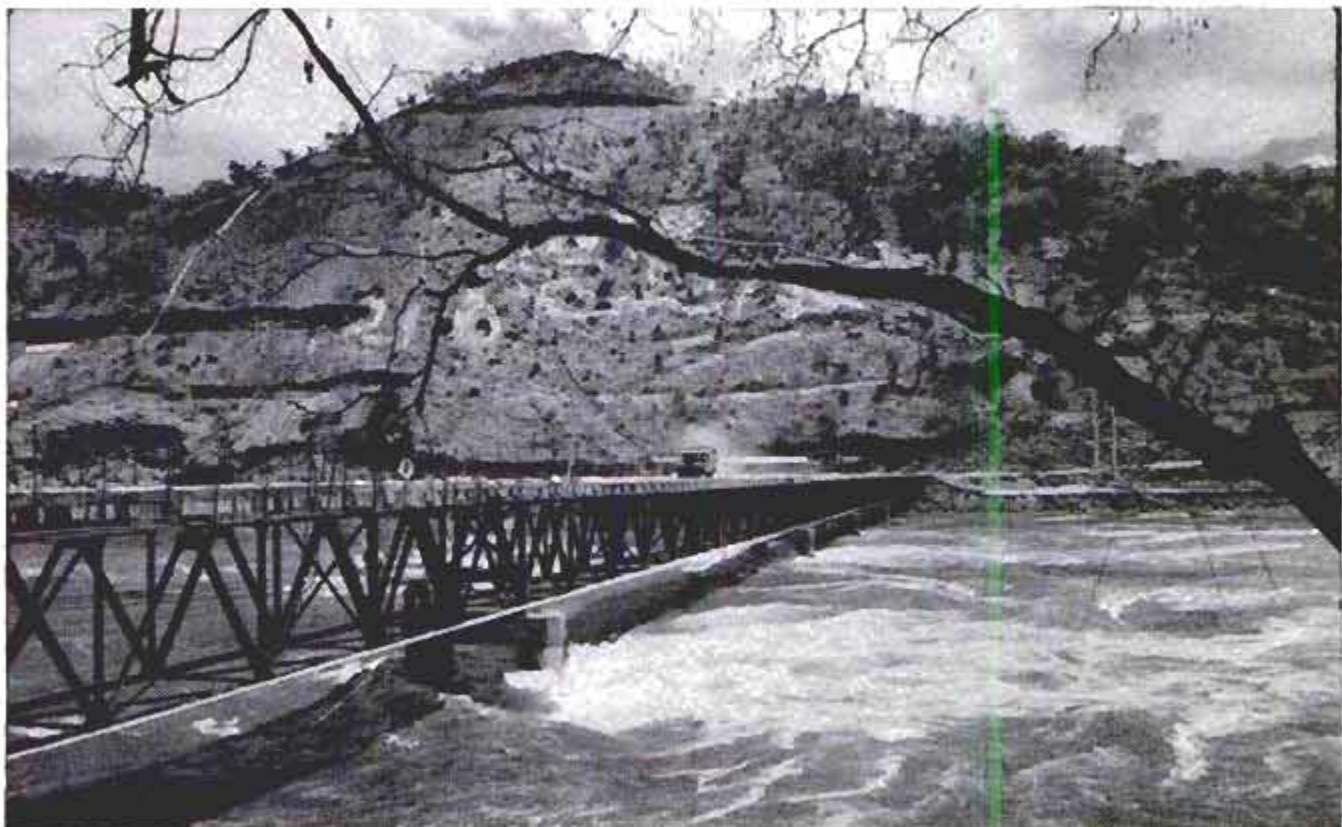
Boiling waters of Zambesi lap at Kariba Dam bridge supports during 1957 flood that submerged cofferdam
