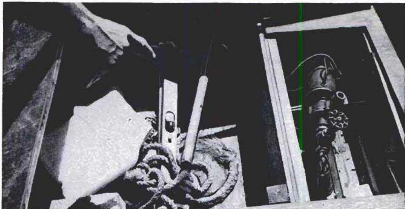
Fig. 8, above. Enclosed space below deck with clutter of damp gear is likely place to find dry rot
