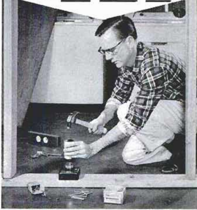
Anchoring 2x4 partition plate to basement floor.
