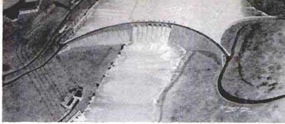
Kariba Dam as it will appear when completed. Water from Zambesi will be diverted into turbines through intakes and tailraces, indicated by dotted lines. Road crosses top of dam
