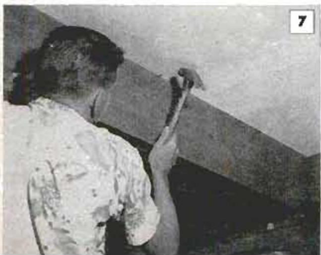
Three sides of box that form simulated beam now are nailed around duct. Lower corners of box are mitered so assembled box will appear as solid wooden beam
