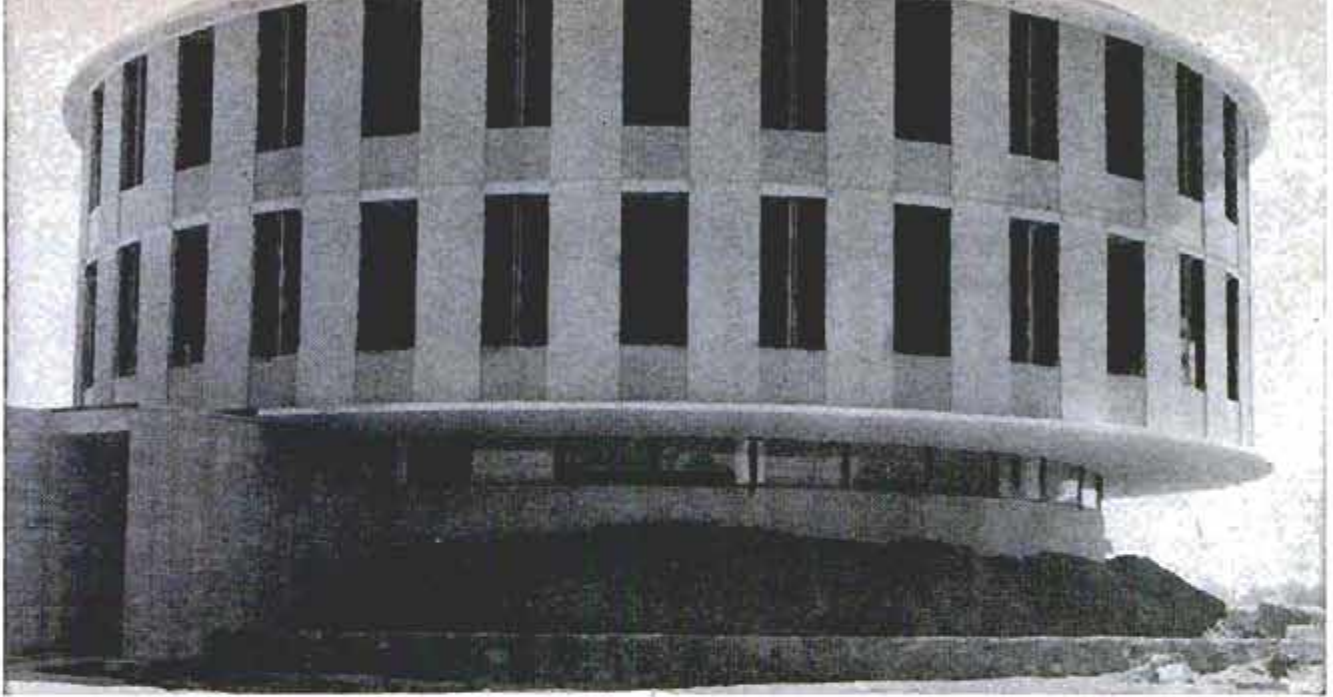
All patients have outside rooms in 66-bed circular unit. Nurses' area and utility rooms are in the center
