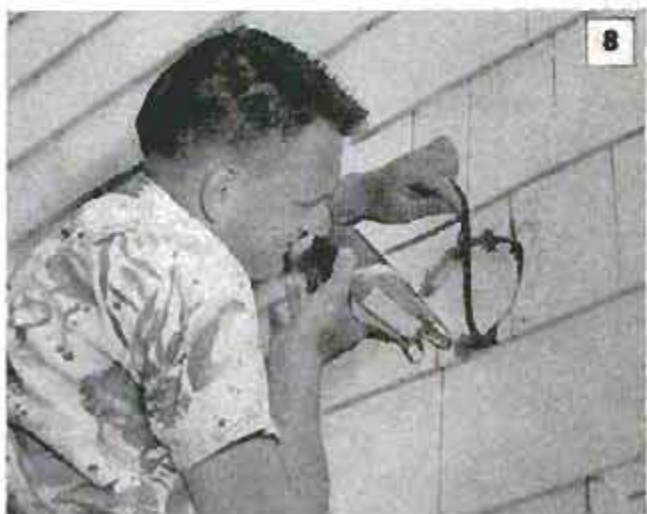
Before horizontal run of ducting is installed, hole is cut through outside wall. End of duct then is protected by weatherproof louver or other device
