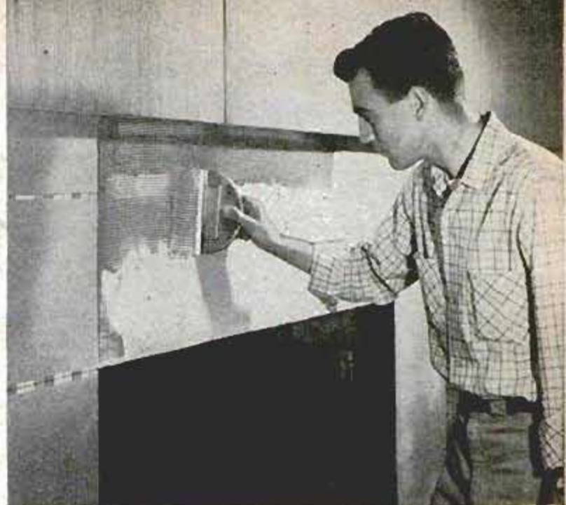
Toothed spreader is used to spread adhesive smoothly and evenly over surfacing material for attaching tile
