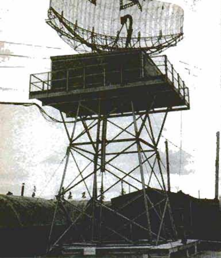
This is a White Alice station main radar-search antenna, without its usual protective dome of plastic
