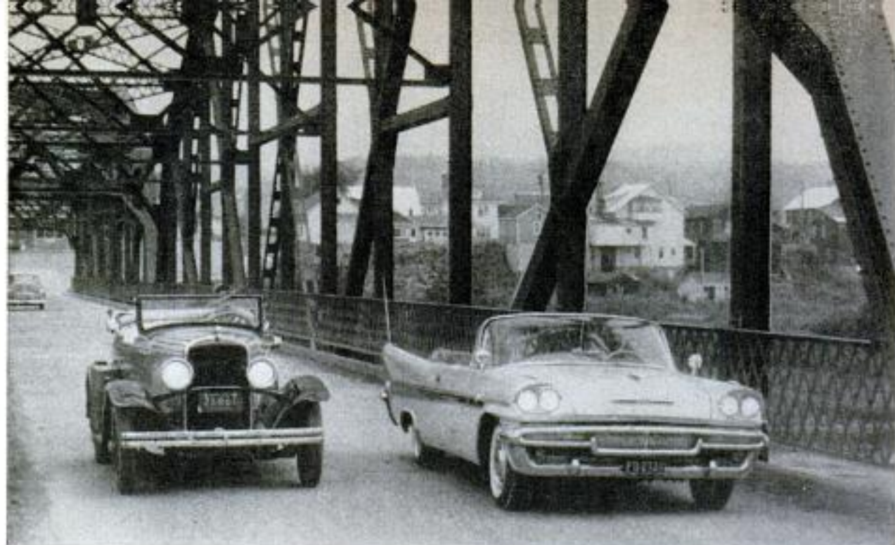
To start the long test, the cars cross the U.S.-Canada border on the bridge at Fort Kent in northern Maine
