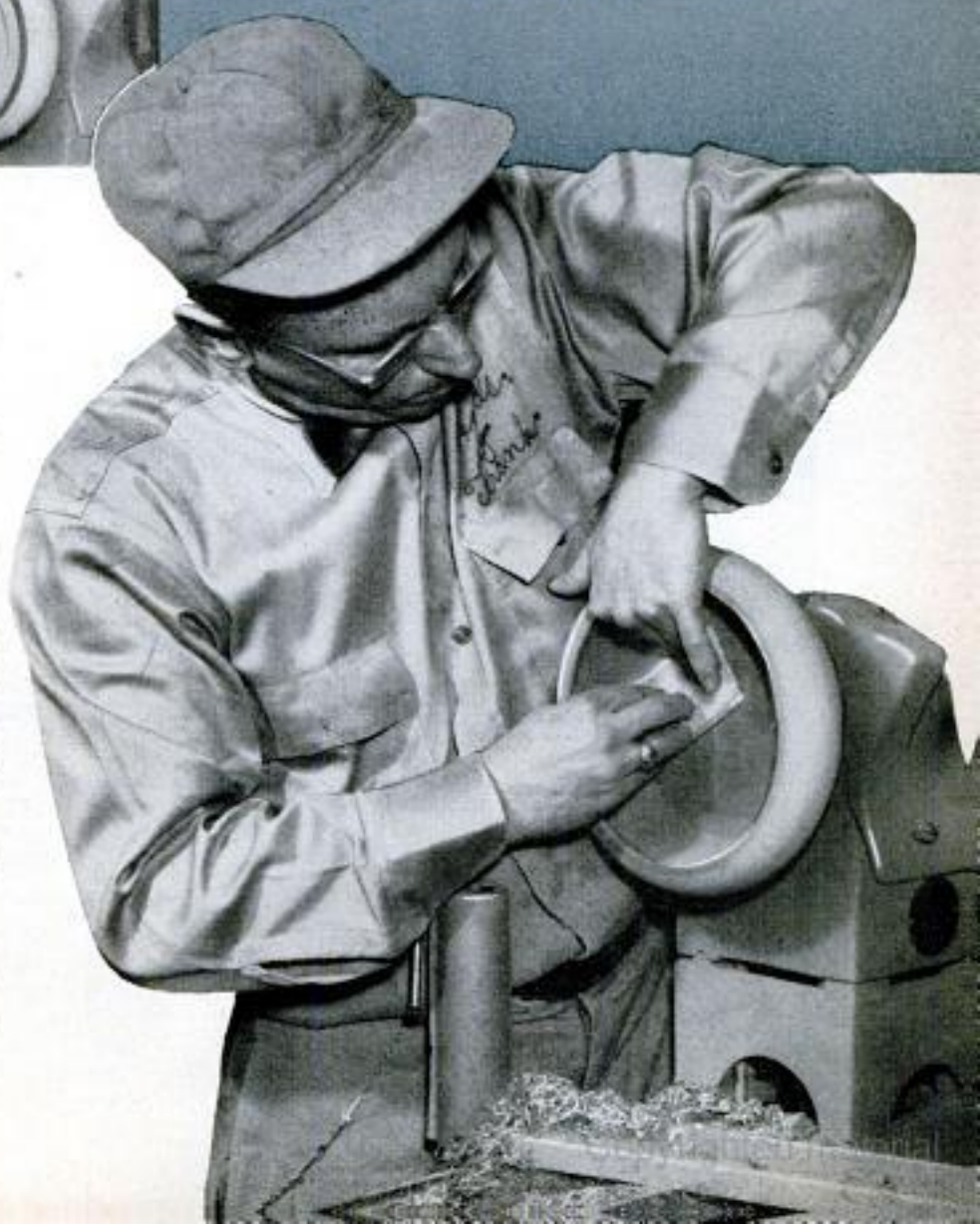
Frank uses five grades of sandpaper to prepare the surface for finishing. The finish includes a coat of sealer, which is followed by three coats of lacquer
