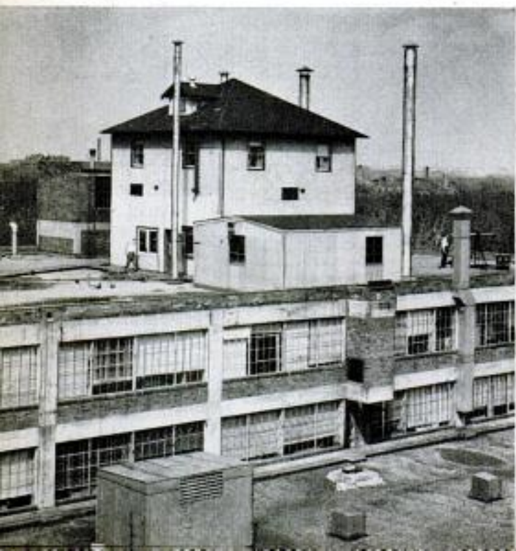
Two-story house atop M-H headquarters building is filled with 200 thermostats for heating research
