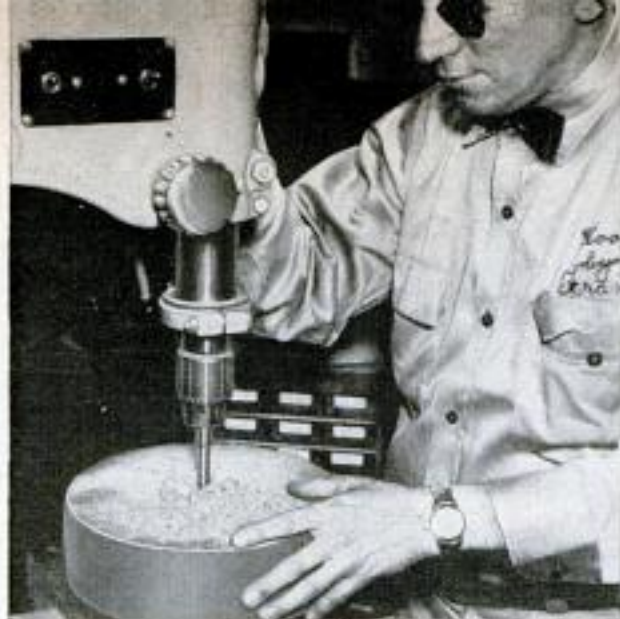
With a drill press he drills a hole which will serve as a maximum-depth guide in his work on the lathe
