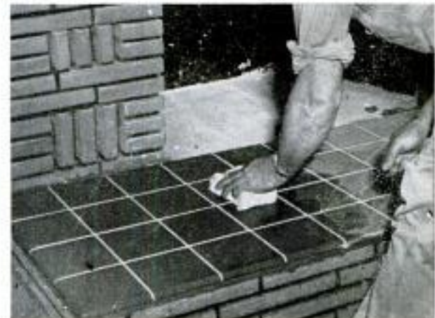
Hearth tile is cleaned with sponge and water. Thin coat of linseed oil is then applied and polished
