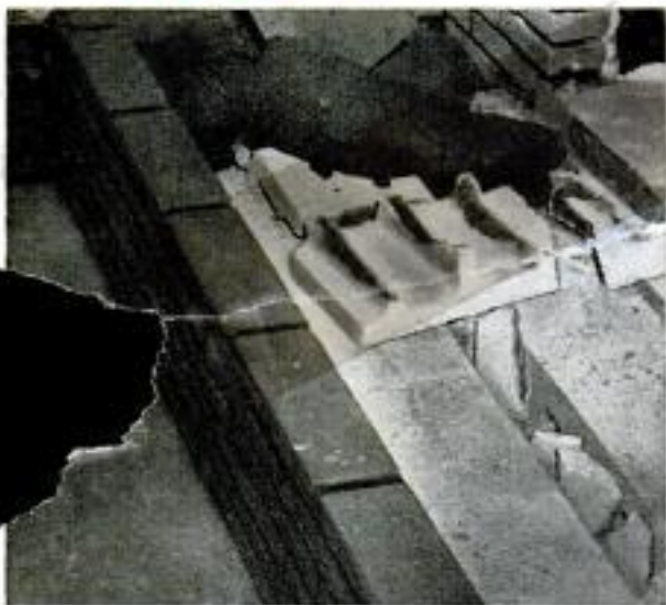
Above, scrap block and brick are used as hearth fill. Below, fill topped with grout, level with firebrick
