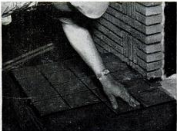
Hearth tile is laid in thin layer of mortar. Note tile is \frac{3}{4} in. above firebrick to form lip for ashes
