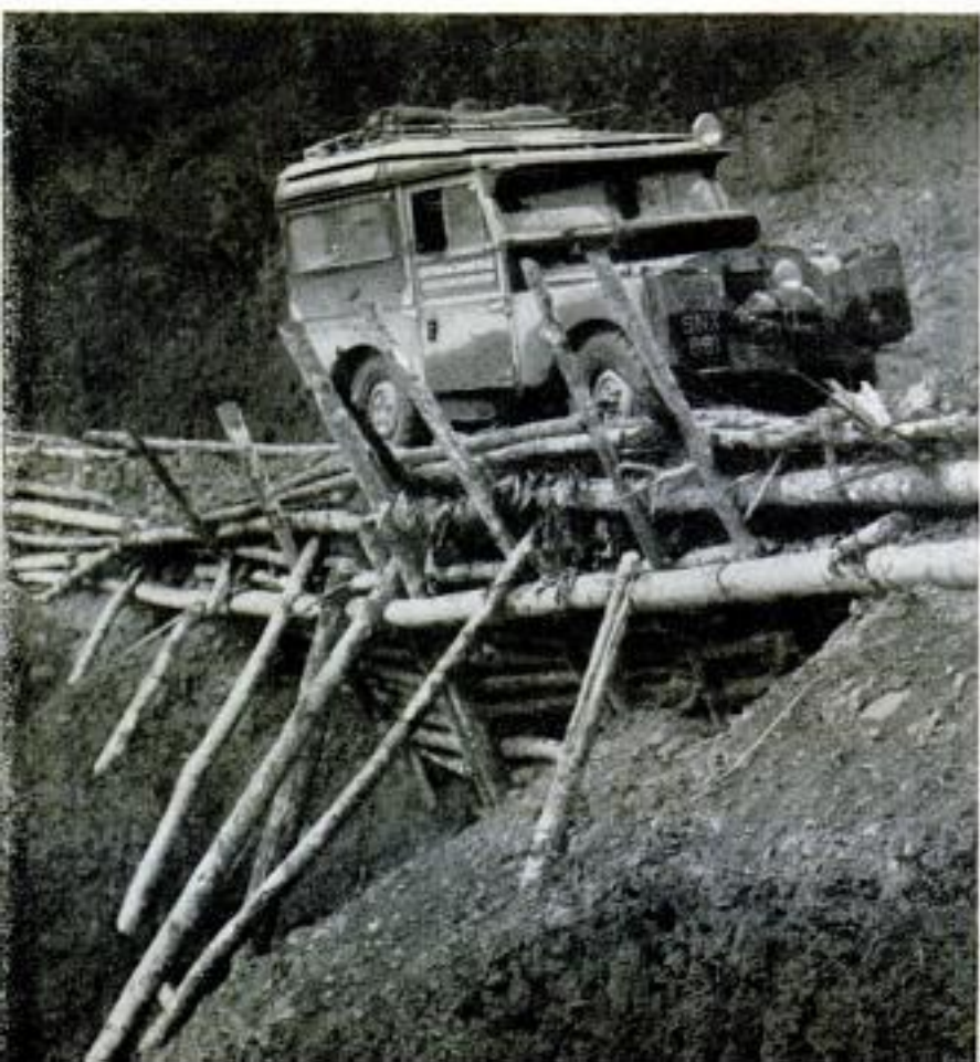
On some of the rivers, Army pontoon ferries were still operating, but they frequently went aground some distance from shore. Below, torrential rains had swept away stretches of the road. Such sections had to be rebuilt with branches
