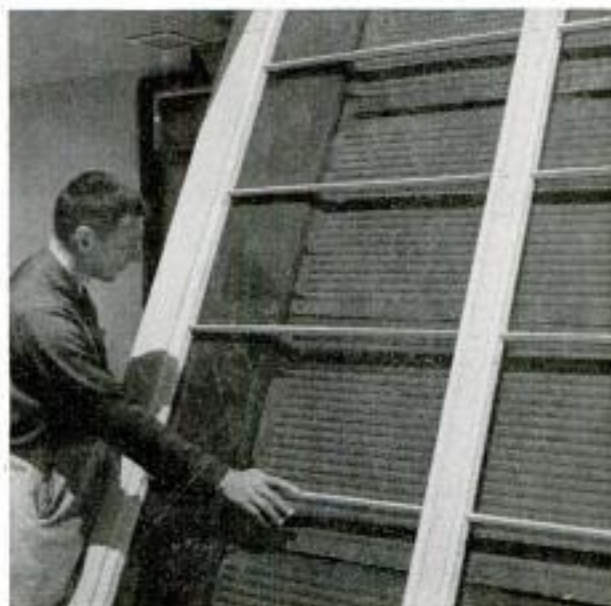
Control panel, above, adjusts heating and cooling circuits. Black heat-collecting plates, below, warm water circulating behind them to 140 degrees
