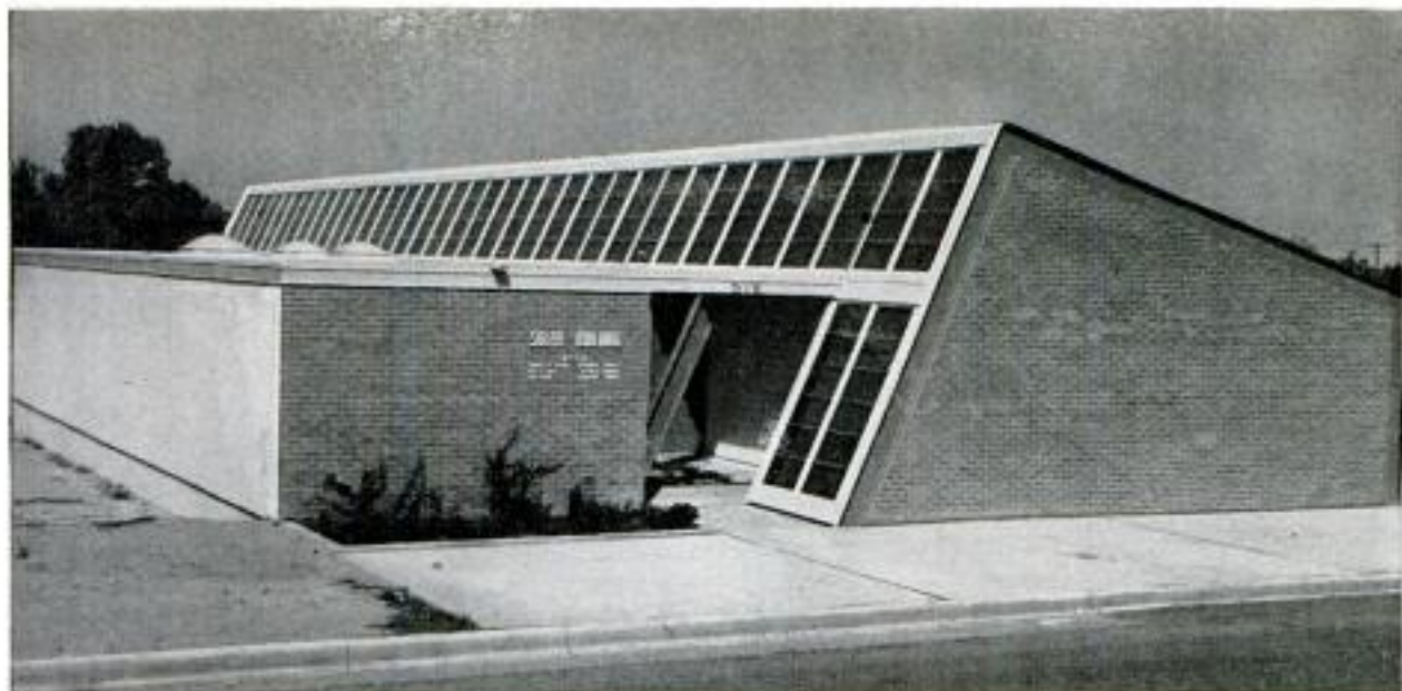
South wall with 830 square feet of solar-energy collecting plates is sloped 30 degrees from vertical
