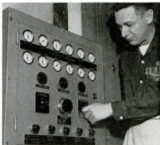
Control panel, above, adjusts heating and cooling circuits. Black heat-collecting plates, below, warm water circulating behind them to 140 degrees
