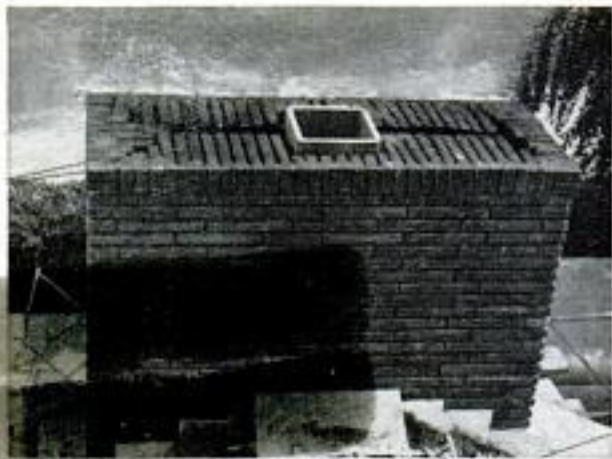
Top of chimney is reached with 18 courses above the ridge. Here fill is completed and ready to be grouted
