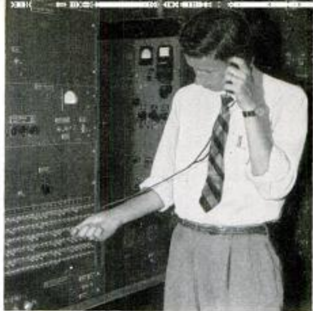
Bank of toggle switches at base of Voice Data Link allows selection of words to be used in messages
