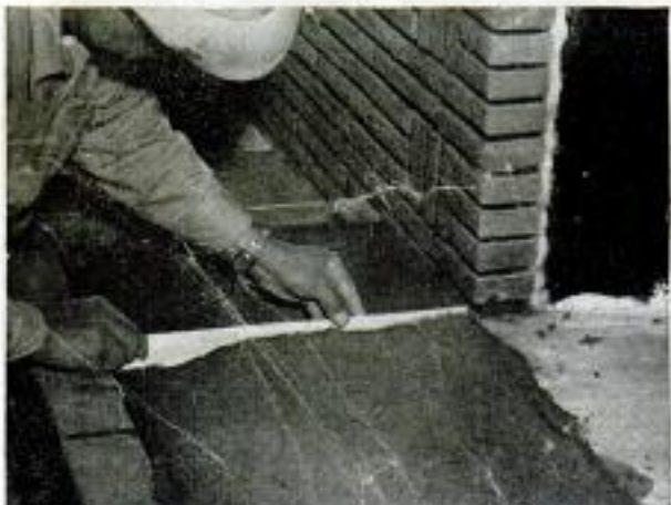
Above, scrap block and brick are used as hearth fill. Below, fill topped with grout, level with firebrick
