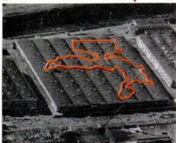
Model is 340 feet long and wide, and its 29,000 square feet represent 550 square miles of bay area. Its tremendous size is outlined at left on warehouse which houses it
