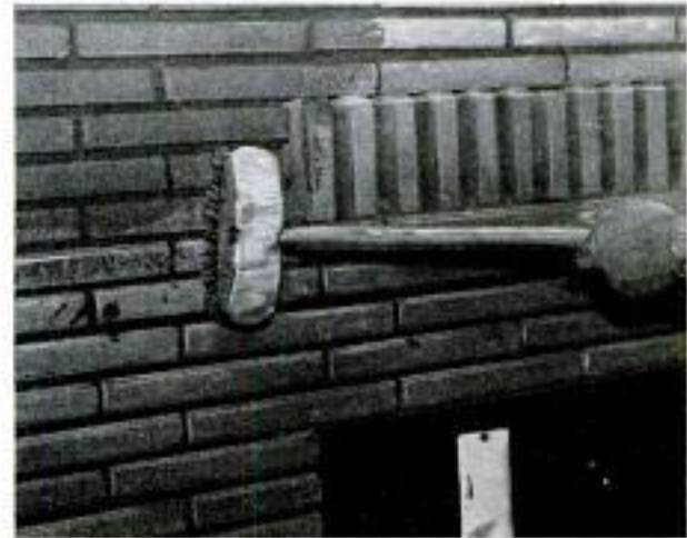
A 10-percent solution of muriatic acid is used to clean brick of mortar stains, then rinsed with water
