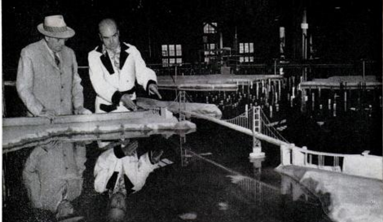
Golden Gate Bridge section of model shows care taken to reproduce San Francisco Bay exactly in miniature
