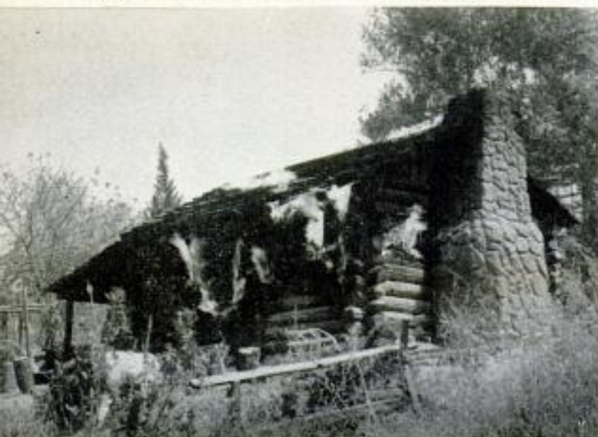
Frontier cabin is left in flames after attack by savages. But flames really come from gas jets and building is concrete
