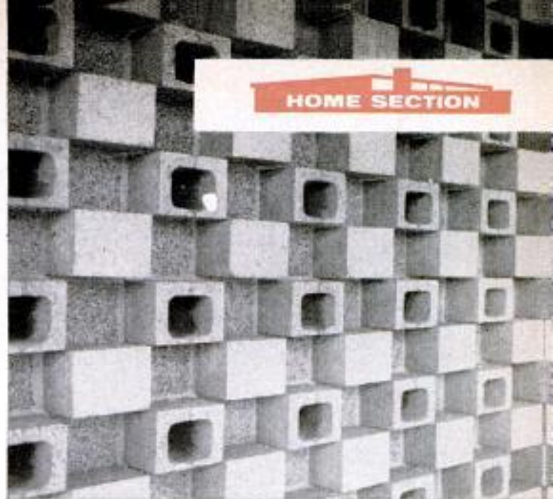
Single-core blocks project from standard-block wall
