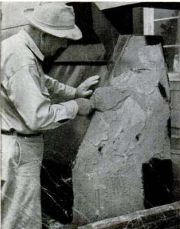
Layer of glass-fiber insulation, which is added to steel liner, is held in place with coating of mortar
