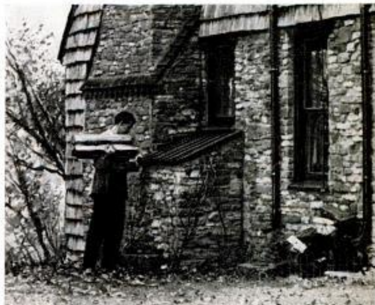
Les takes his turn at splitting shakes as the pile grows. Below, solid-stone wood box on outside of living-room wall can be filled from the outside. Stonework is tied into the wall and corner of chimney
