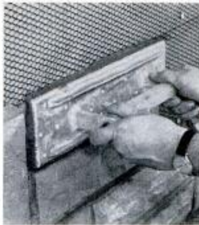
"Stone" mold is pressed lightly to embed it in metal-lath surface
