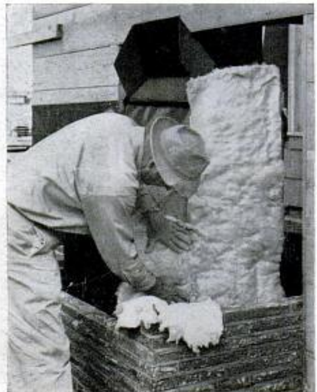
Besides acting as insulation, glass fiber also serves as spacer to keep common brick from touching liner
