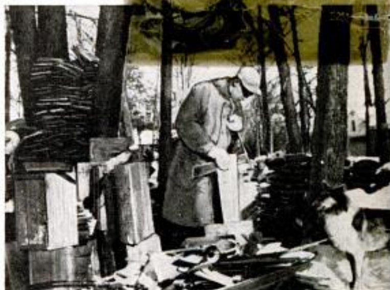
Les takes his turn at splitting shakes as the pile grows. Below, solid-stone wood box on outside of living-room wall can be filled from the outside. Stonework is tied into the wall and corner of chimney
