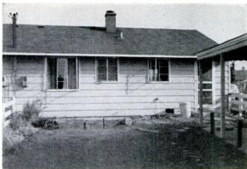
Rear view of home before split-level addition was started. Earthmoving machines couldn't operate in small space so excavation was by hand
