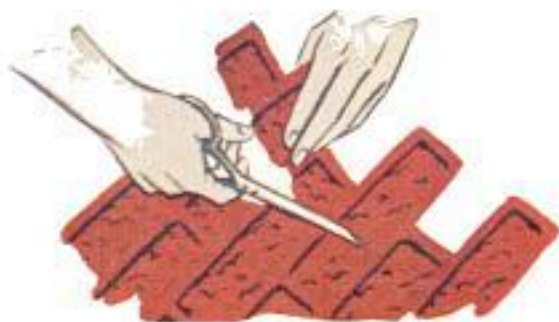
Brick is easily cut with scissors, knife or razor blade for fitting at sills, casings and wall ends
