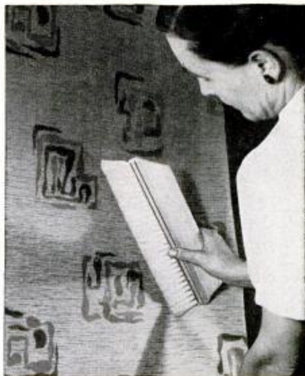
Brush out strip to smooth it, working from center outward to remove wrinkles. Damp cloth can be used
