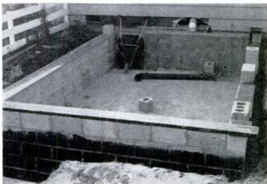
Concrete-block walls are started, above, on concrete-slab floor. The white lines on the photograph below indicate the framing for the upper level and location of a new window for one of the original bedrooms
