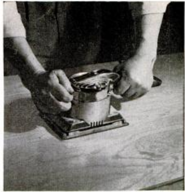
After plywood has been attached to both sides and mastic has set, wood is sanded with fine-grit paper
