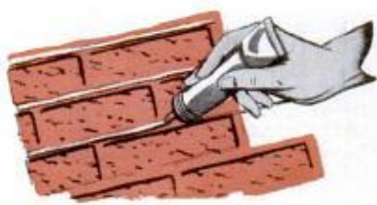
Bead of adhesive is applied to the mortar lines on back of panel. Both vertical and horizontal are coated
