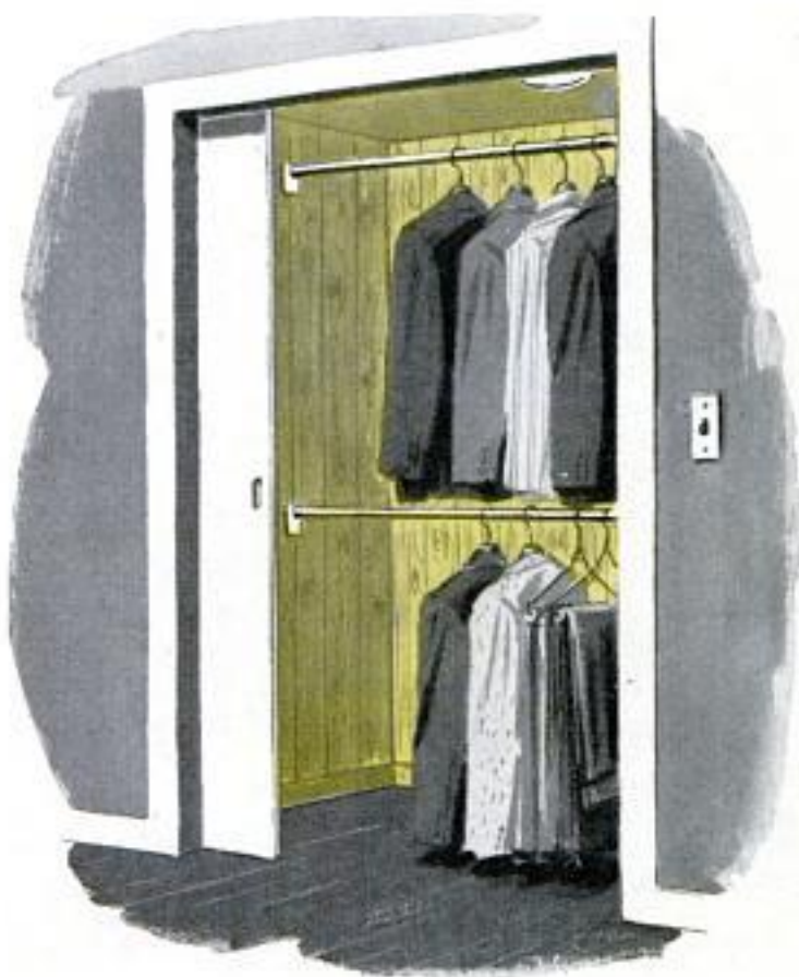
In closet below, original clothes pole has been moved up, a second pole installed lower down, so closet capacity is doubled
