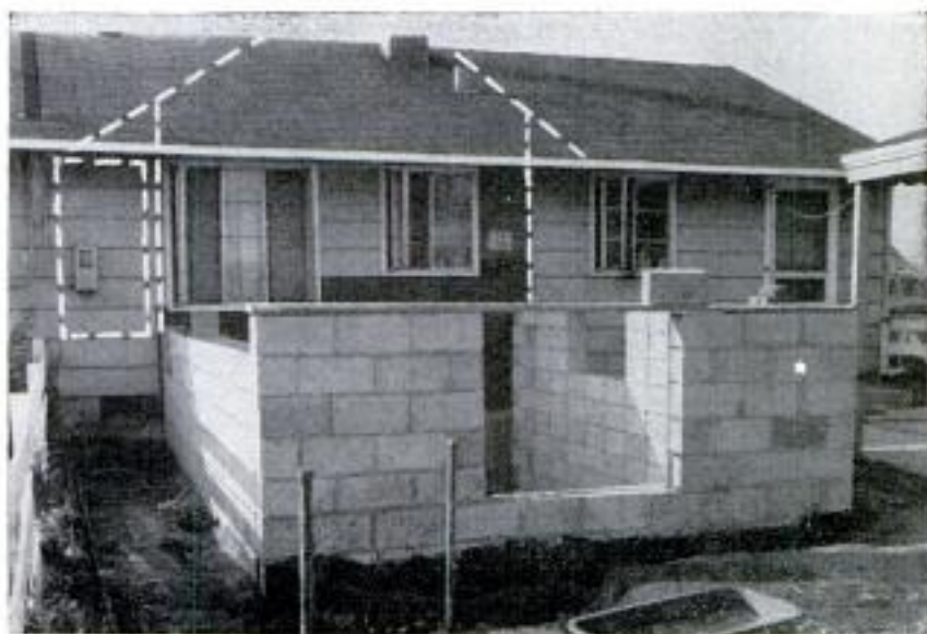
Concrete-block walls are started, above, on concrete-slab floor. The white lines on the photograph below indicate the framing for the upper level and location of a new window for one of the original bedrooms
