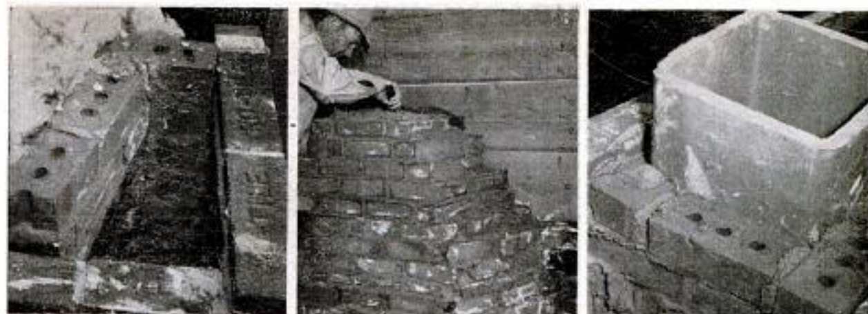
Left, steel liner is encased with common brick. Cross-row of brick in background forms back of cold-air duct. Center and right, brick is corbeled 30 deg. to form 12 x 12-in. flue opening. Inside is buttered with mortar
