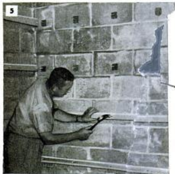
Above, fastener is similar to that pictured in Fig. 1. Suitable for light to medium loads. Below, special fastener is attached to wall with adhesive.
