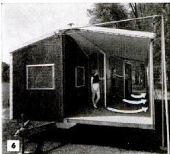
6 Now, above, the end walls and two interior walls swing into position, as indicated by the arrows
