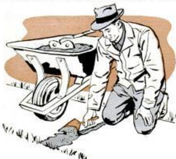
Crack in walk then is filled with concrete, which is tamped thoroughly to compact it into all spaces
