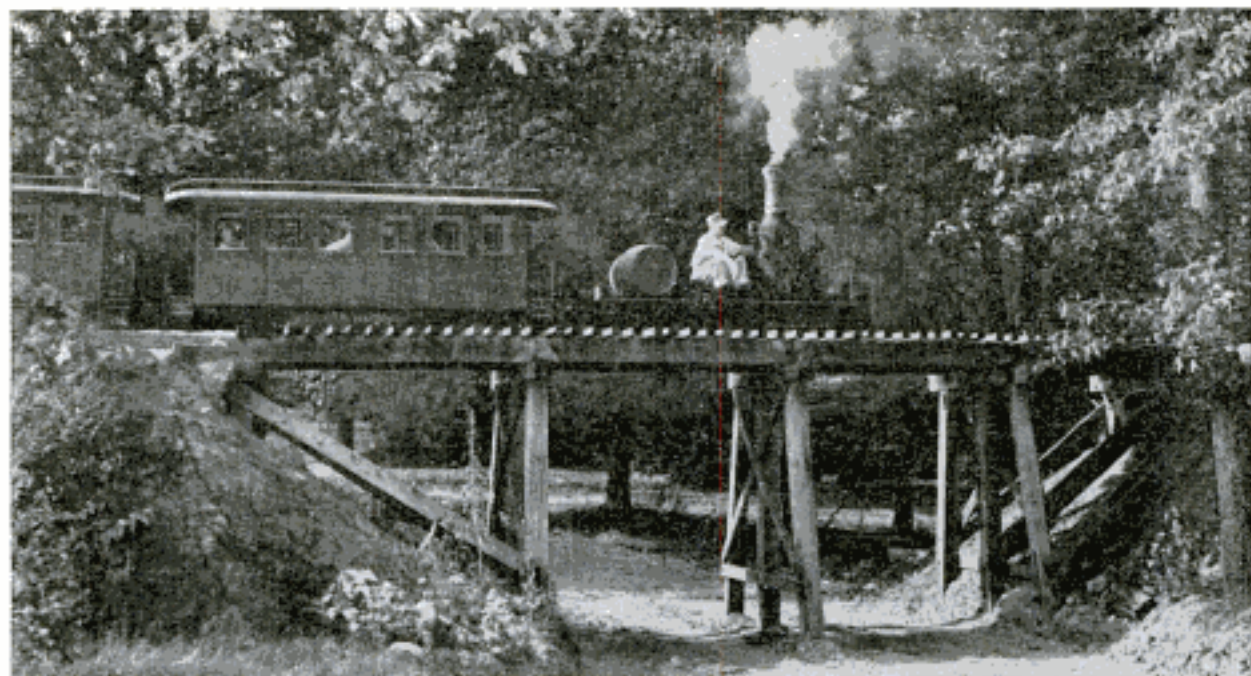
Eastbound train, right on time, steams across the main trestle, which is 40 feet long, 16 feet high
