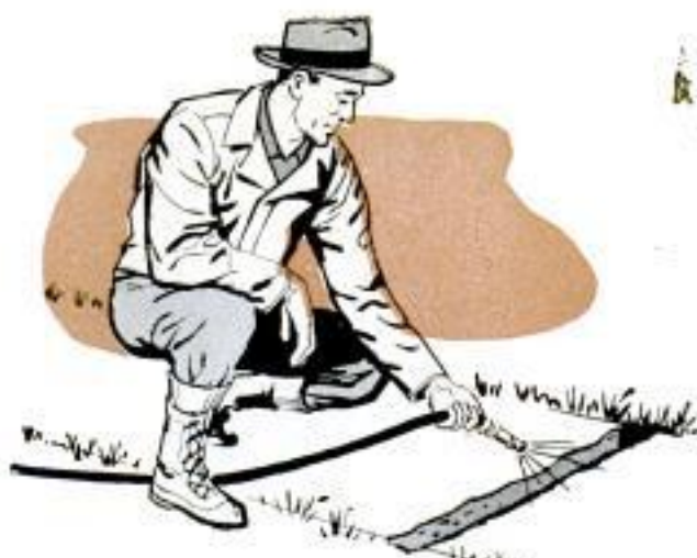
Old concrete then must be thoroughly wet down to prevent it absorbing water in fresh concrete mix
