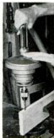
Air from vacuum cleaner operates \frac{1}{8} -inch drill on standard drill chuck (above), sands boat bow (below) Electrolux Corp., 500 Fifth Ave., New York City
