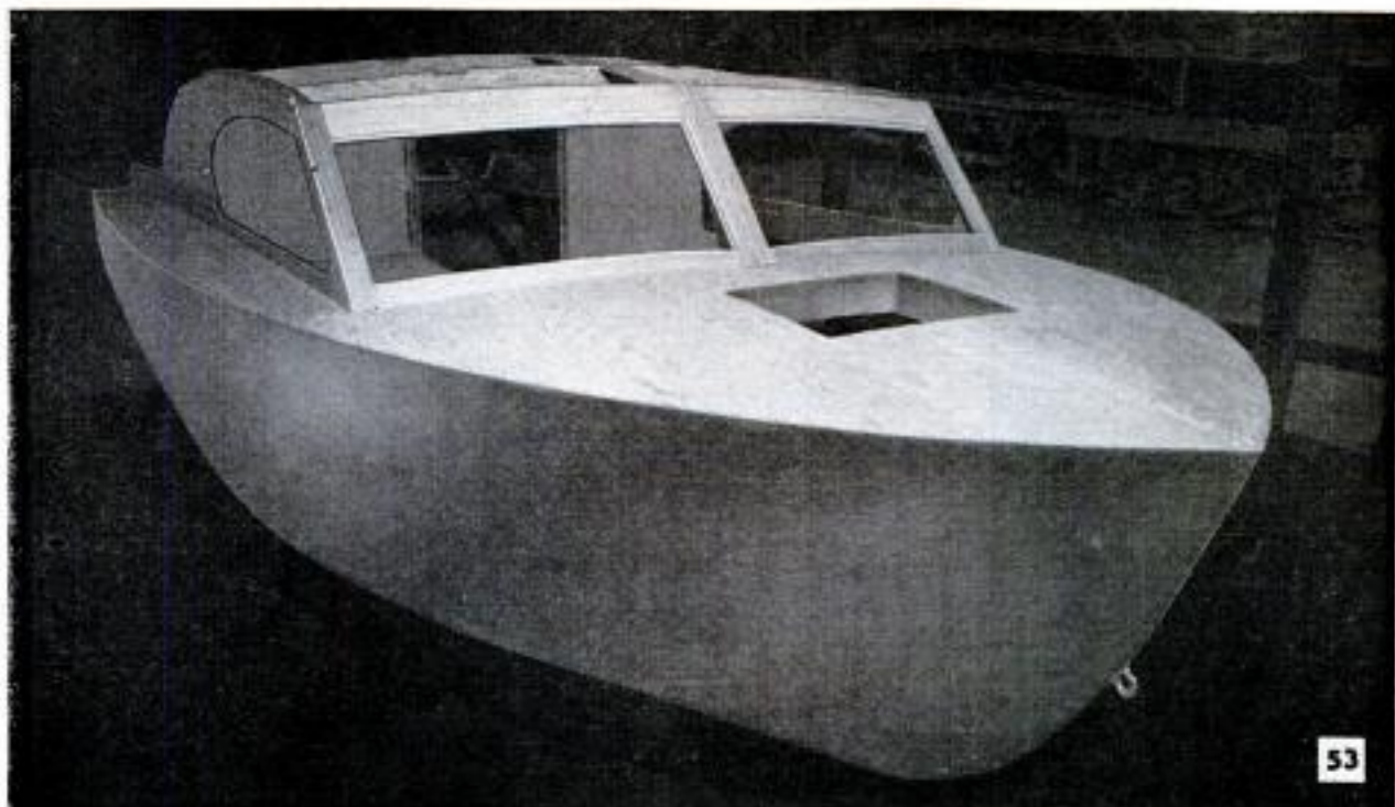
Cabin sides and windshield have been added and beams installed to support plywood roof which is added next
