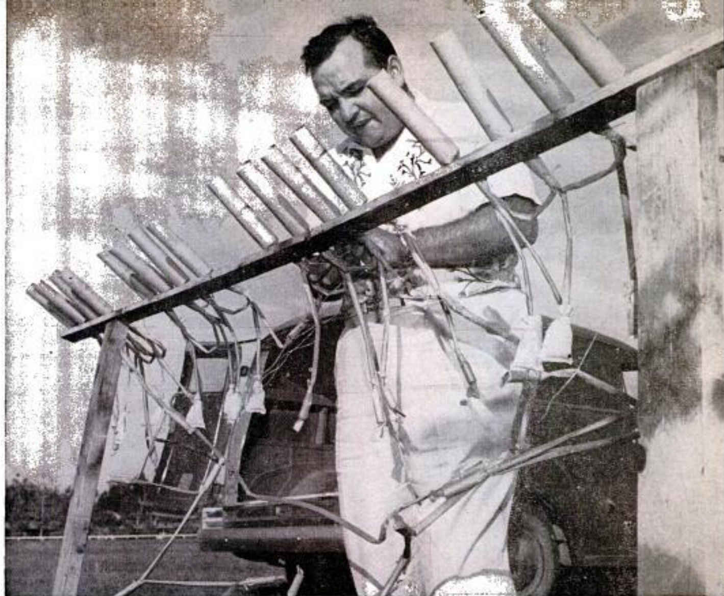
Lizza checks wiring which will detonate this barrage of "candles." They are triggered from firing station
