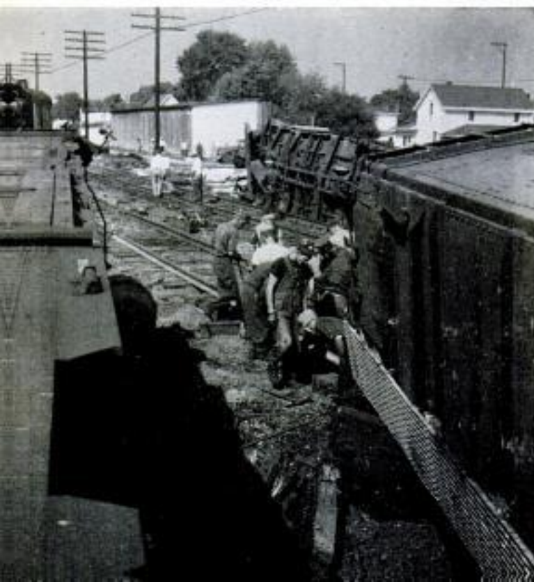
Track-repair crew replaces the bent and broken rails as fast as the crane moves wreckage out of the way
