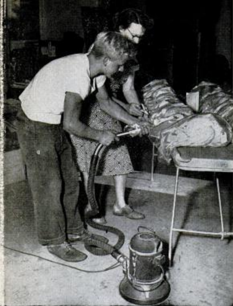
Vacuum cleaner, above, pulls packaging bags tight against turkeys. Fans, below, keep eggs fresh by forcing air chilled to 50 degrees through baskets
