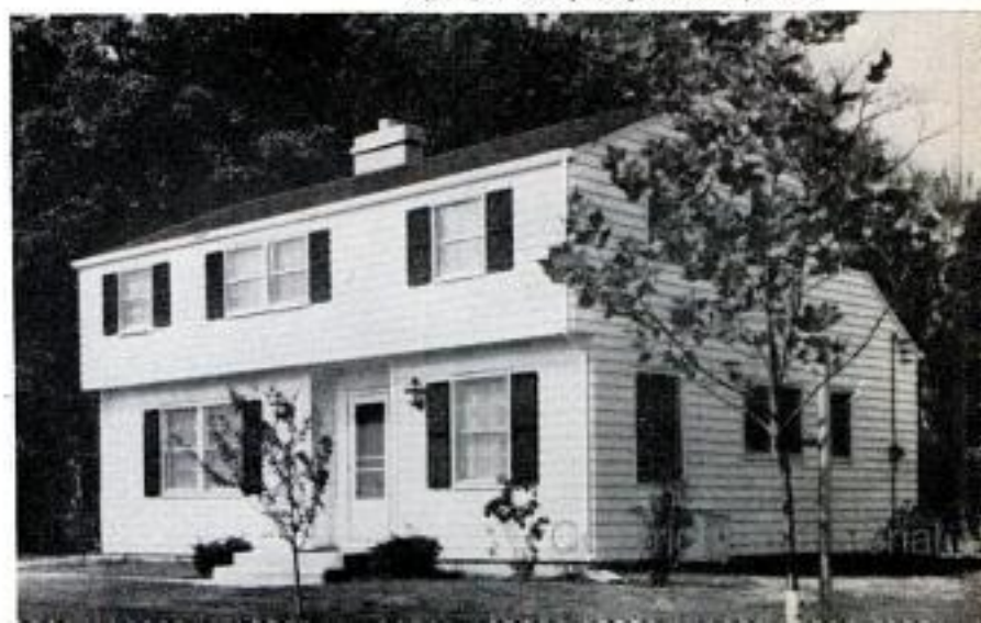
Midwest Houses, Inc., Mansfield, Ohio.
