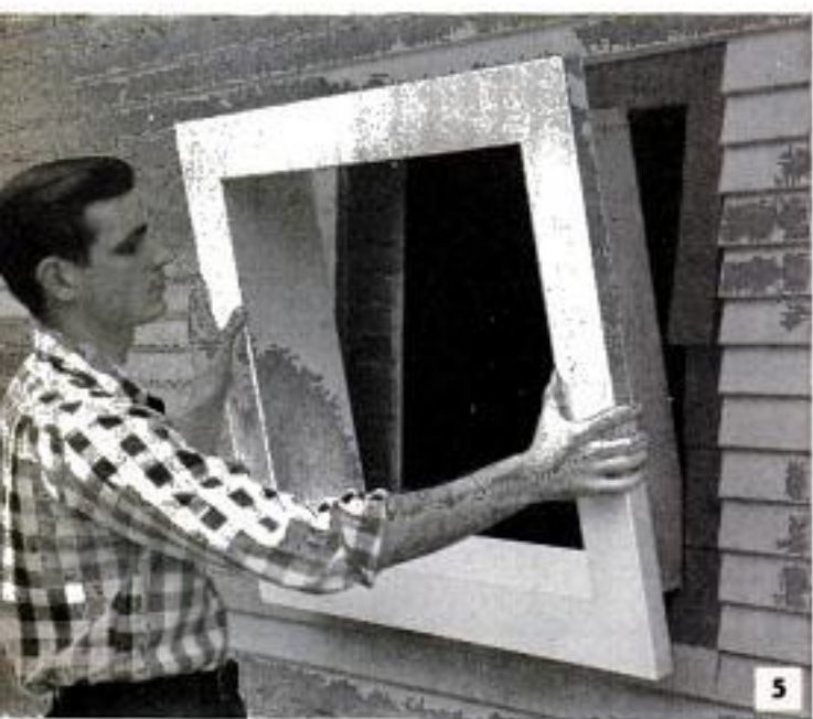
Above, this part you make yourself. It is called a surround and is nailed securely in the opening
