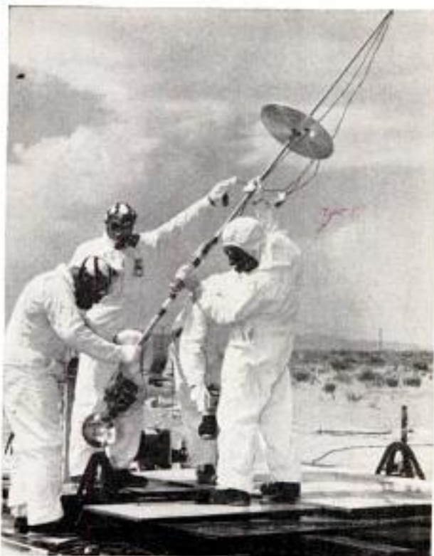
Camera on a "fish pole" is lowered into a "hot" tank at Hanford. Strange rig had to be devised because the tank was intensely radioactive and there was only a small opening at the top. Below, a new electrostatic generator strikingly resembles a guided missile
