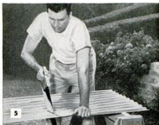
Above, cross pieces are staggered to break dominant lines of corrugated roof. Fig. 4, pre-painted 2 x 4 nailed directly to house supports upper end of roof. Fig. 5, glass fiber is easy to cut with fine-tooth saw
