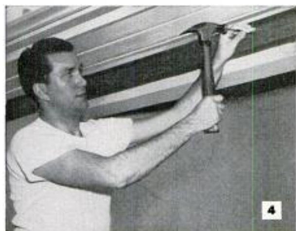
Above, cross pieces are staggered to break dominant lines of corrugated roof. Fig. 4, pre-painted 2 x 4 nailed directly to house supports upper end of roof. Fig. 5, glass fiber is easy to cut with fine-tooth saw
