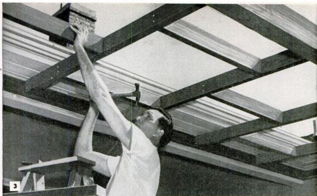
Above, cross pieces are staggered to break dominant lines of corrugated roof. Fig. 4, pre-painted 2 x 4 nailed directly to house supports upper end of roof. Fig. 5, glass fiber is easy to cut with fine-tooth saw
