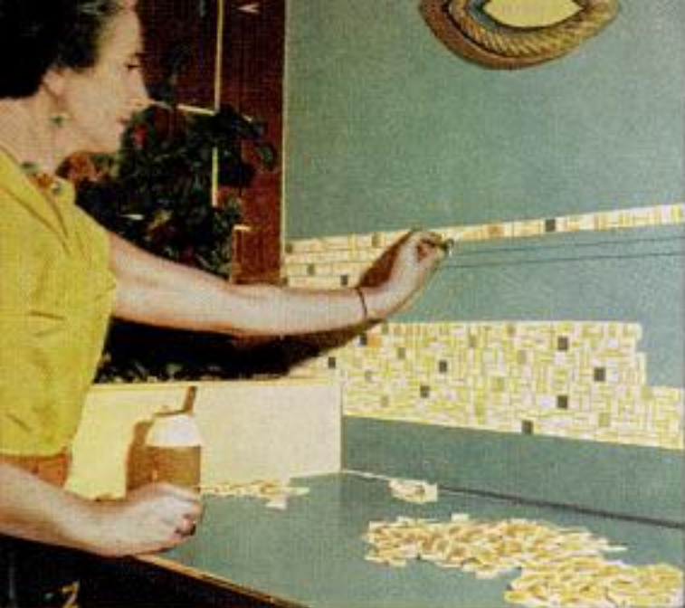
The beginning of an attractive, easy-to-clean splashboard above the work counter in a kitchen
