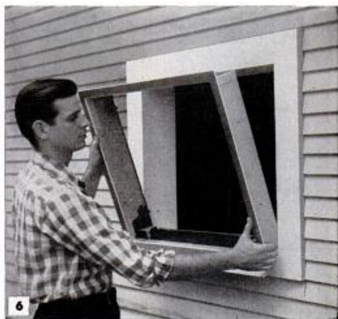
Above, metal sleeve assembly is installed next and is screwed solidly to the surround at top and sides
