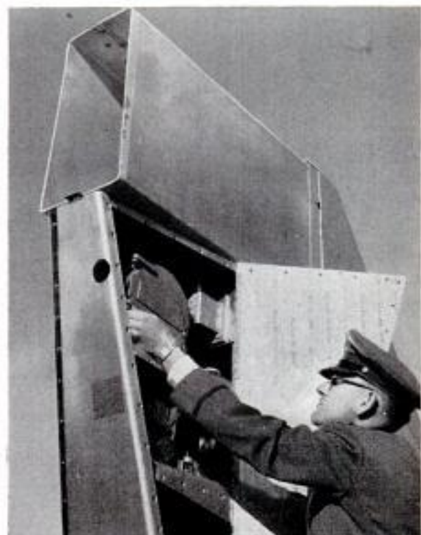
Photo officer adjusts the camera which shoots through a hole in the tail of the drag parachute sled
