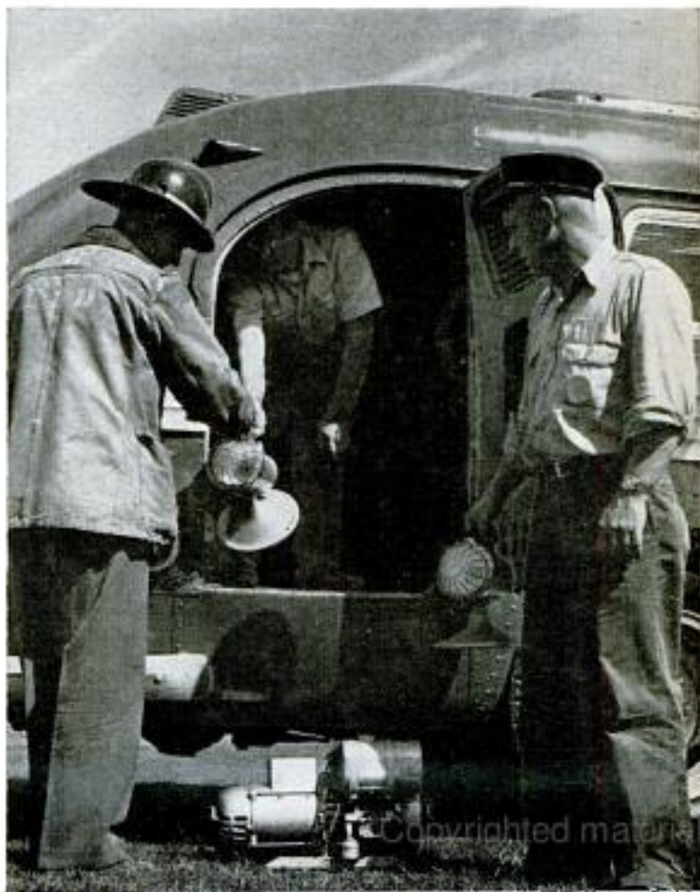
Once a luggage compartment, now storage space for two portable electric generators, wires and lights
