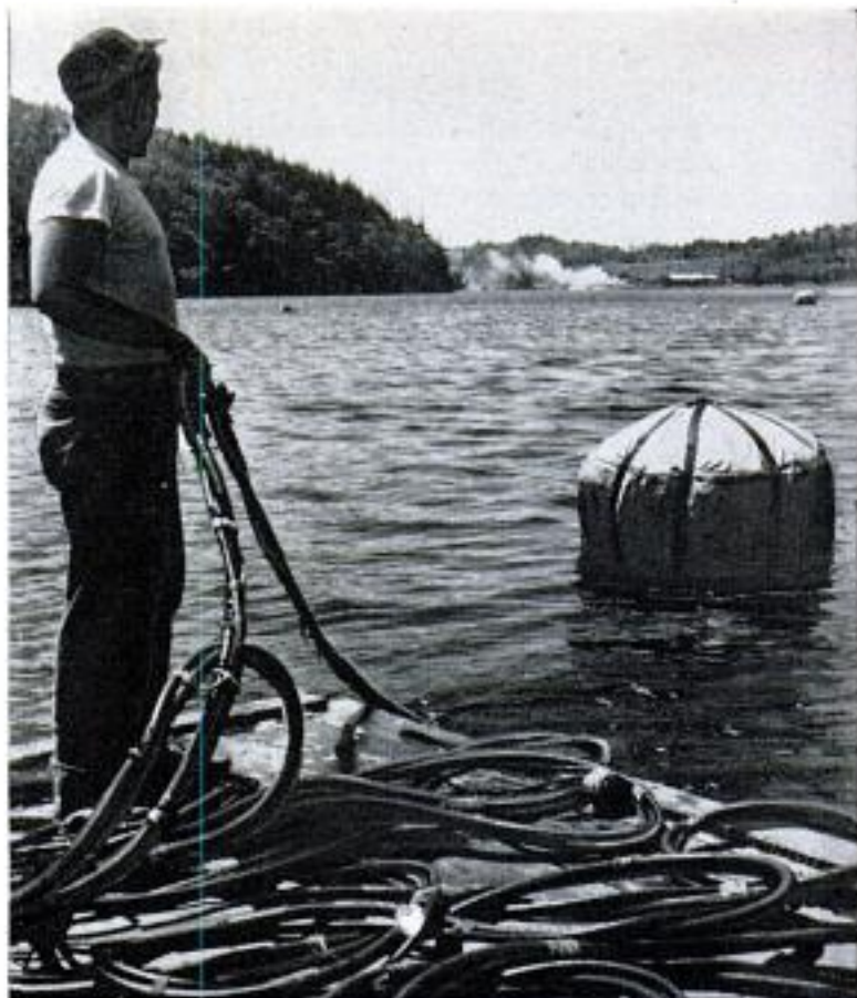
Canvas-bag buoys, when inflated with air, bring logs to surface
