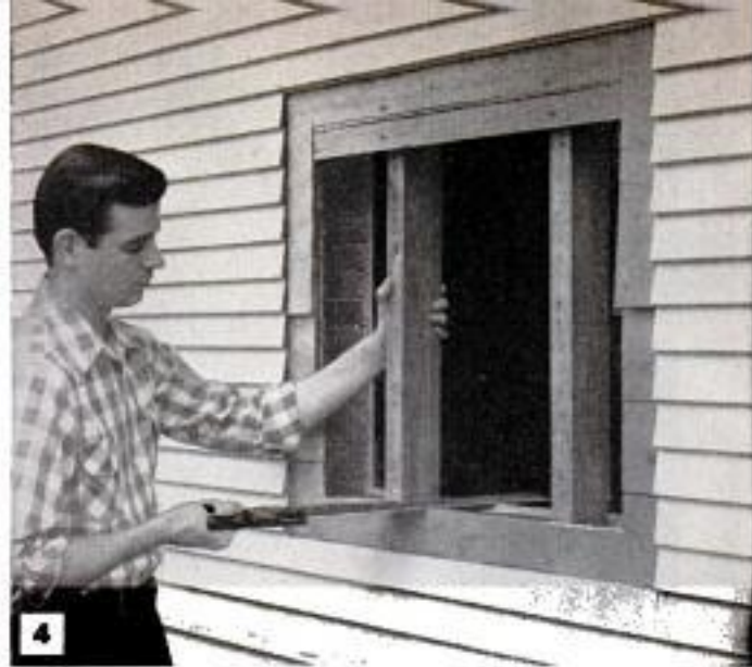
When siding and sheathing have been ripped off rough-cut opening, a handsaw is used to saw off the studs flush. Notice how siding has been cut back
