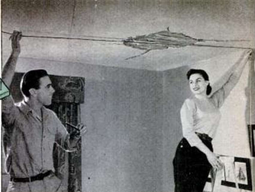
Photos and information courtesy The Uppson Co. Above, for equal borders and correct location of furring strips, first establish center line at right angles to joists
