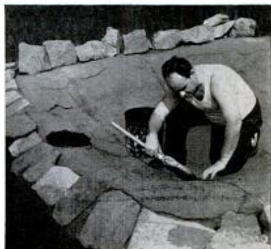
Above, flagstones weight the edge of the paper liner and help decorate pool. Below, short-handle broom will be found handy for applying the roofing cement to the lapped roofing seams
