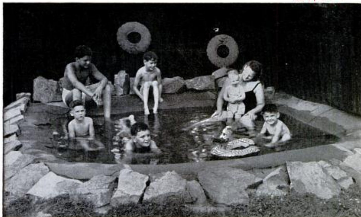
Completed pool being enjoyed by whole family. Top layer of liner can be colored, slate-surfaced roll roofing
