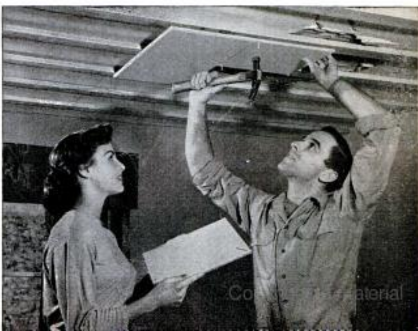
Above, furring strips are nailed to ceiling joists for safe support of tile. Below, after correct positioning of all strips, tiles are applied starting at center of ceiling
