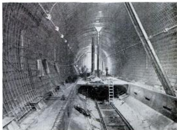
Above, build-up of the two islands at ends of the tunnel required 5\frac{1}{2} -million cubic yards of "fill." Below, double-shell steel tunnel casing is wide enough for 23-foot, two-lane road
