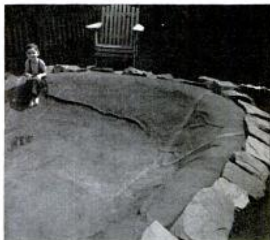
Above, flagstones weight the edge of the paper liner and help decorate pool. Below, short-handle broom will be found handy for applying the roofing cement to the lapped roofing seams
