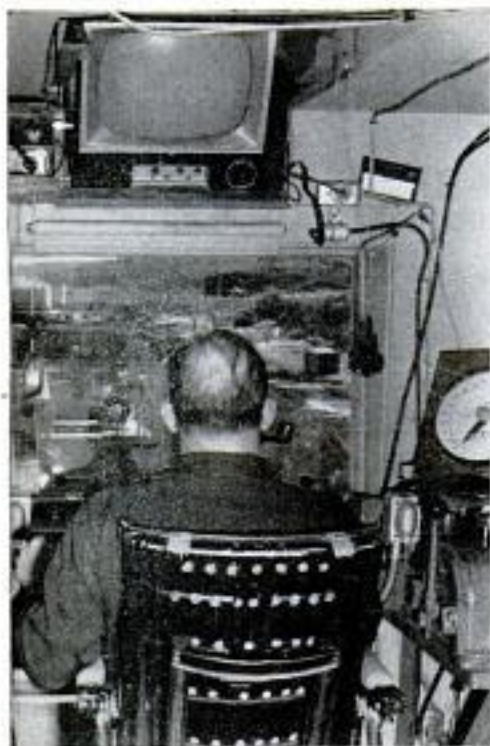
Above, cabledway operator watches loading from control house. Right bottom, cables pick up concrete buckets from railroad cars. Right top, bucket is guided to the dam for dumping and return to siding
