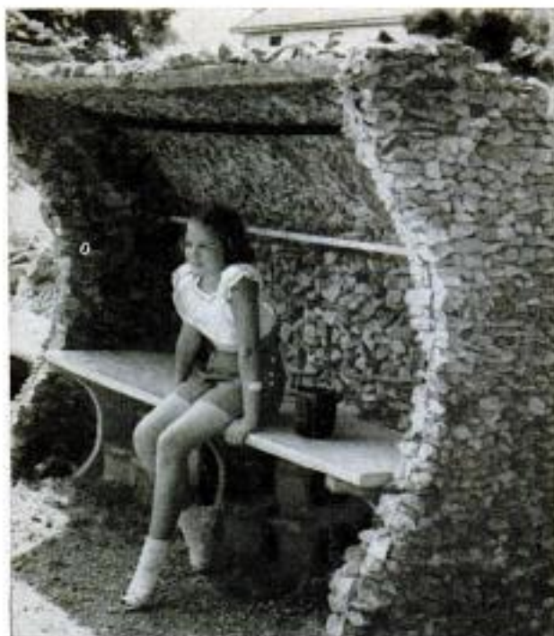
Rock settee has a chicken-wire skeleton. Below, the 10-foot Cupid's heart with arrow has served as altar for many weddings. Bottom, sample of stone fences
