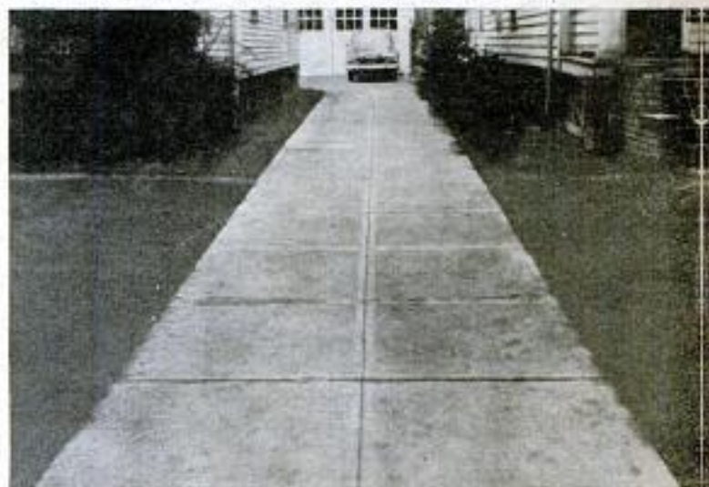
This wire-reinforced driveway has withstood wear and erosion for many years and is still intact, no cracks or frost damage visible throughout the length
