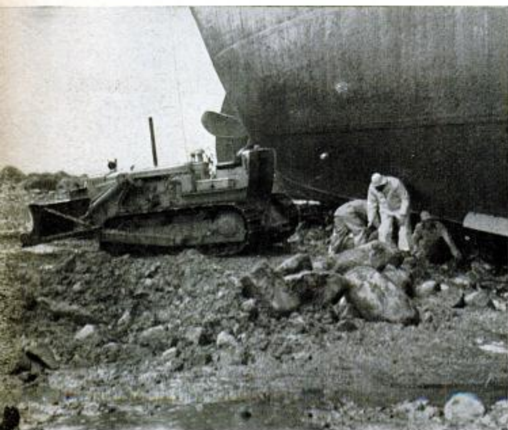
Salvage workers had to crawl under the ship to clear away boulders. Logs and sheets of steel were placed in the bulldozed channel to ease the movement of the ship. Much of the salvage work had to be done in rain
