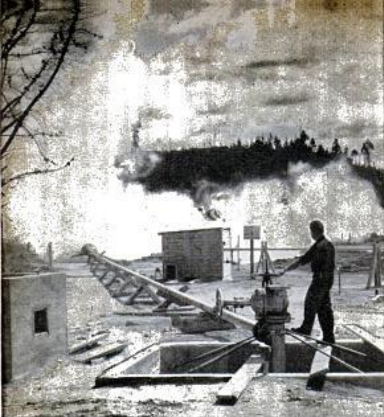
Steam from a "cleaned" well is deflected into horizontal pipes and shoots 100 yards across countryside
